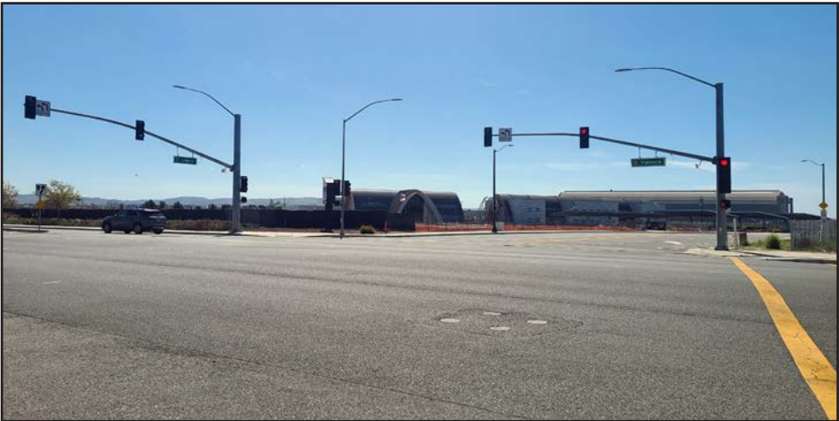
View 8: From the northern corner of the Valencia Avenue and Kensington Park Drive intersection, looking south at a construction site at the southern corner of the intersection. Legacy Magnet Academy campus, and the Tustin Hangar #2 in the background.
