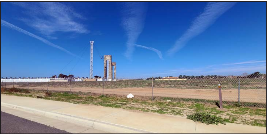
View 2: From the north side of Legacy Road, looking northwest at the project site and the former MCAS Tustin facilities in the background.
