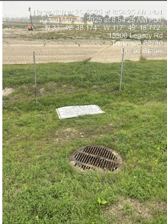
Photo 16: Stormwater inlet adjacent to western edge of parcel, shown here.
