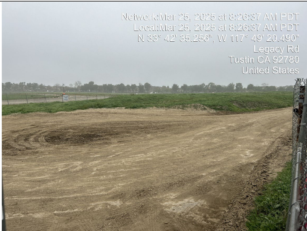
Photo 12: Site overview. View of the southern corner of the site facing west from the southern corner of the parcel.
