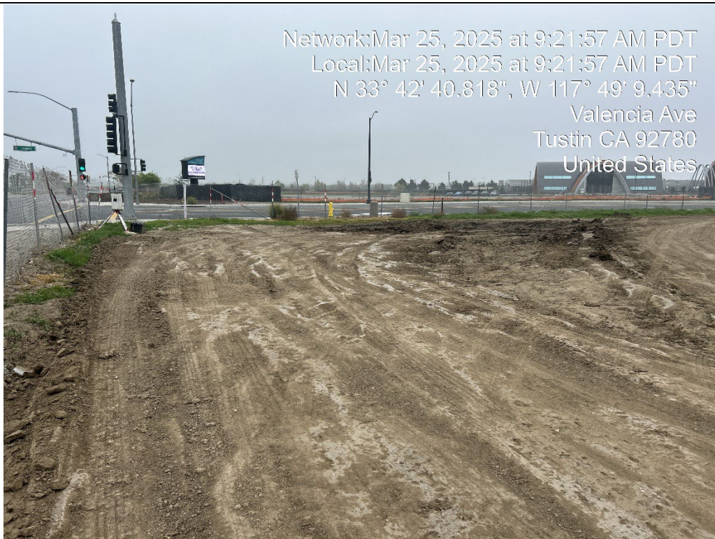
Photo 10: Site overview. View of the northern corner of the parcel looking east.
