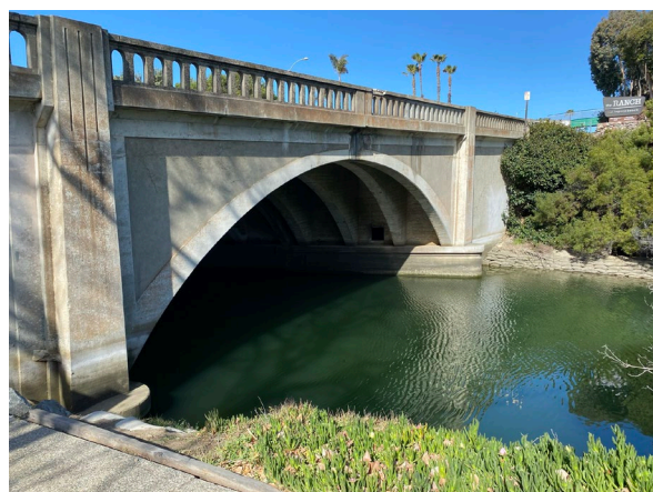
Photograph 10. The Coast Highway Bridge over Aliso Creek, originally constructed in 1926, is a historic architectural resource.
