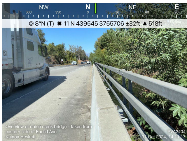
Photo 6: Overview of Euclid Avenue segment from Chino Creek Bridge
