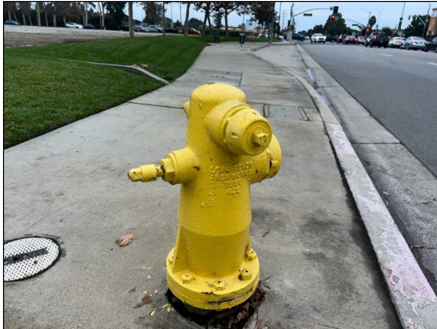
Figure 5. 1990-Dated Fire Hydrant on Clark Avenue (view South; October 14, 2024).
