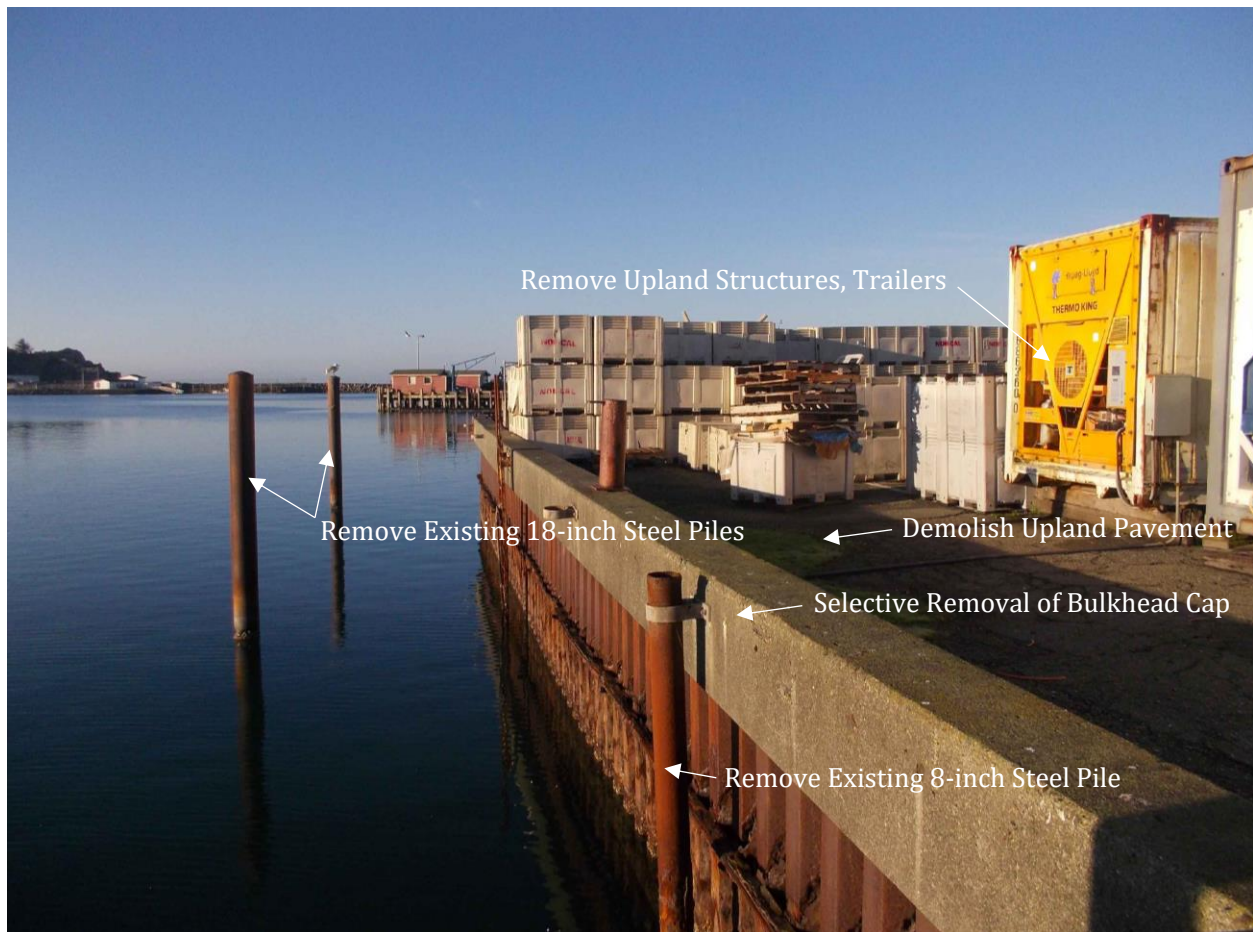
Figure 7. To be Removed Steel Piles, Bulkhead Cap, and Upland Pavement
