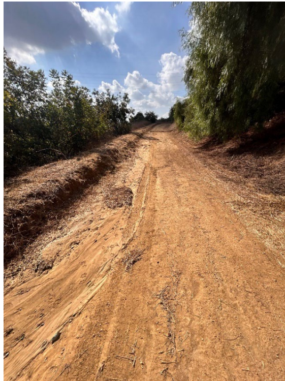
Photo 4: Downhill drainage movement through section of Bonnie Cove West Trail.
