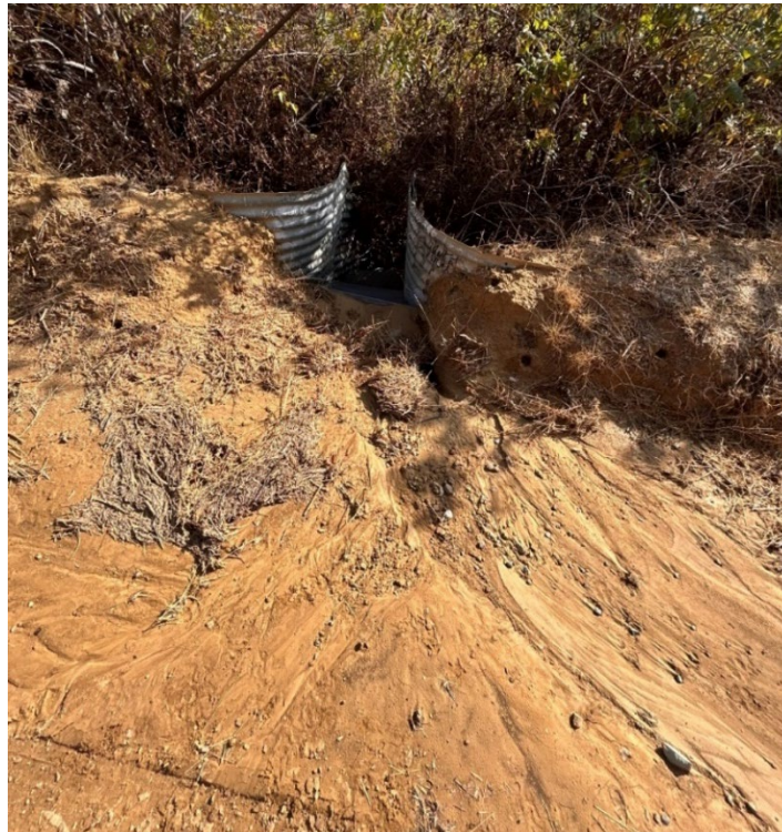
Photo 6: Culvert outlet on Bonnie Cove West Trail, facing east.
