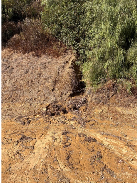
Photo 5: Water runoff outlet on Bonnie Cove West Trail, facing west.
