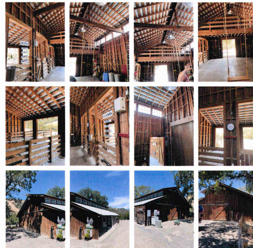
7 Existing Barn - Exterior and Interior Photos
