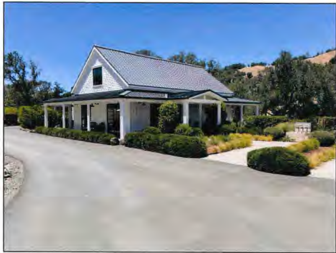
VIEW OF SOUTH FACADE LOOKING EAST FROM ENTRY DRIVE
