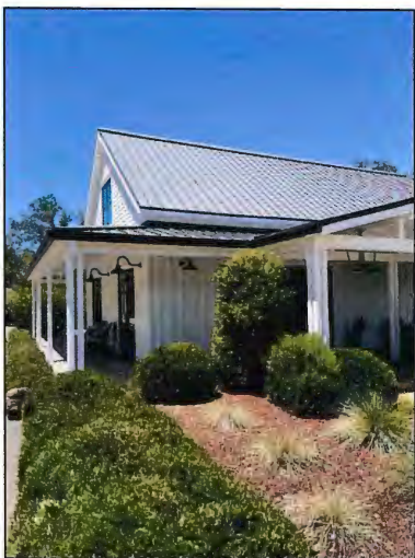
VIEW OF SOUTH FACADE LOOKING EAST
