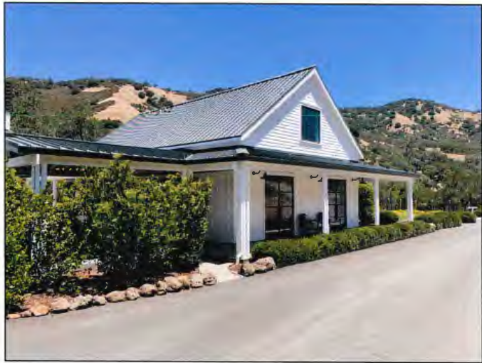
VIEW OF SOUTH FACADE LOOKING WEST FROM ENTRY DRIVE
