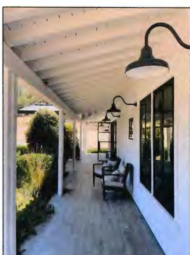
COVERED PORCH LOOKING SOUTH
