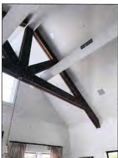
GREAT ROOM EXPOSED TRUSSES & CEILING TREATMENT
