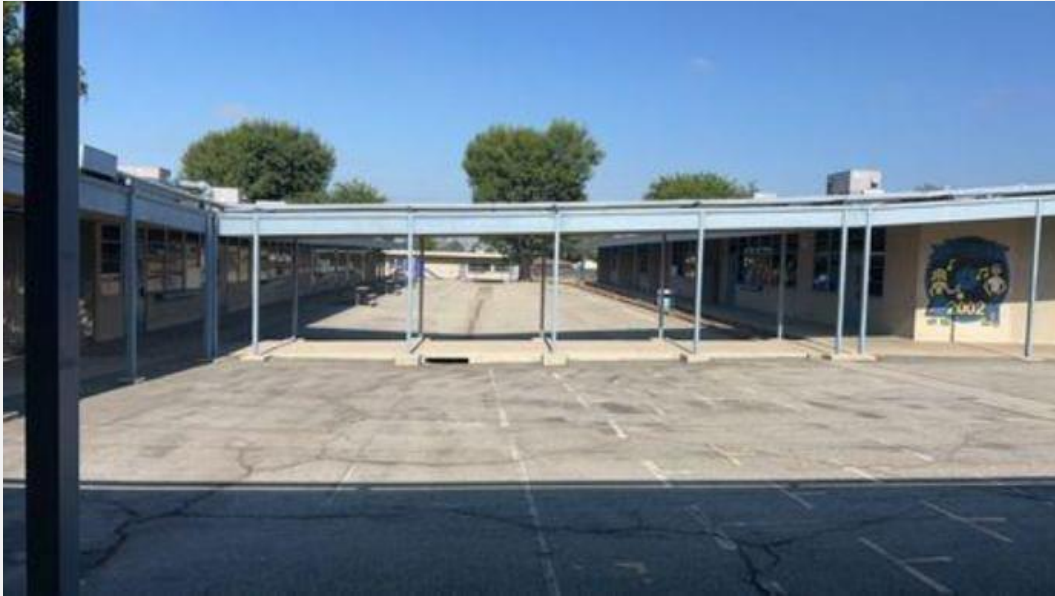
Exhibit 1. Overview of the central section of W.R. Powell Elementary School, view facing west.
