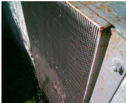
Trash rack with screen
