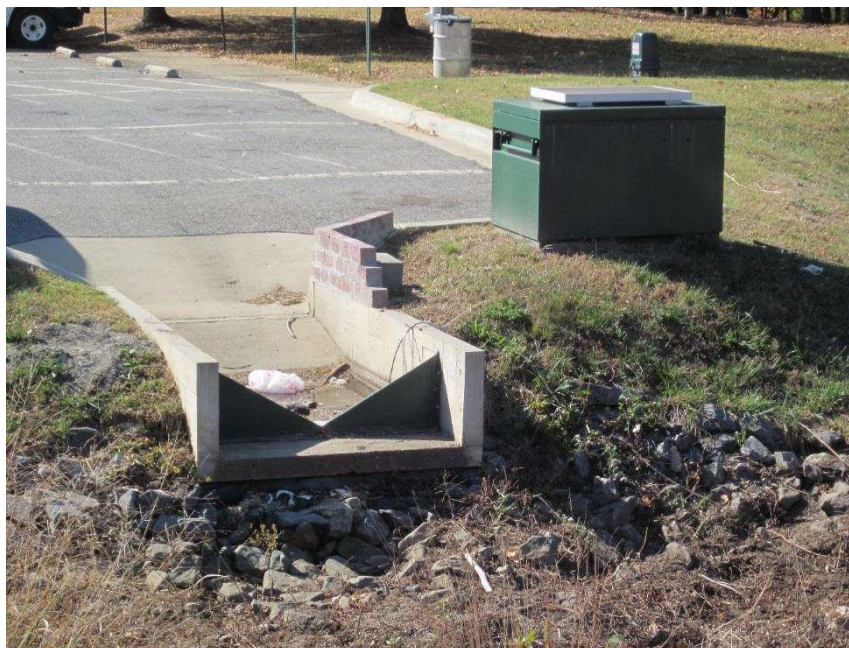
Figure 4. Example inlet structure.
