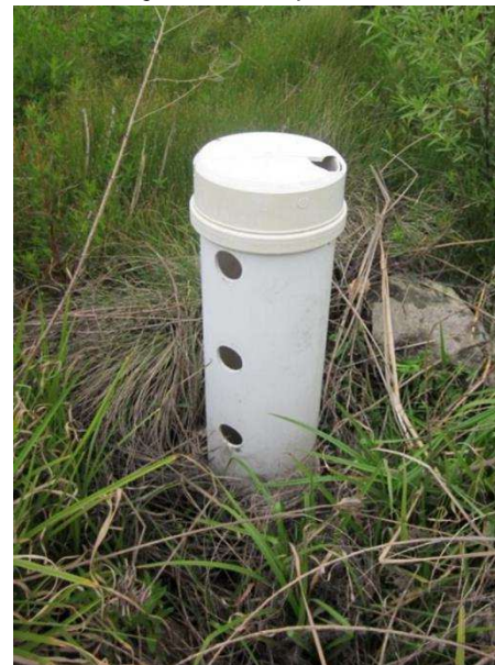
Figure 2. Variable flow outlet structure.
