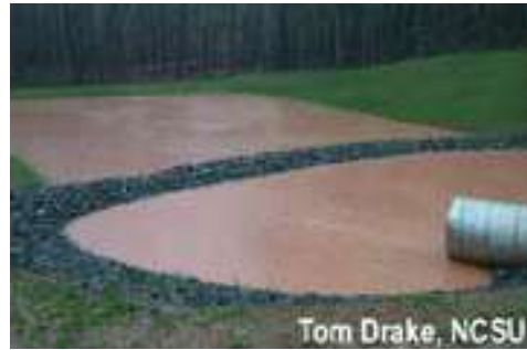
Figure 2: Forebay filled with storm water
