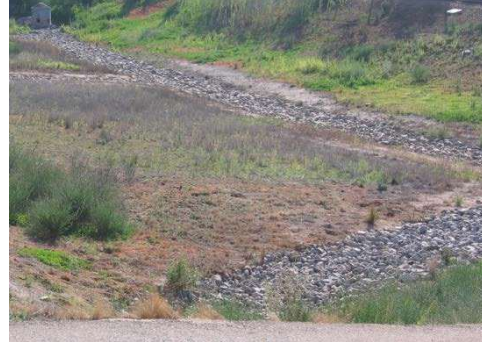
Figure 3: Gravel filled low-flow trench
