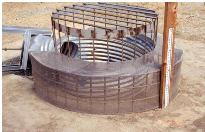
Figure 1. Example of outlet structure.
