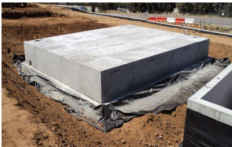
Figure 3. Subsurface design of an extended detention basin, during construction.
