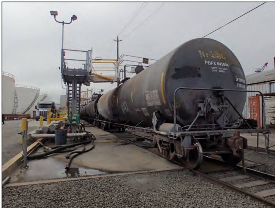
488 Wright Avenue. Railroad car fuel supply rack. View south. LSA photograph 9/26/24.
