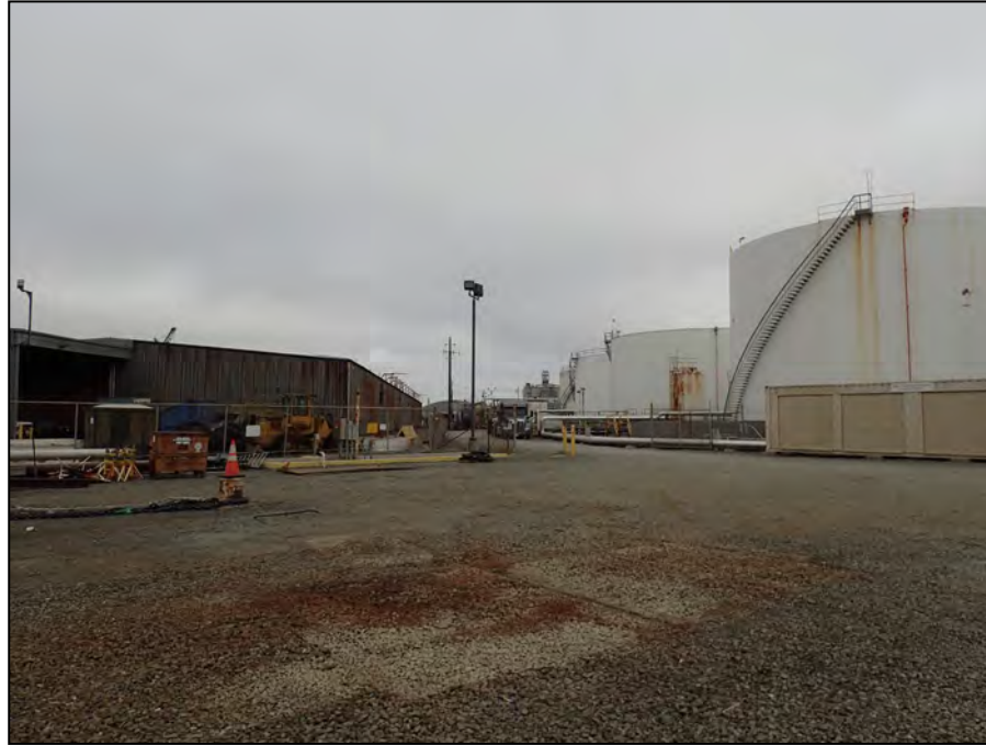
488 Wright Avenue. View north from southwestern corner of 11.5-acre property. Tanks at right, railroad car fuel rack in background. LSA photograph 9/26/24.
