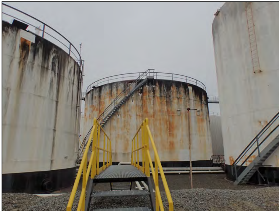
488 Wright Avenue. View west from eastern property boundary. Representative tanks, piping, and metal bridge walk over earthen berm. LSA photograph 9/26/24.
