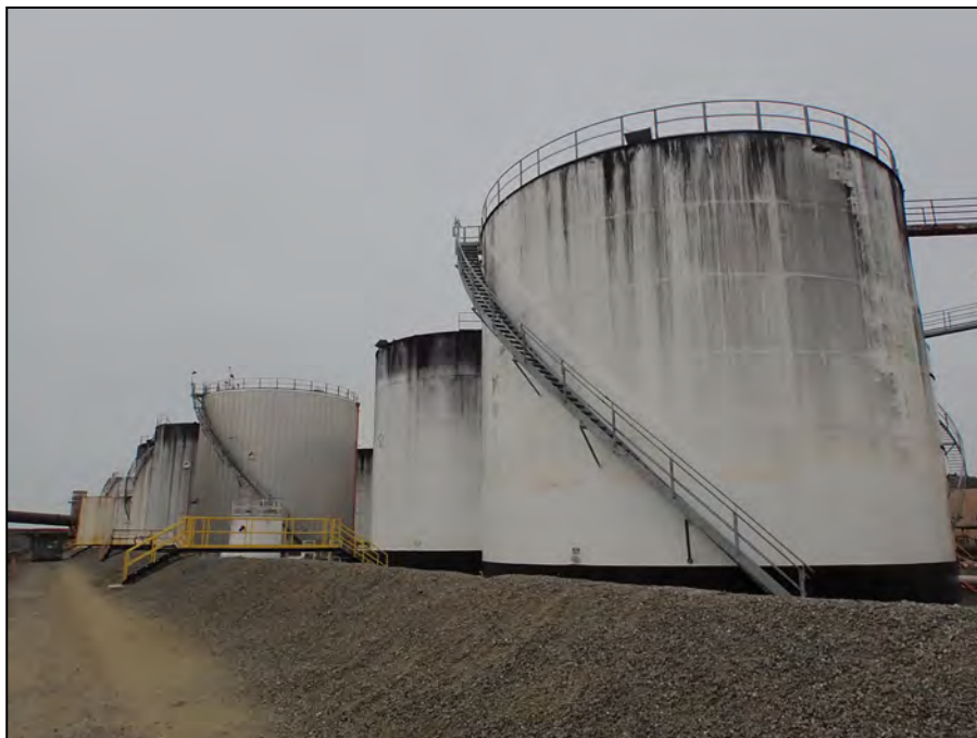
488 Wright Avenue. View south from eastern property boundary. Representative tanks, piping, and metal bridge walk over earthen berm. LSA photograph 9/26/24.
