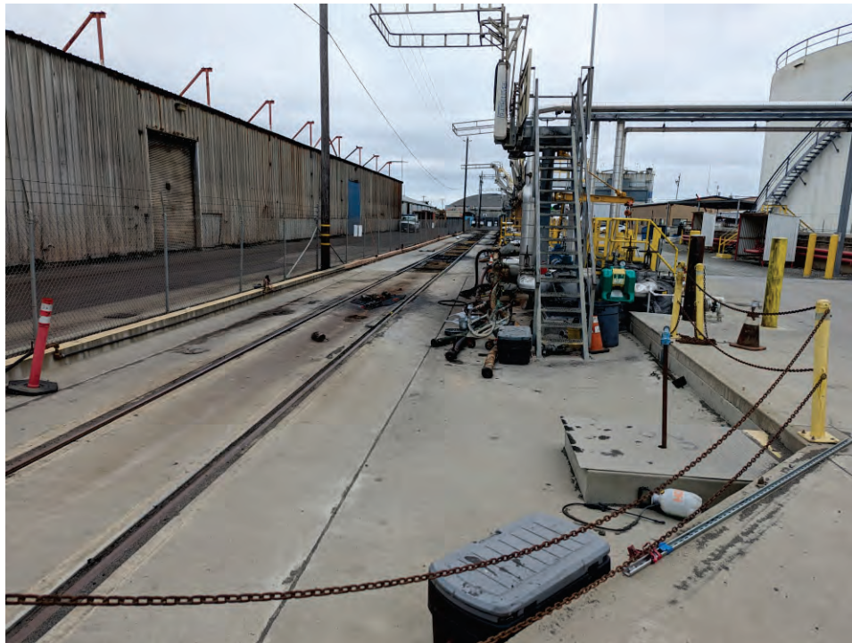
Existing Rail Lines
