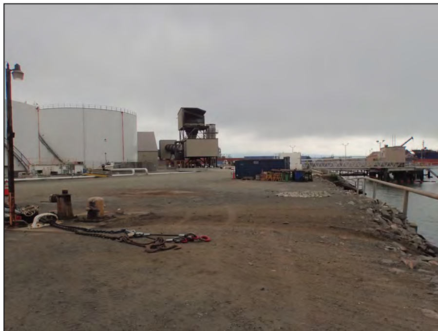
488 Wright Avenue. View east from southwestern corner of 11.5-acre property. Tanks at left, portion of marine dock at right. Cement processing plant in background. LSA photograph 9/26/24.
