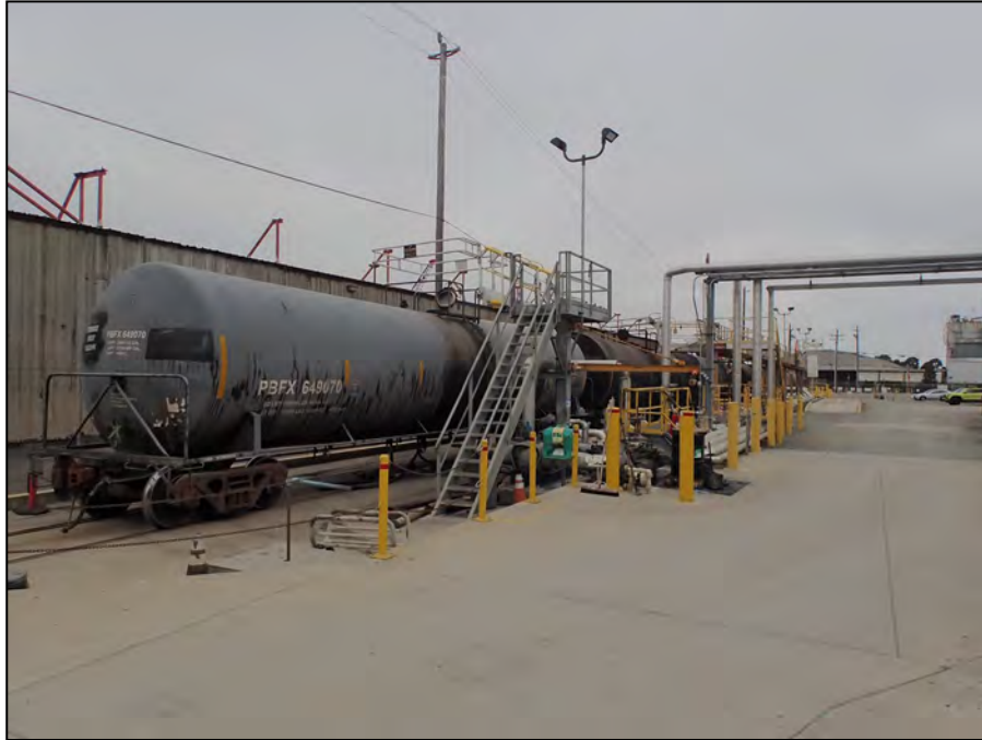
488 Wright Avenue. Railroad car fuel supply rack. View northwest. LSA photograph 9/26/24.
