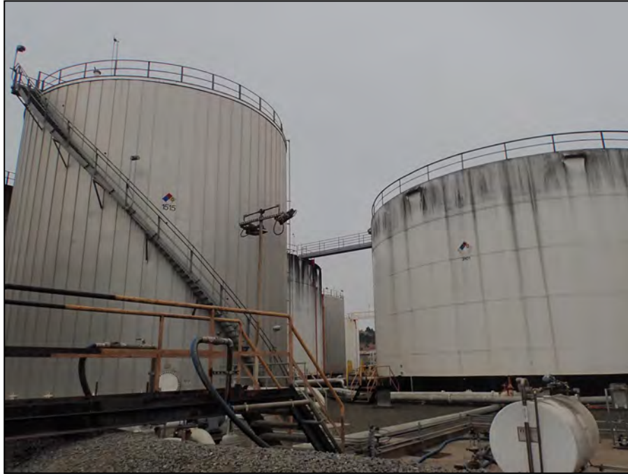
488 Wright Avenue. View west and through tank farm from eastern property boundary. LSA photograph 9/26/24.
