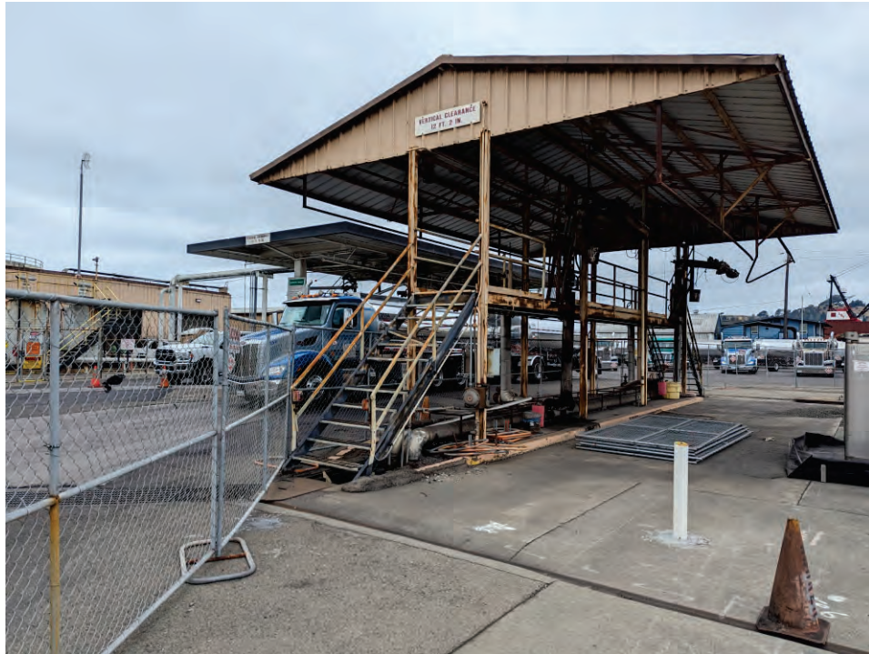
Existing Truck Rack
