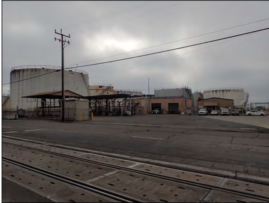
488 Wright Avenue. Asphalt and fuel supply racks at left foreground and 53,000-gallon diesel tank behind. Shop and office buildings at right. View southwest from across Wright Avenue. LSA photograph 9/26/24.
