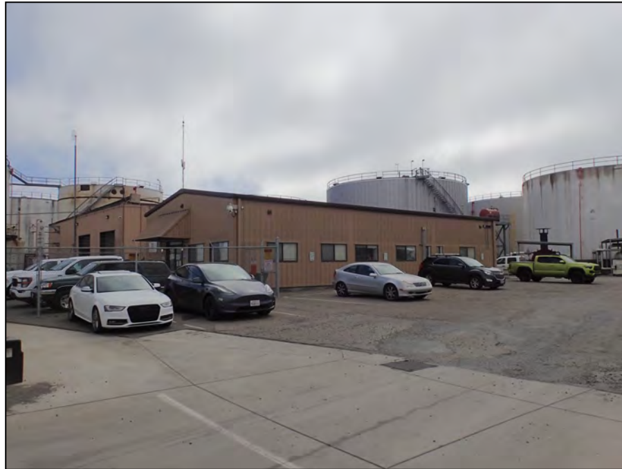
488 Wright Avenue. Office building and detached shop building (behind). View southeast. LSA photograph 9/26/24.
