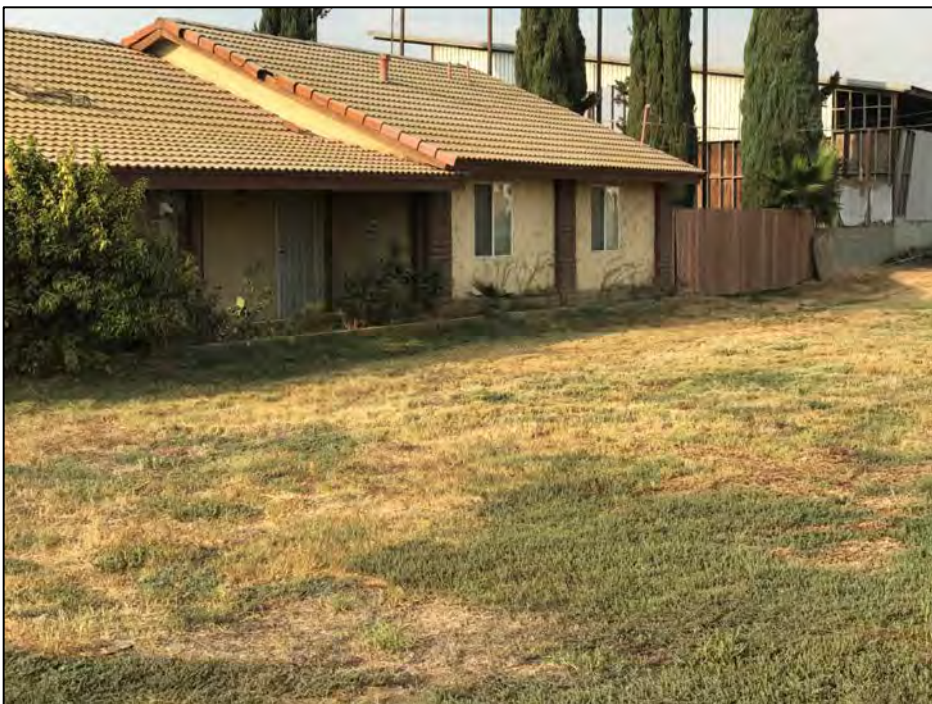
Close-up view of the recessed porch and entry of 7445 Schaefer avenue with the ancillary pole structure in the background. Source: VCS Environmental.
