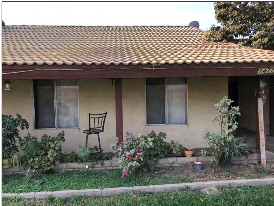
Close-up view of the north (front) elevation of 7477 Schaefer Avenue showing aluminum sash windows and the recessed porch. Source: VCS Environmental.
