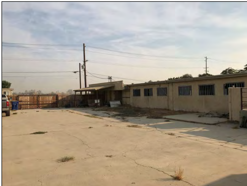
View northeast of the west elevation of the milking parlor. Source: VCS Environmental.
