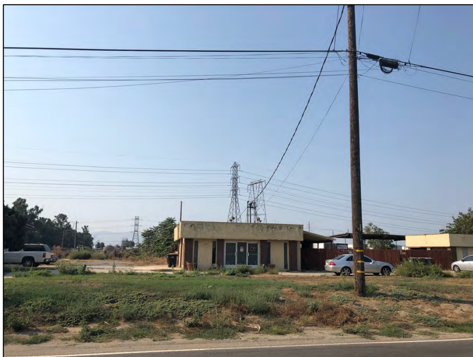
View south of the milking parlor. SCE Chino-Mira Loma 1 TL and Chino-Mira Loma 3 tower lines are partially visible to the rear. Source: Urbana Preservation & Planning, LLC.
