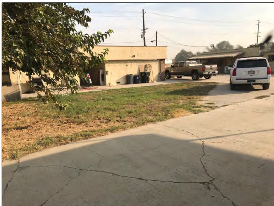
View northeast of the south elevation of the garage and the milking parlor in the background on the right. Source: VCS Environmental.
