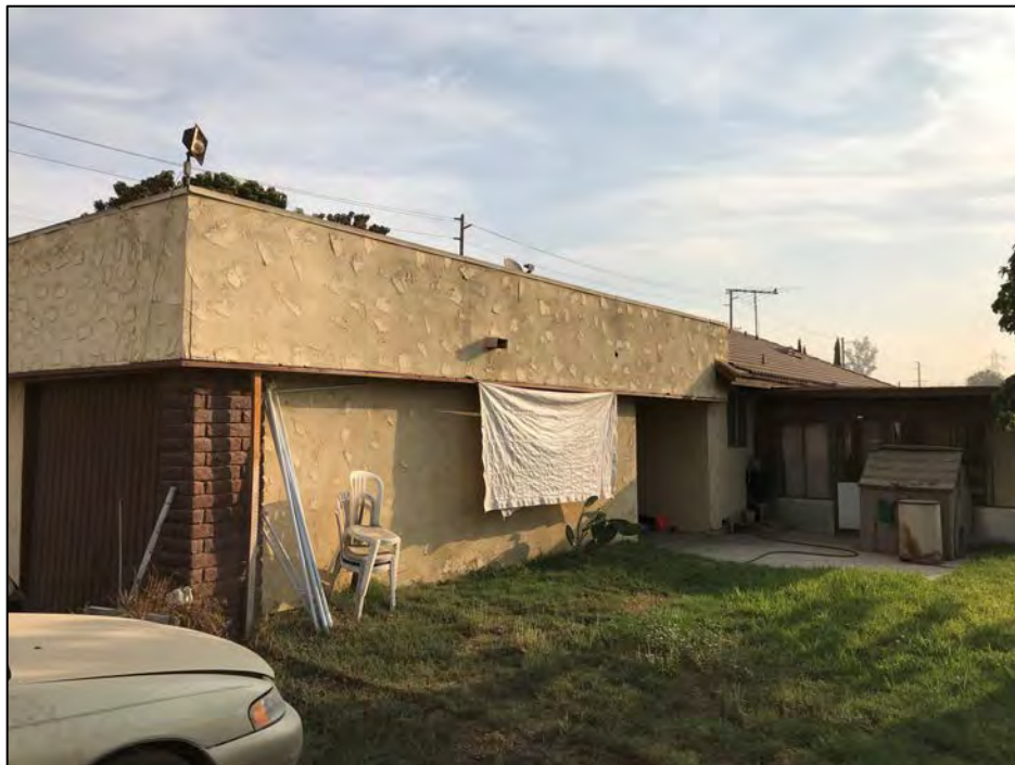
View northeast of the south and west elevations of the garage. Source: VCS Environmental.
