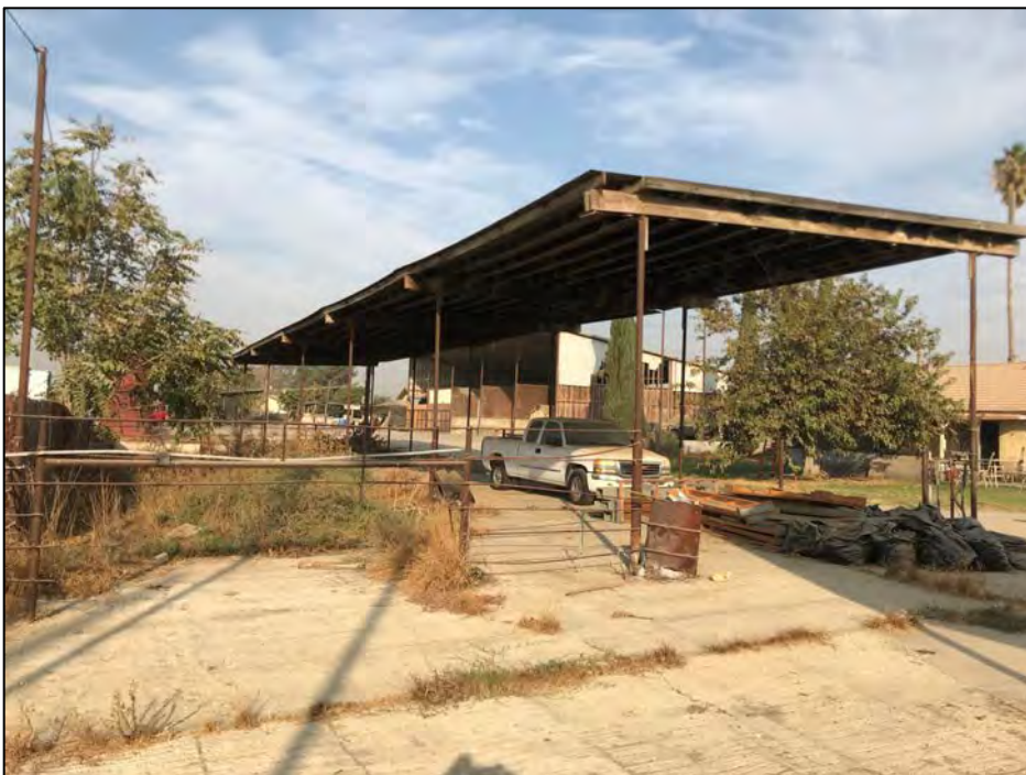
View west of a pole structure behind the dwelling. Source: VCS Environmental.
