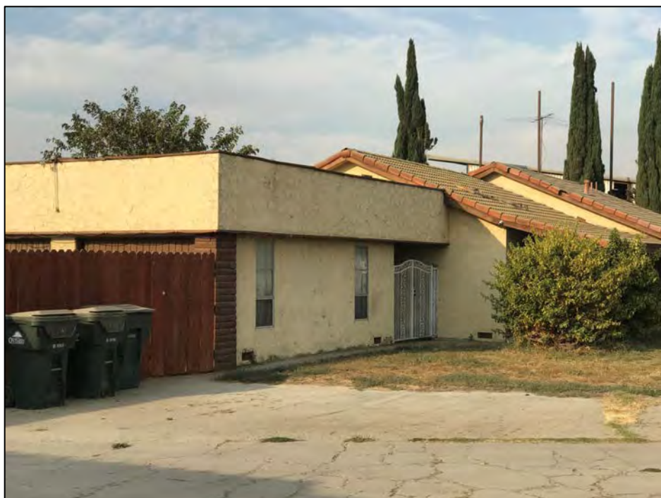
View southwest of the garage connected to the dwelling by a covered breezeway. Source: VCS Environmental.
