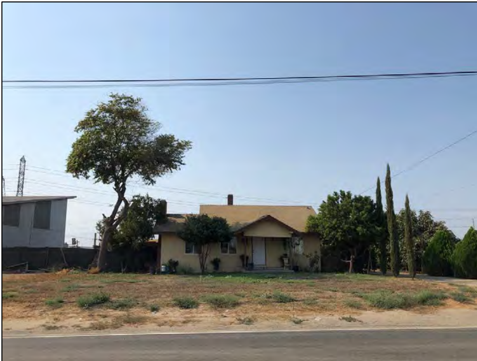
View south of the 7435 Schaefer Ave. dwelling north elevation. An ancillary building from 7445 Schaefer Avenue is partially visible east. Source: Urbana Preservation & Planning, LLC.
