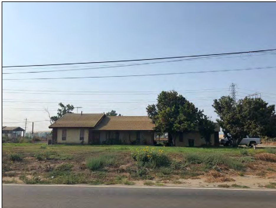
View south of the north elevation of 7477 Schaefer Ave., taken from Schaefer Avenue. Source: Urbana Preservation & Planning, LLC.
