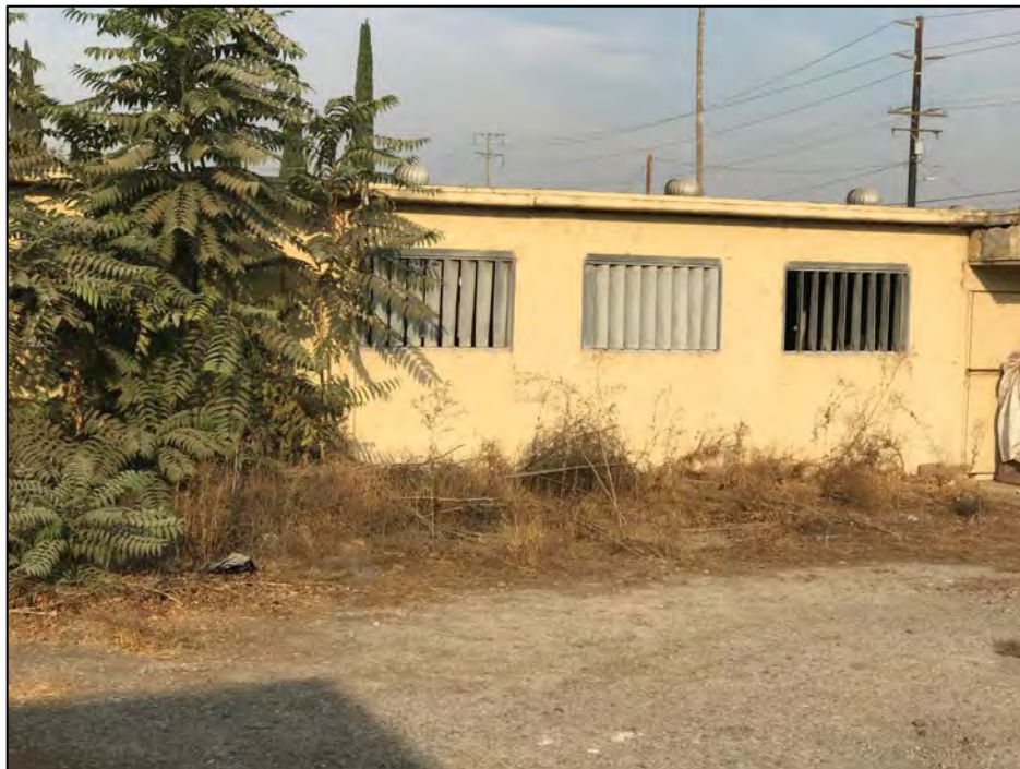
View west of the east elevation of the milking parlor showing metal louvers vent openings. Source: VCS Environmental.
