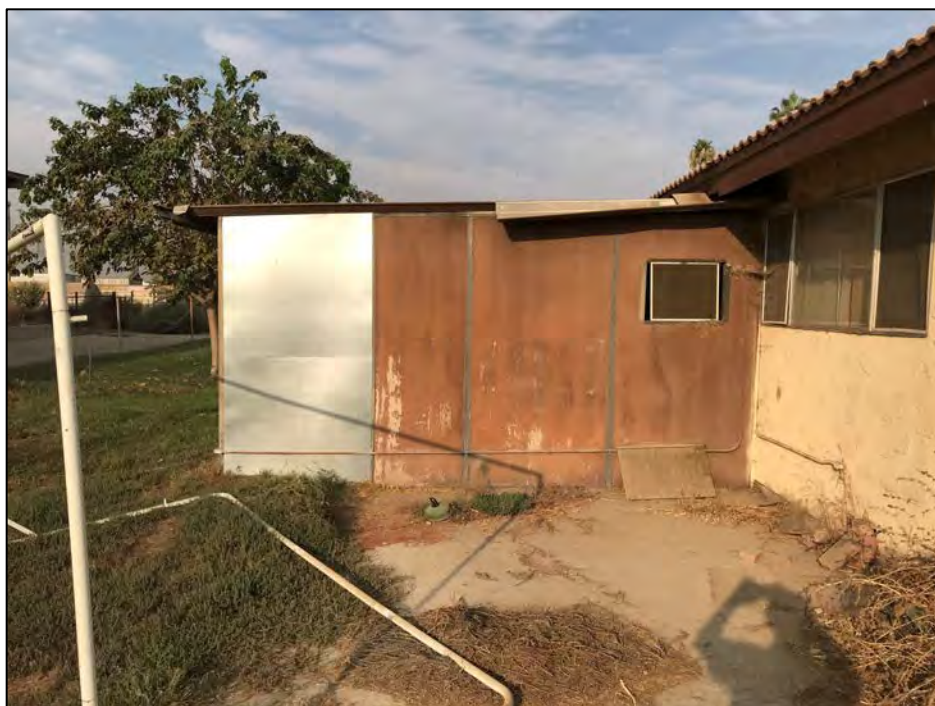
View west of the east elevation of the enclosed porch. Source: VCS Environmental.
