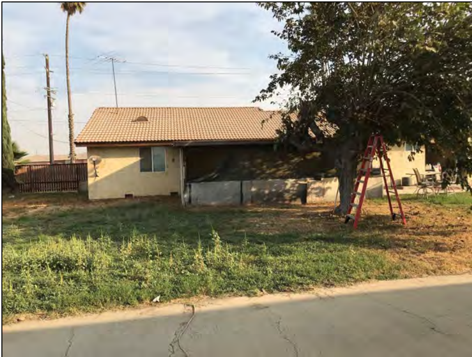
View north of the south elevation showing a rear porch. Source: VCS Environmental.
