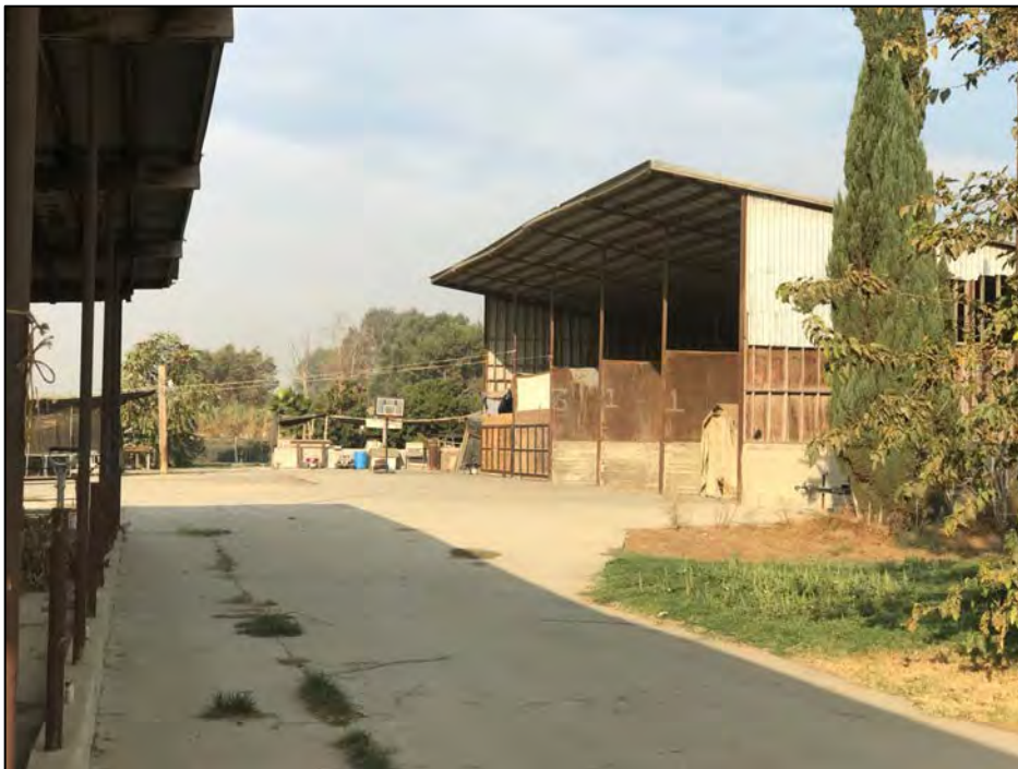
View west of the ancillary pole structure between the 7435 and 7445 Schaefer Avenue dwellings. Source: VCS Environmental.
