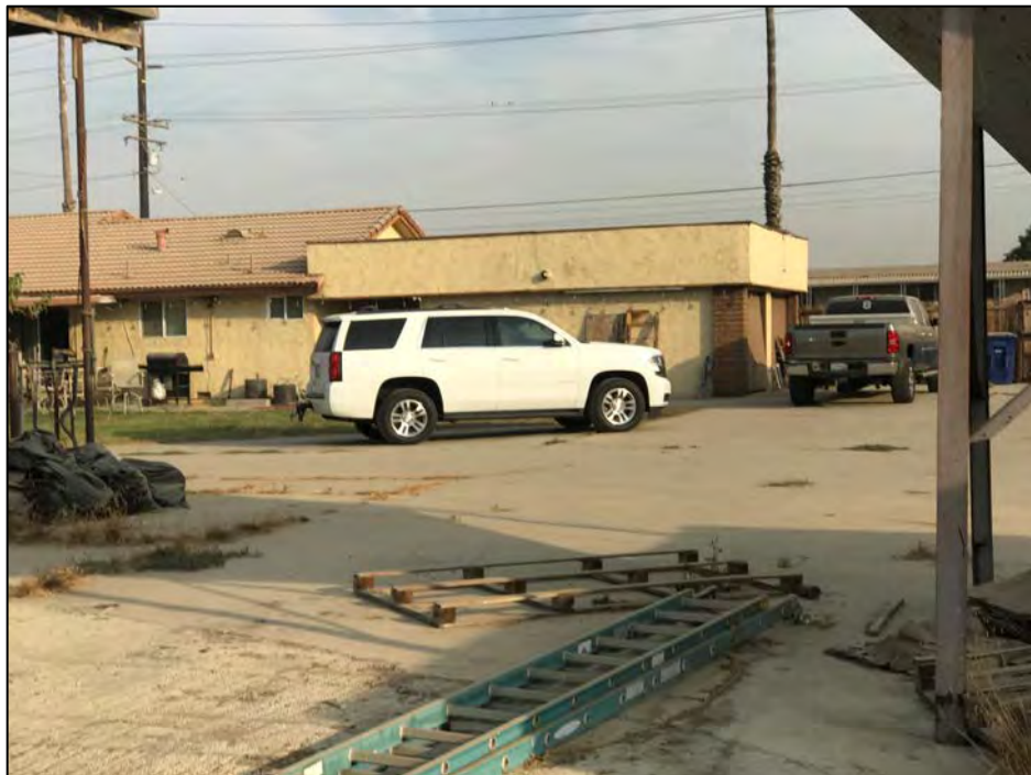
View north of the south (rear) elevation showing the garage on the right attached to the dwelling on the left. Source: VCS Environmental.
