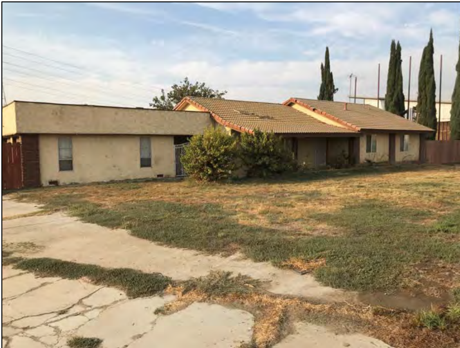
View southwest of the north (front) elevation of 7445 Schaefer Ave. Source: VCS Environmental.
