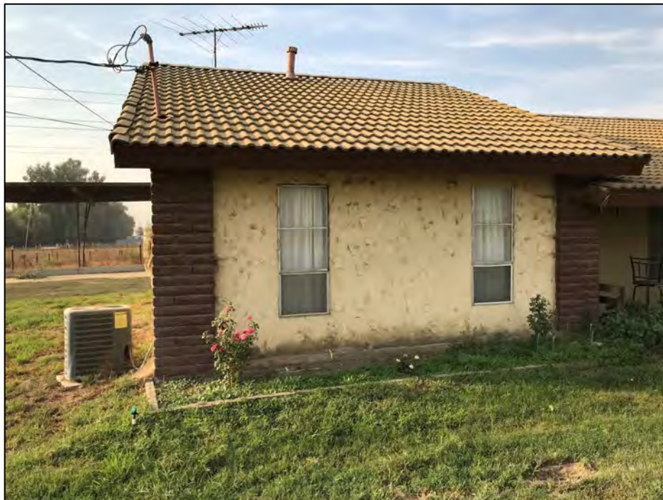
View south of the north elevation showing aluminum sash windows and stucco siding. Source: VCS Environmental.
