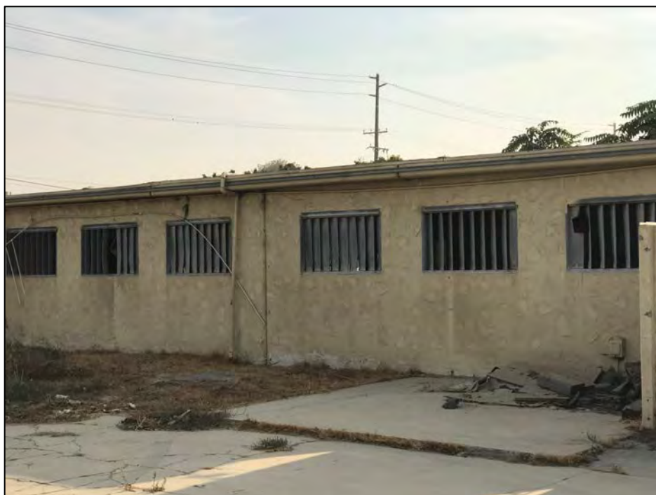
Close-up view of the west elevation showing metal louver vent openings. Source: VCS Environmental.
