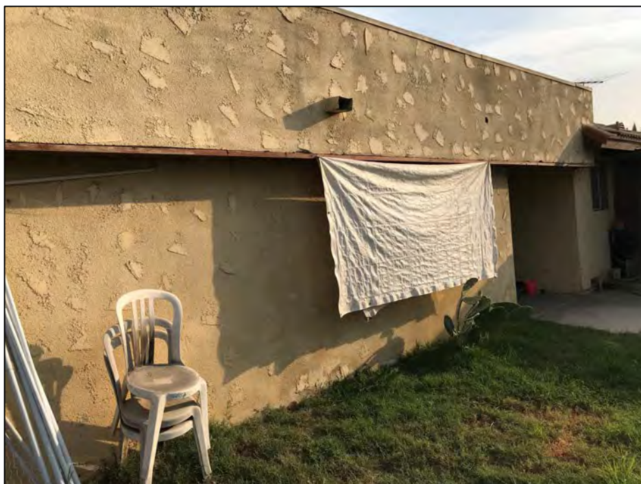
Close-up view of the south elevation of the garage. Source: VCS Environmental.
