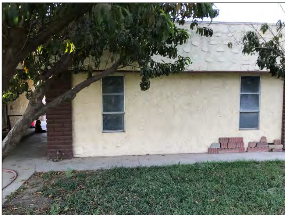
Close-up view of the garage attached to the 7477 Schaefer Avenue dwelling by a covered breezeway. Source: VCS Environmental.
