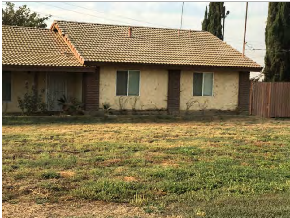
Close-up view of the aluminum sash windows and decorative brick pilasters. Source: VCS Environmental.
