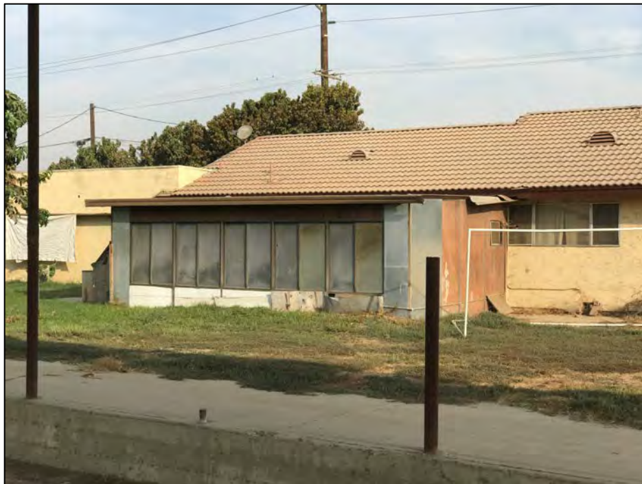
View north of the rear porch on the south elevation enclosed at an unidentified date. Source: VCS Environmental.
