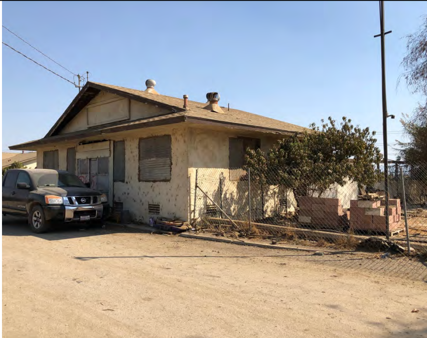
View southeast of the west and north elevations of the milking parlor. Source: Urbana Preservation & Planning, LLC.
