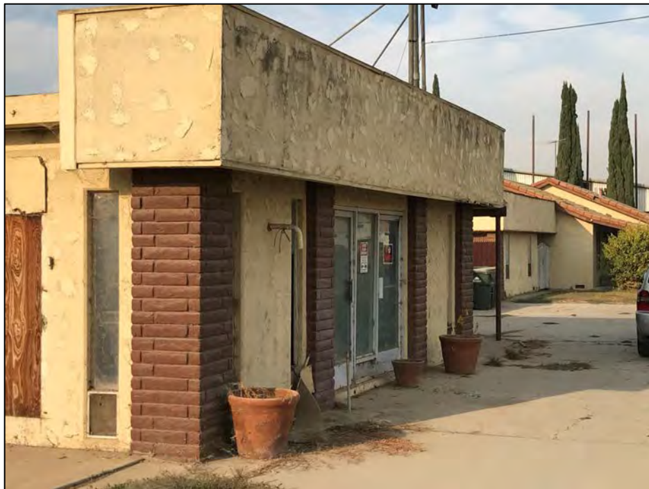
View west of the north (front) and east elevations of the milking parlor showing the parapet and brick pilasters. Source: VCS Environmental.
