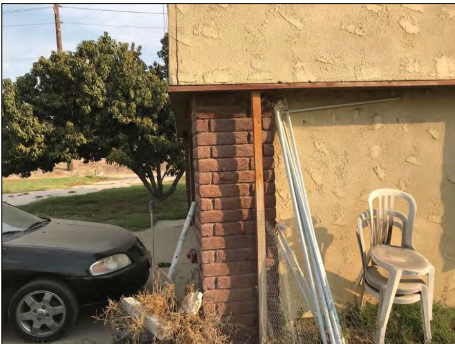
Close-up view of the brick corner quoins / pilasters of the garage's south elevation. Source: VCS Environmental.
