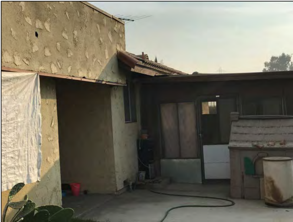
Close-up view of the covered breezeway between the dwelling and garage and the west elevation of the rear porch. Source: VCS Environmental.
