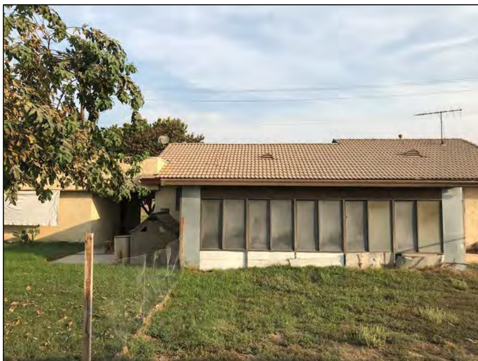
View north of the south elevation showing the enclosed porch. Source: VCS Environmental.
