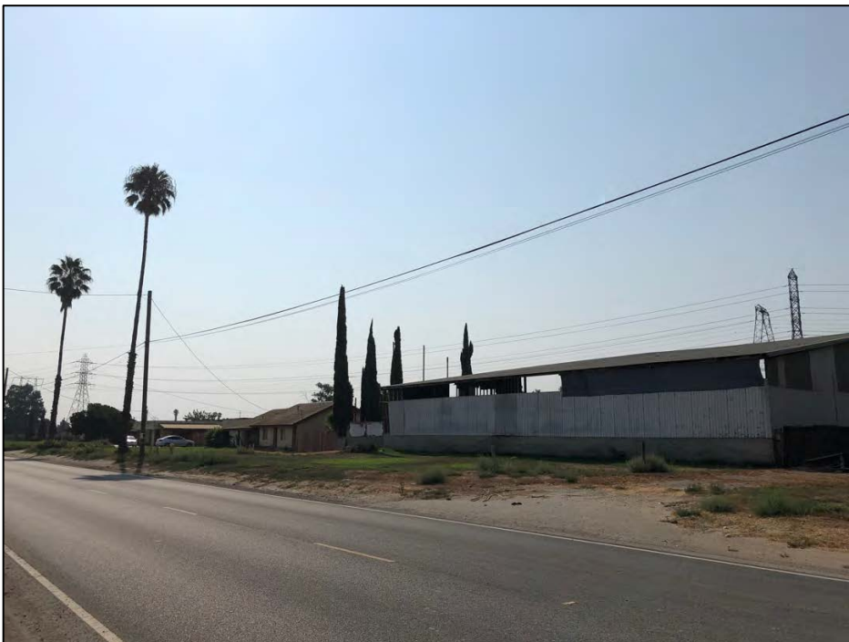
View southeast of an ancillary pole structure and 7445 Schaefer Ave., taken from Schaefer Avenue. Source: Urbana Preservation & Planning, LLC.
