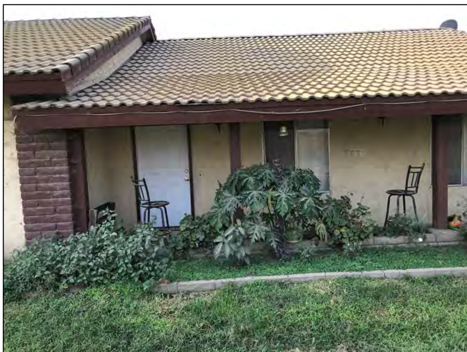
Close-up view of the north elevation showing the entrance and brick corner quoins / pilasters. Source: VCS Environmental.
