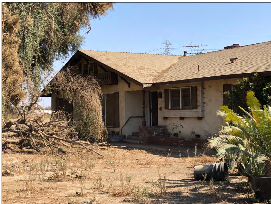
Close-up view of the façade showing the wood sash windows, faux balcony, brick planters, and turned wood porch post. Source: Urbana Preservation & Planning, LLC.
