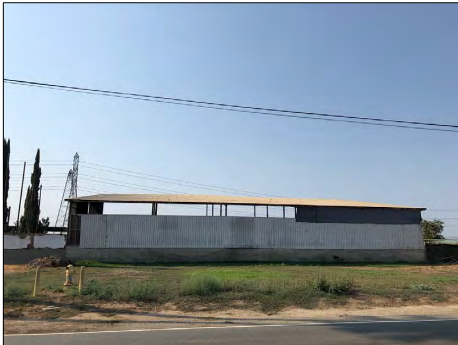
View south of an ancillary pole structure just west of 7445 Schaefer Ave., taken from Schaefer Avenue. Source: Urbana Preservation & Planning, LLC.
