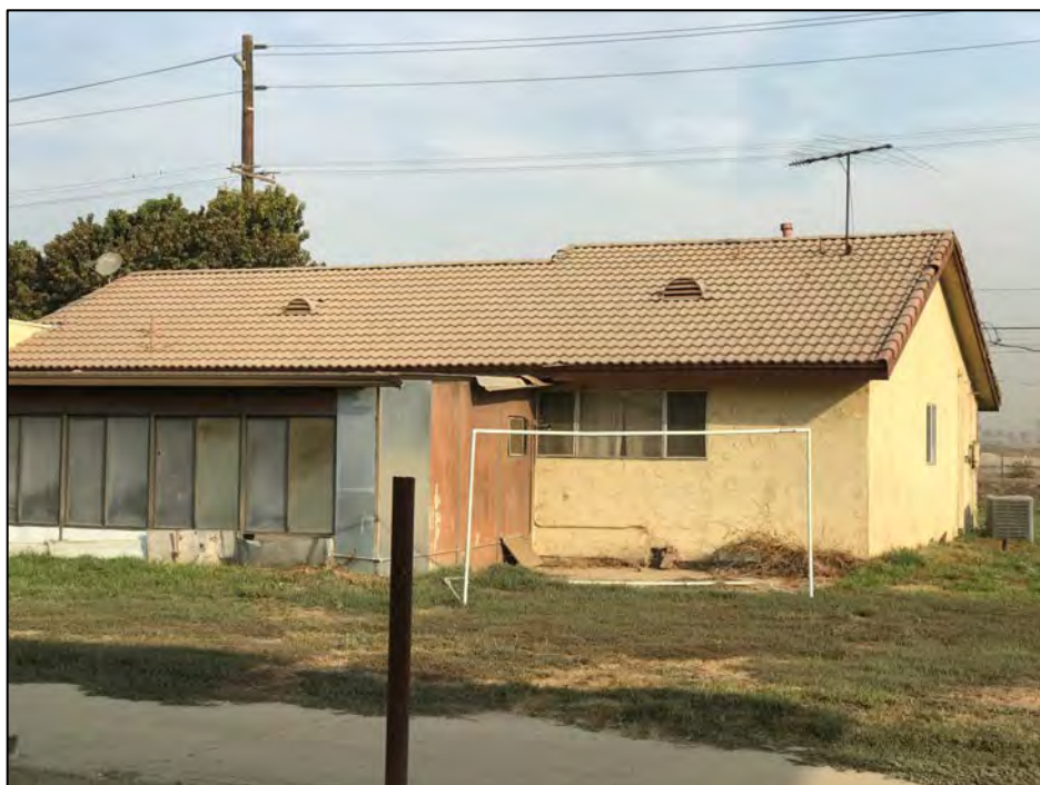
View north of the south (rear) elevation showing an enclosed rear porch. Source: VCS Environmental.
