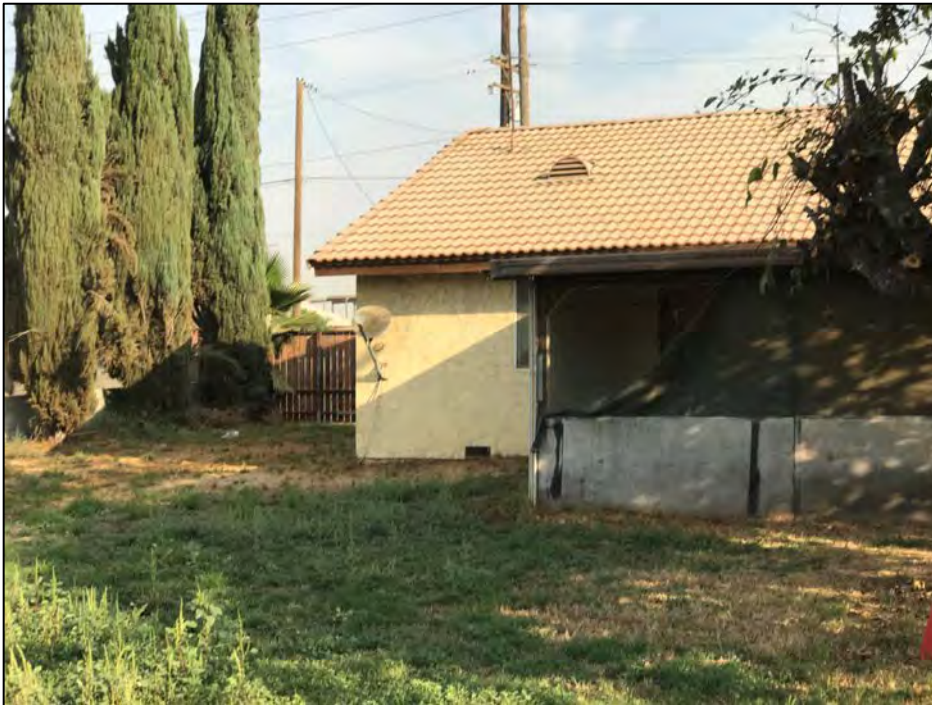
View northwest of the south elevation. Source: VCS Environmental.
