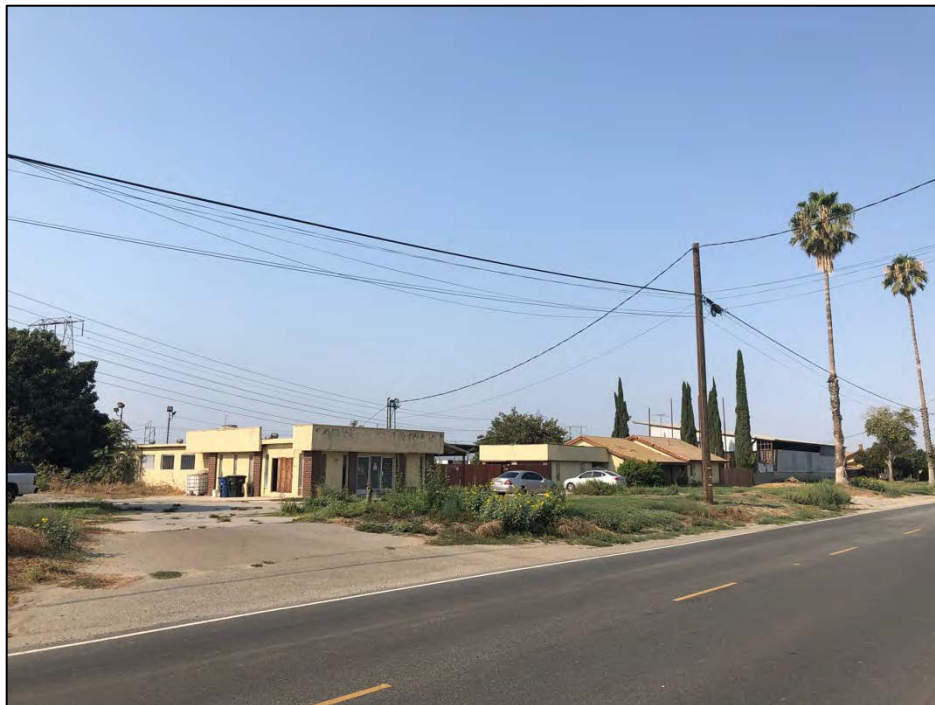
View southwest of 7445 Schaefer Avenue including the milking parlor and ranch style dwelling, taken from Schaefer Avenue. Source: Urbana Preservation & Planning, LLC.
