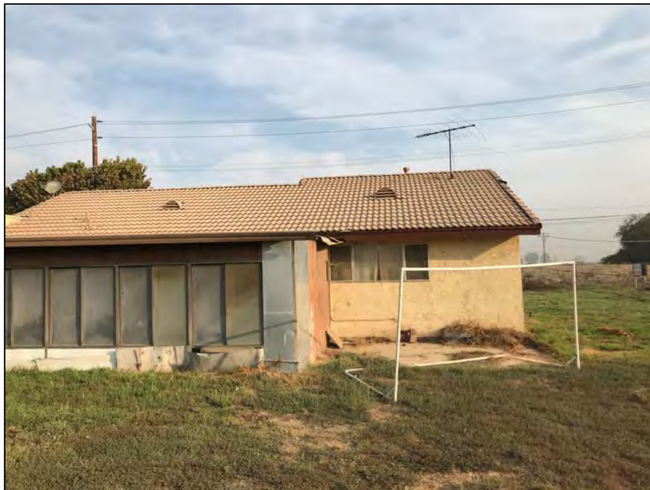
View north of the south elevation of 7477 Schaefer Avenue. Source: VCS Environmental.
