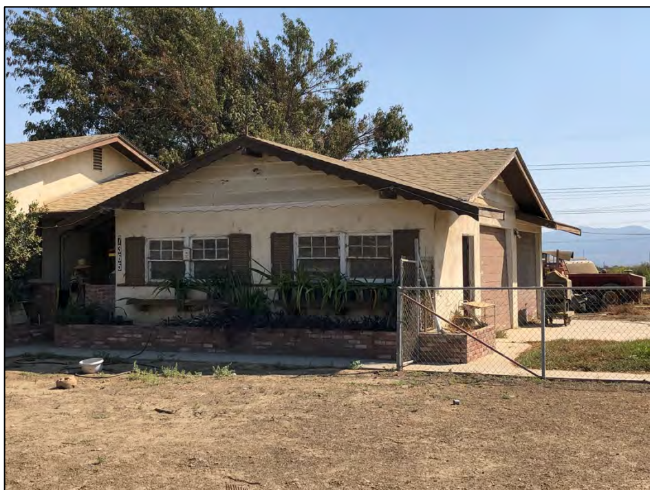
Close-up view of the garage showing the wood sash windows, shutters, scalloped edges, and brick planters. Source: Urbana Preservation & Planning, LLC.
