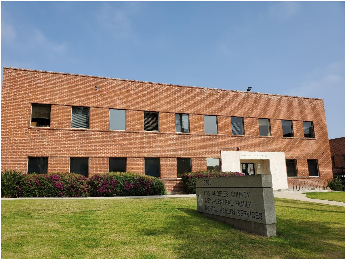
Figure 16 3751 Stocker Street, Primary Elevation, Lawn and Sign Monument
