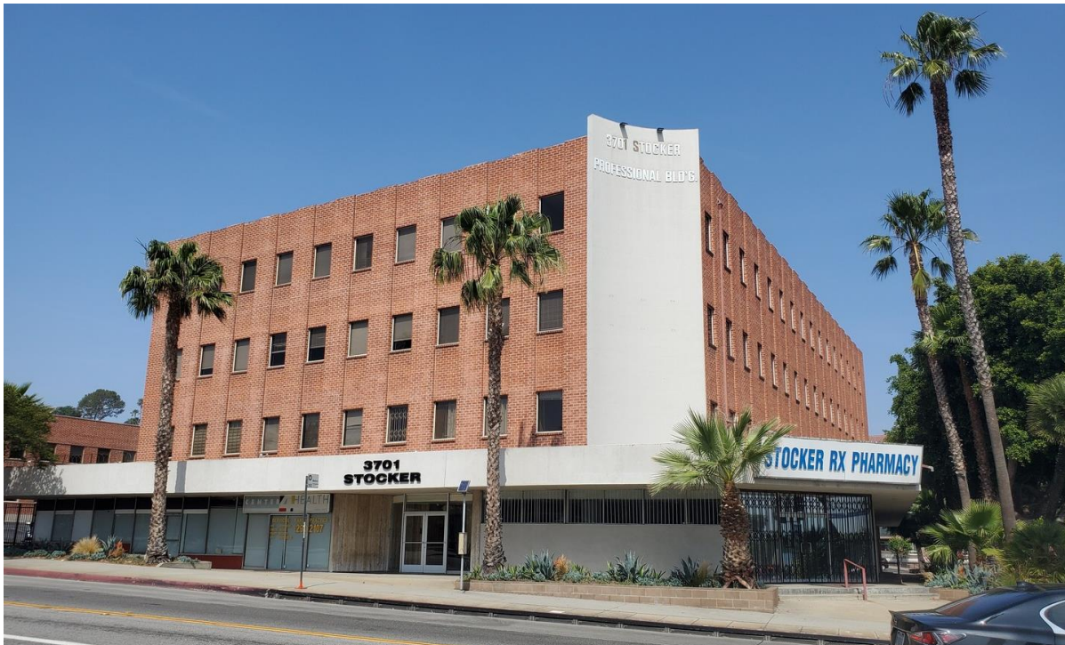
Figure 11 3701 Stocker Street’s Primary Façade, View East
