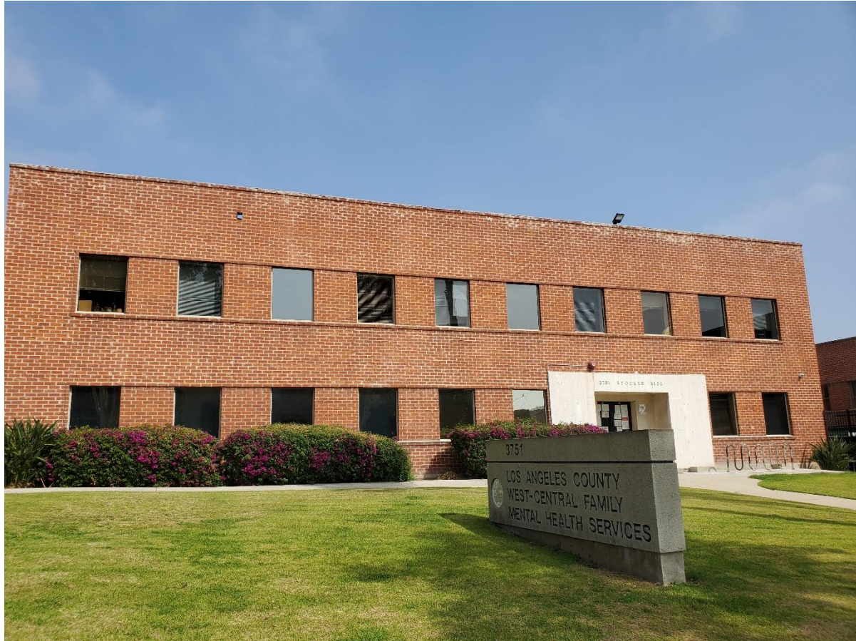
Photograph 5 3751 Stocker Street, Primary Elevation, Lawn and Sign Monument
