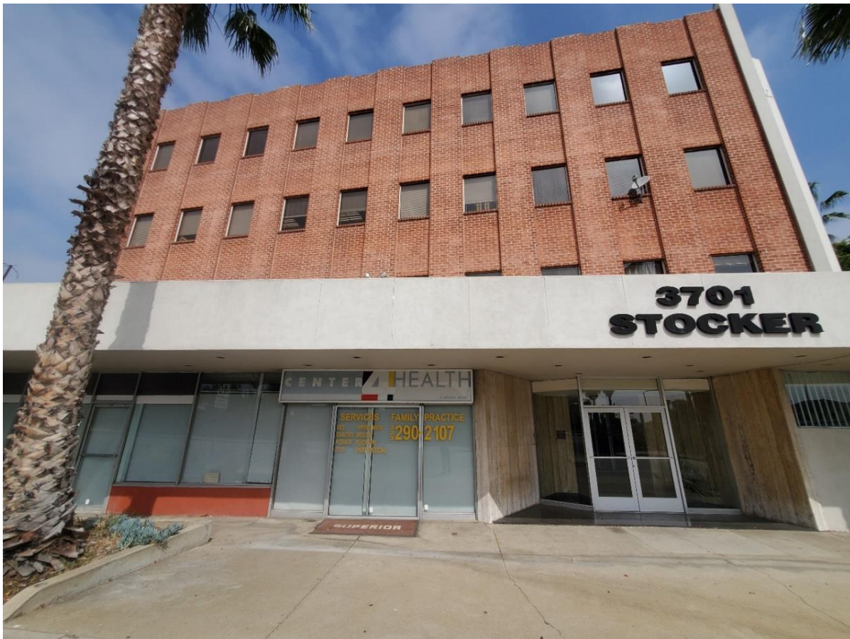
Figure 13 3701 Stocker Street Main Entrance, View Northwest
