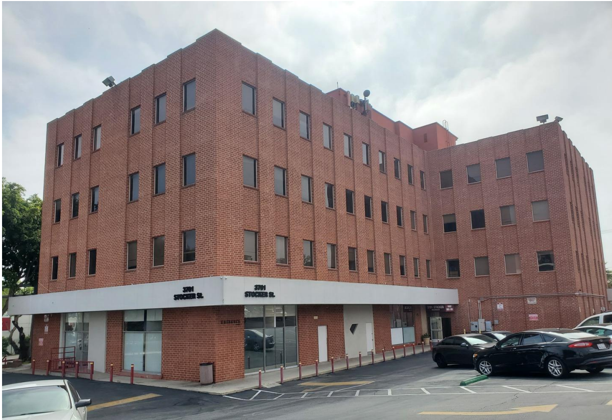
Figure 12 3701 Stocker Street's Rear Elevation, View Southeast
