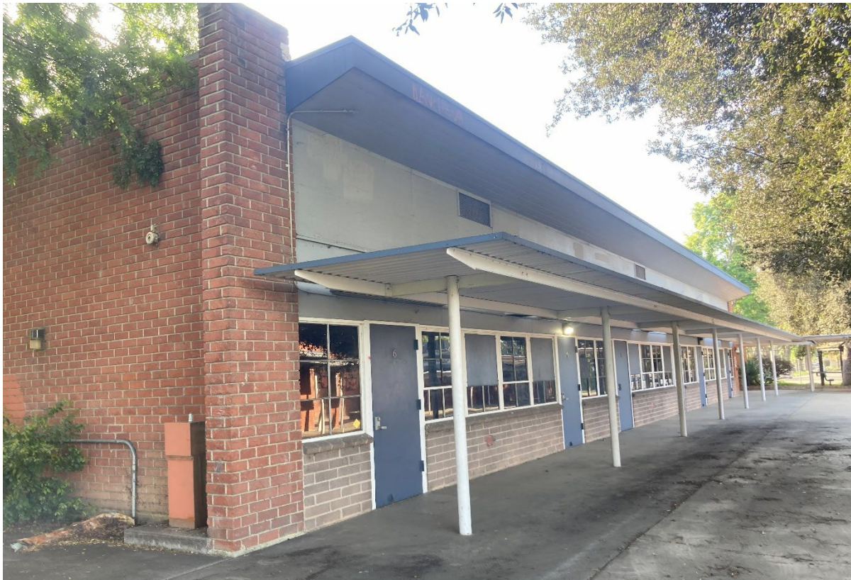
Figure 7 Del Norte School Covered Walkway and Classrooms, View North
