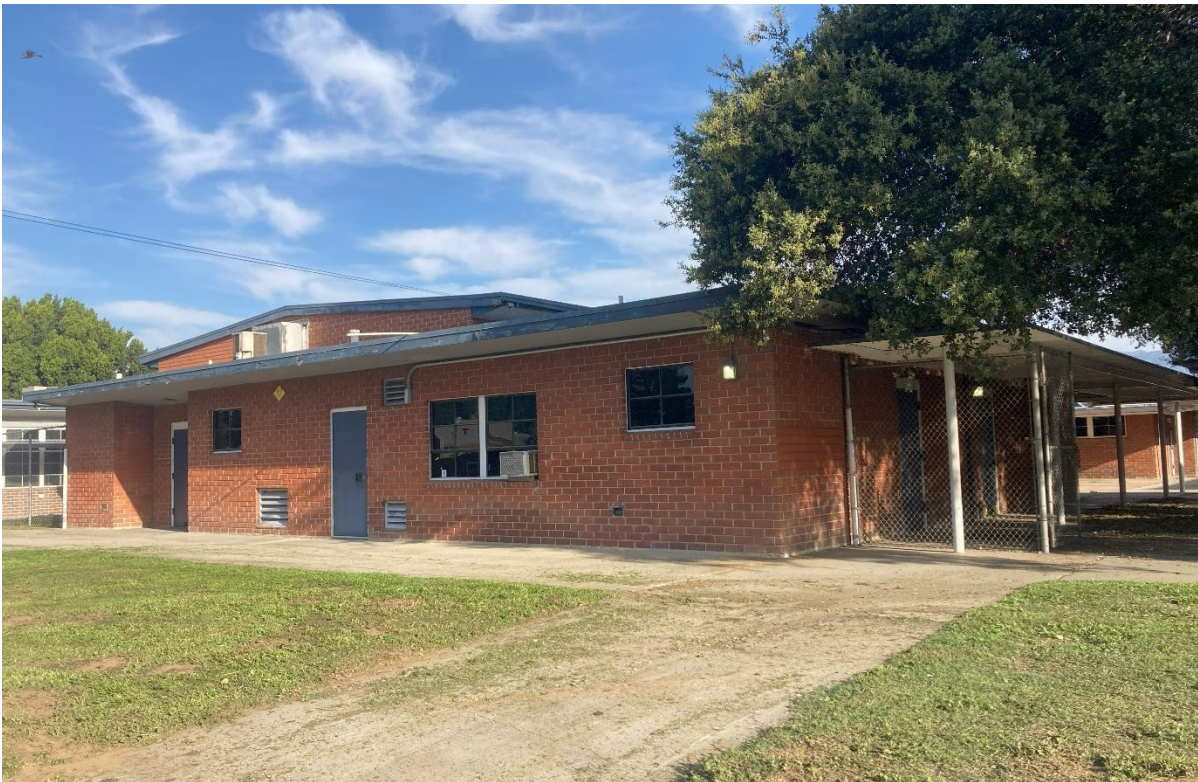
Figure 5 Del Norte School Buildings Clad in Brick with Flat or Gabled Roofs, View North
