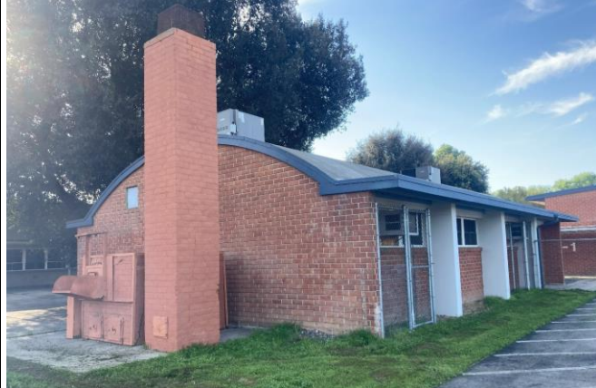
Figure 4 Del Norte School Covered Walkway and Classrooms, View North
