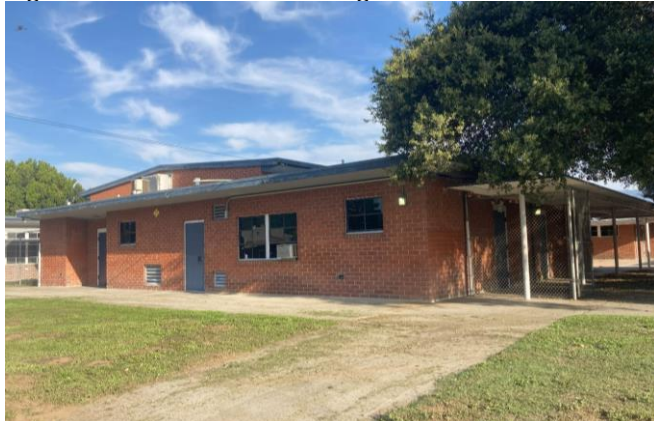
Figure 2 Del Norte School Buildings Clad in Brick with Flat or Gabled Roofs, View North
