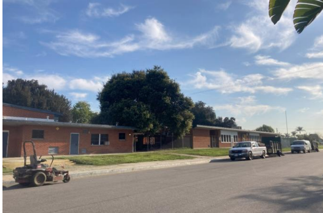
Figure 1 Del Norte School Primary (South) Elevation, View Northeast
