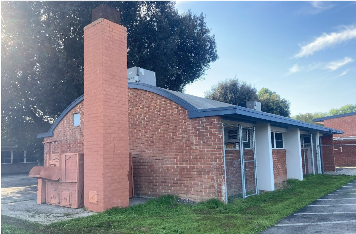
Figure 6 Del Norte School Domed Roof Building and Furnace, View Southeast
