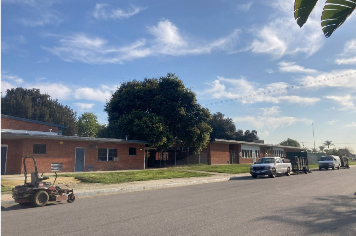
Figure 4 Del Norte School Primary (South) Elevation, View Northeast
