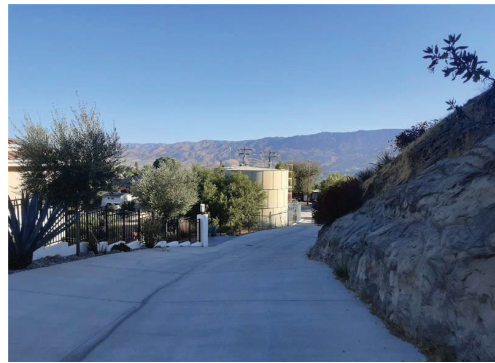
Photograph 2. Existing paved access road adjacent to Alta Vista Tank No. 1, facing north toward the Alta Vista tanks and nearby residence.
