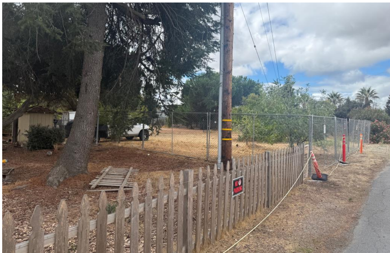
Photograph 7 Condit Sports Facilities Expansion site, View to the southwest
