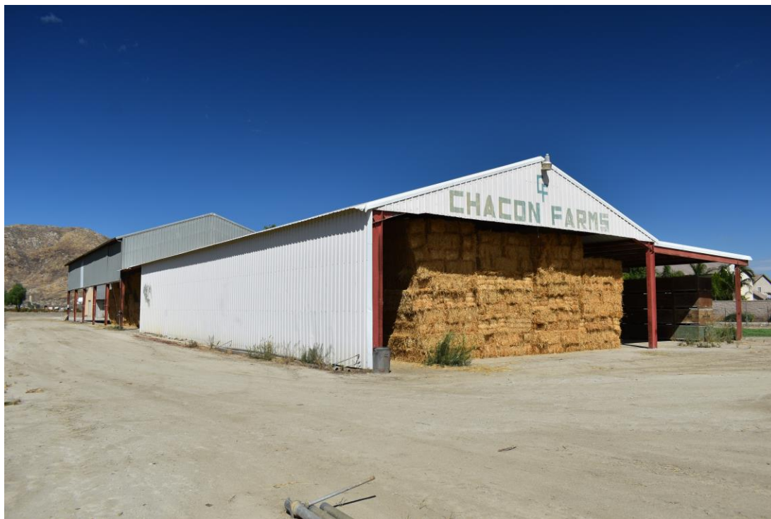
Exhibit 11. Overview of Barns 1 and 2, with Barn 2 in foreground, facing northwest.
