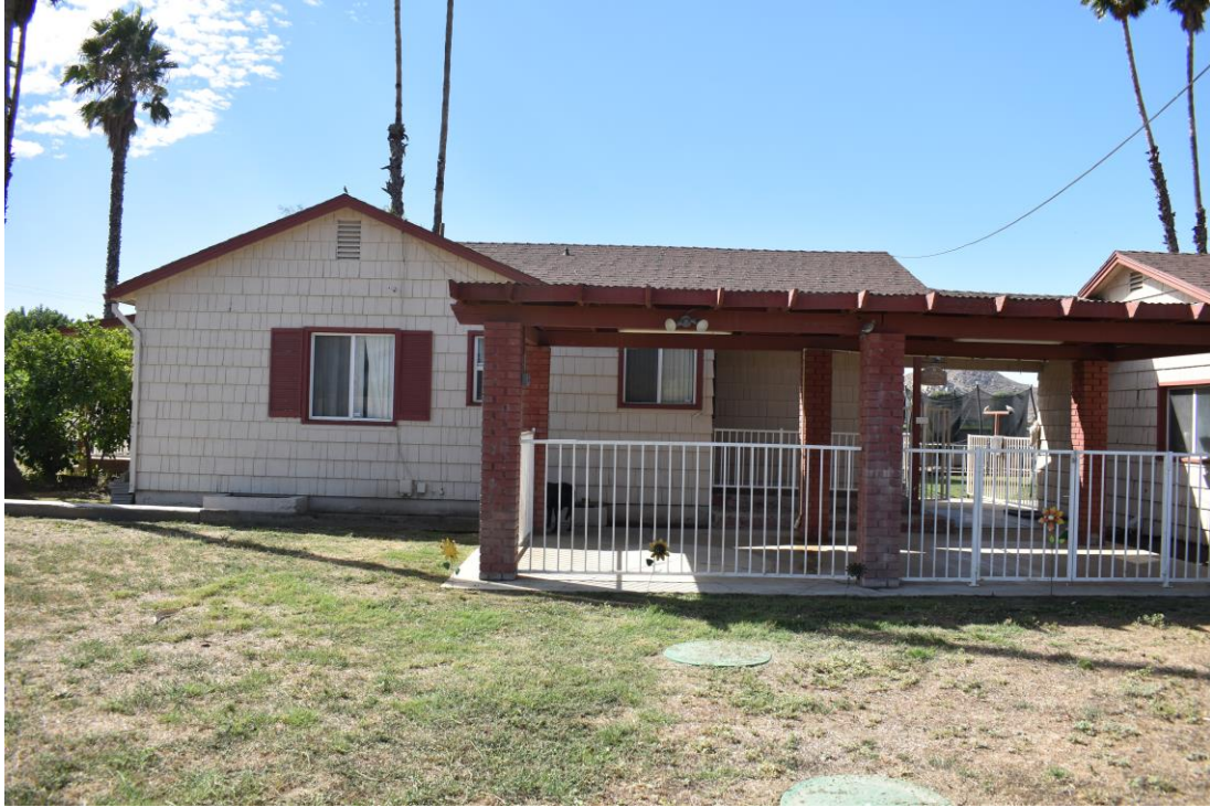
Exhibit 4. Overview of north elevation of Residence 1, with patio area and breezeway, facing south.
