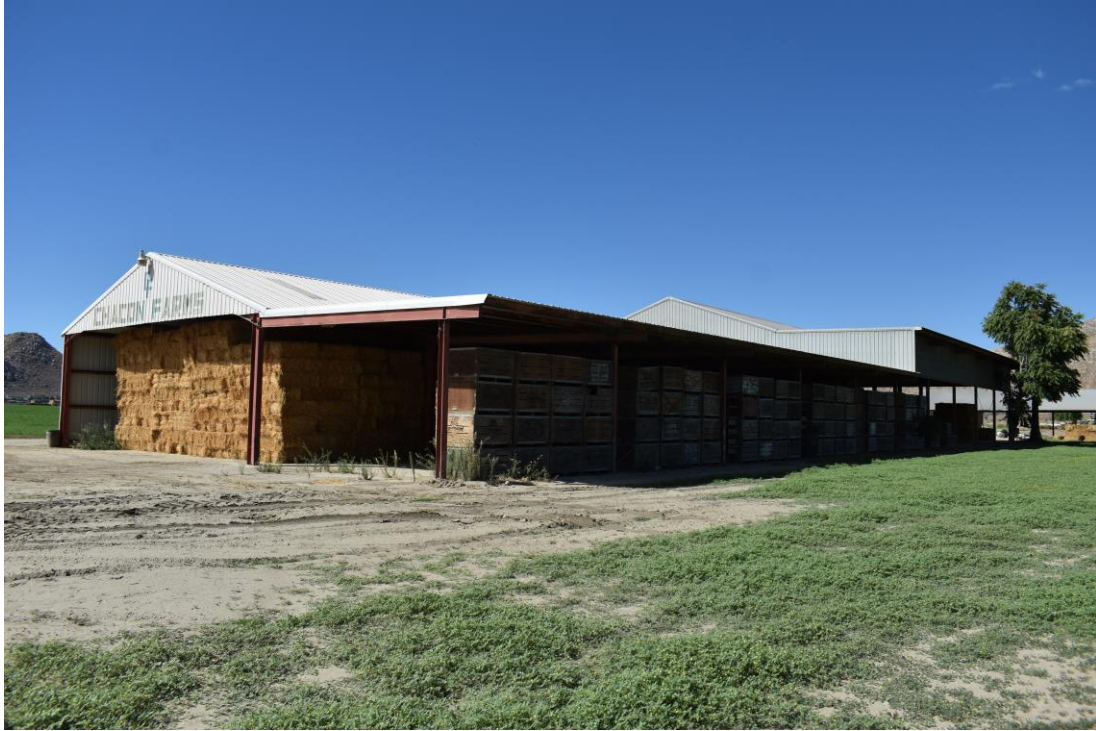
Exhibit 13. Overview of Barns 1 and 2, with Barn 2 in foreground, facing southwest.
