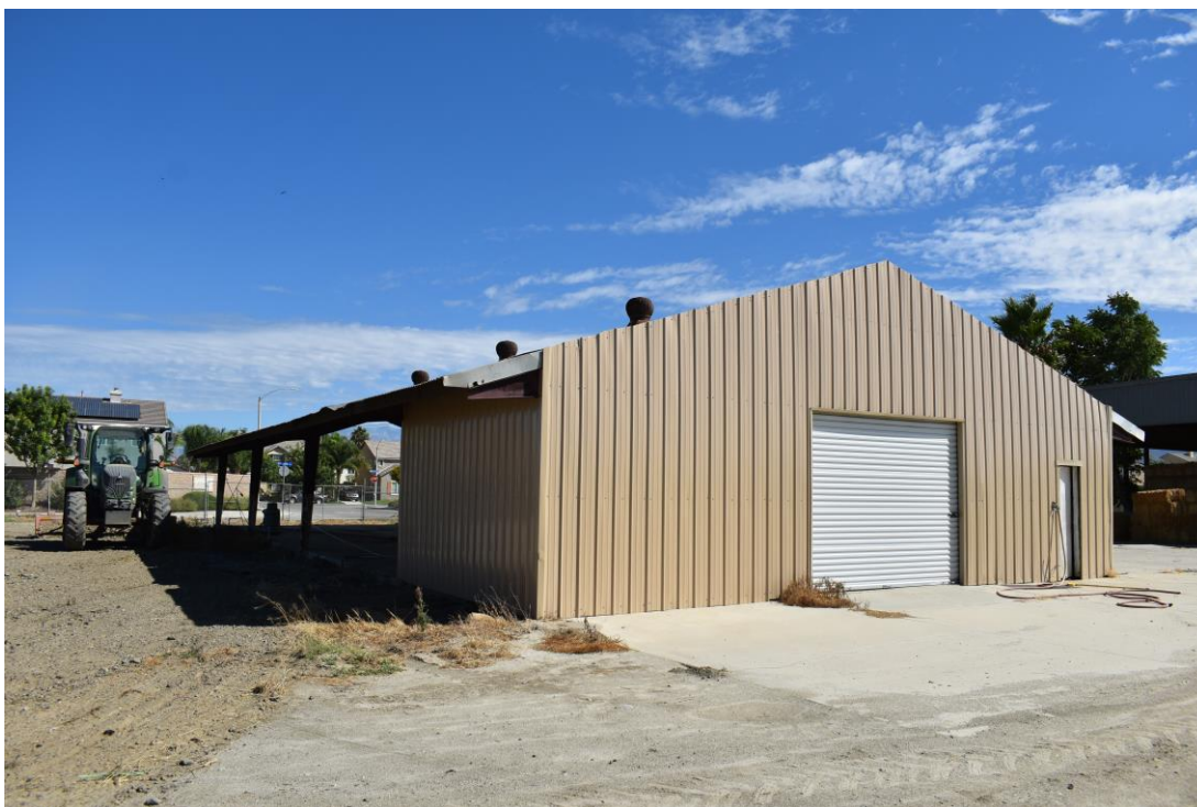
Exhibit 15. Overview of south elevation of Tool Shed, facing northeast.
