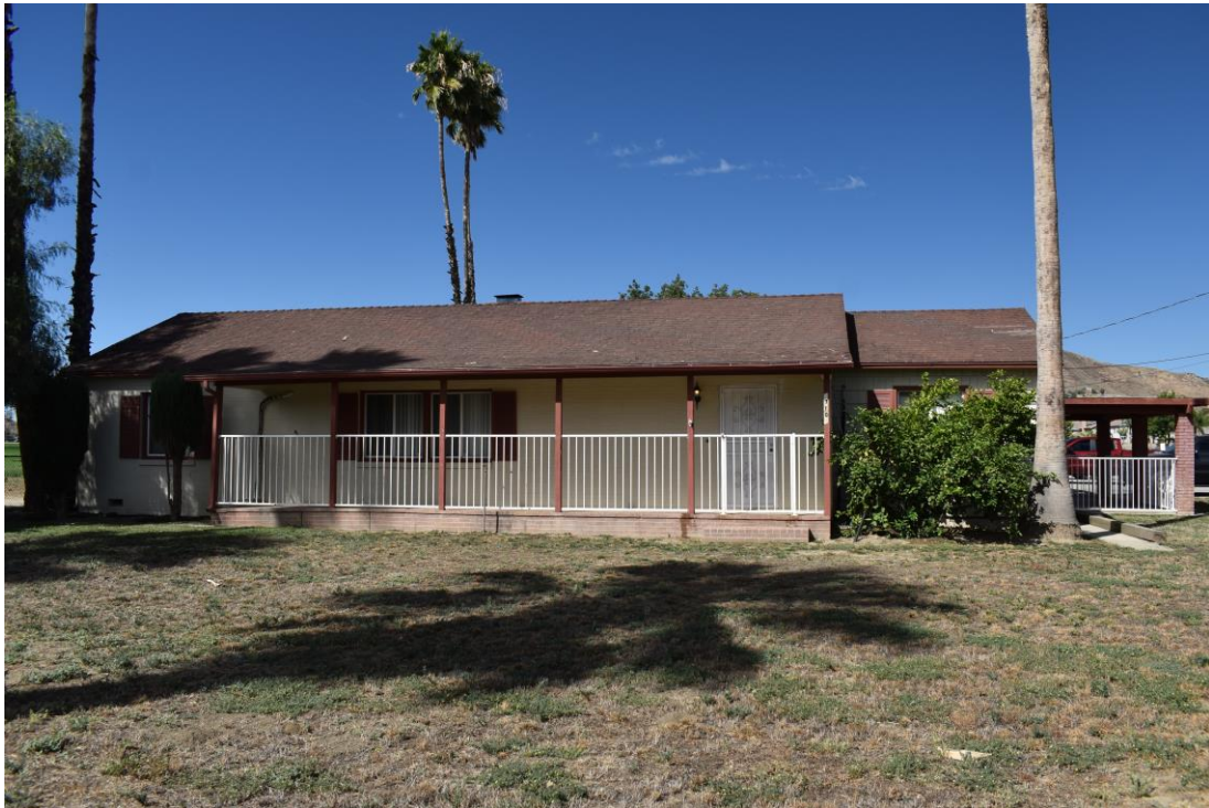
Exhibit 1. Overview of primary (east) elevation of Residence 1, facing west.
