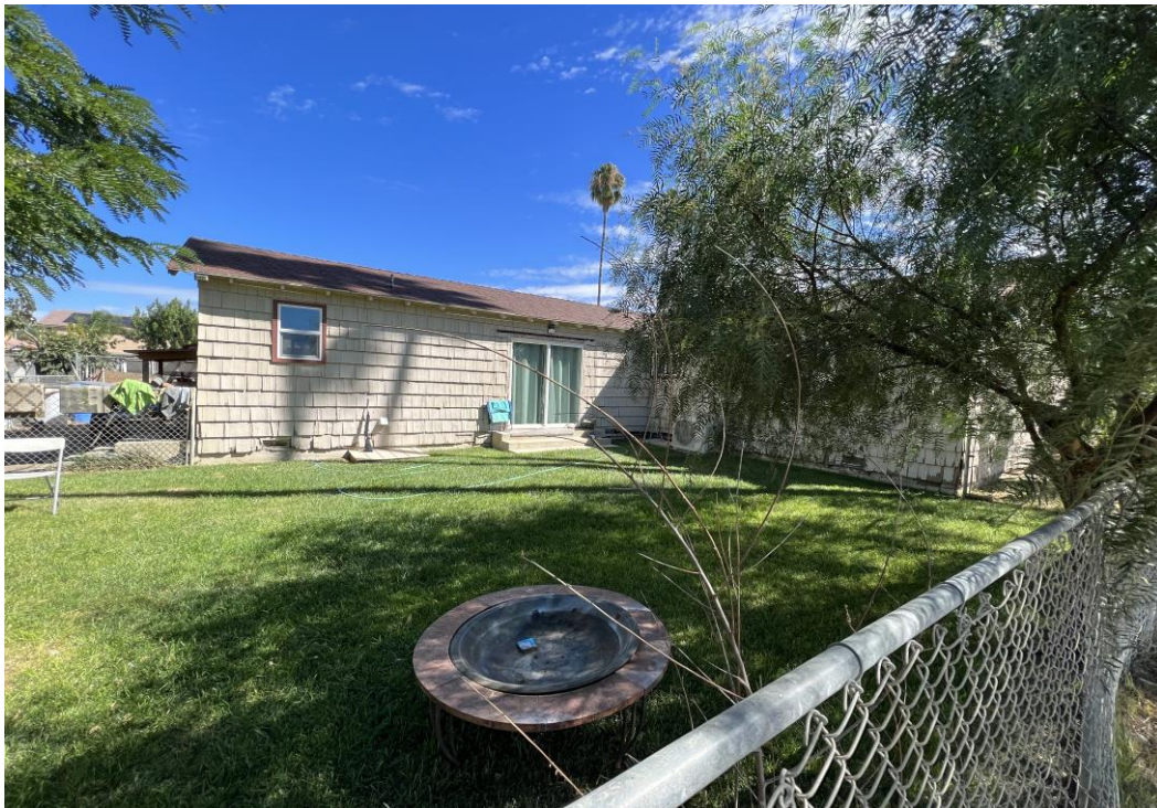
Exhibit 9. Overview of south and west elevation of Residence 2, facing northeast.
