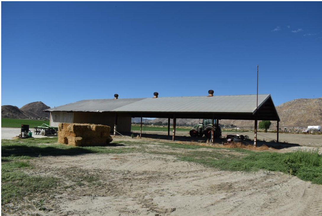
Exhibit 14. Overview of Tool Shed, facing southwest.
