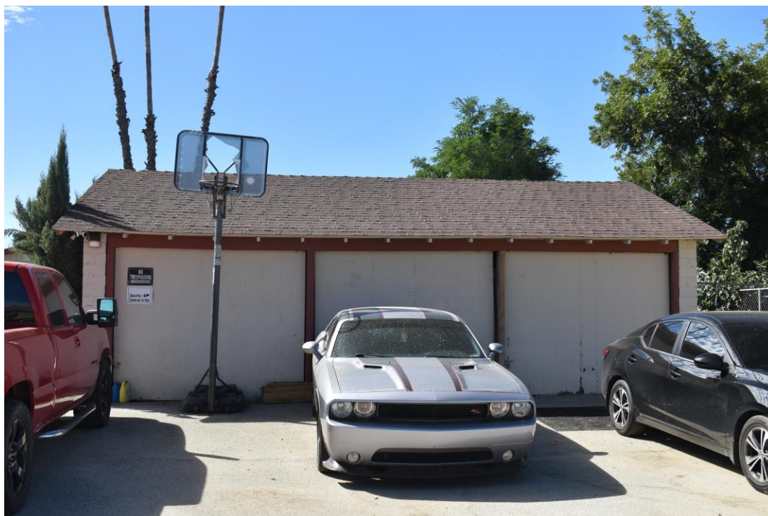
Exhibit 10. Overview of north elevation of Garage 2, facing south.
