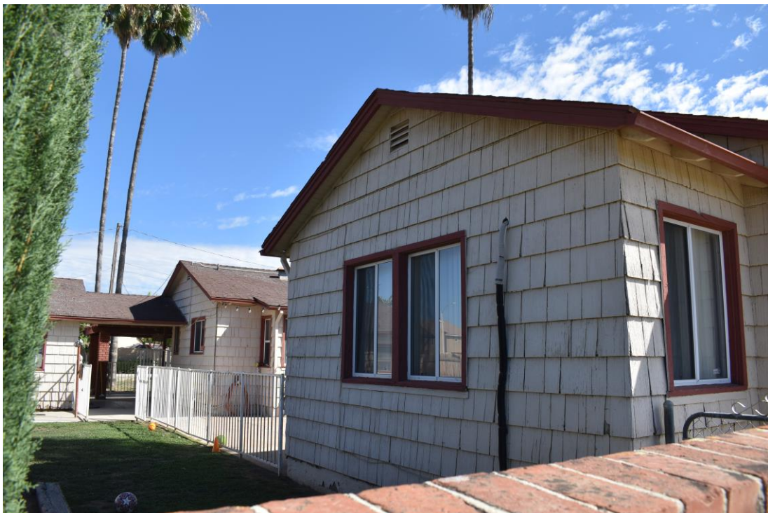
Exhibit 3. Overview of west elevation of Residence 1, facing northeast.
