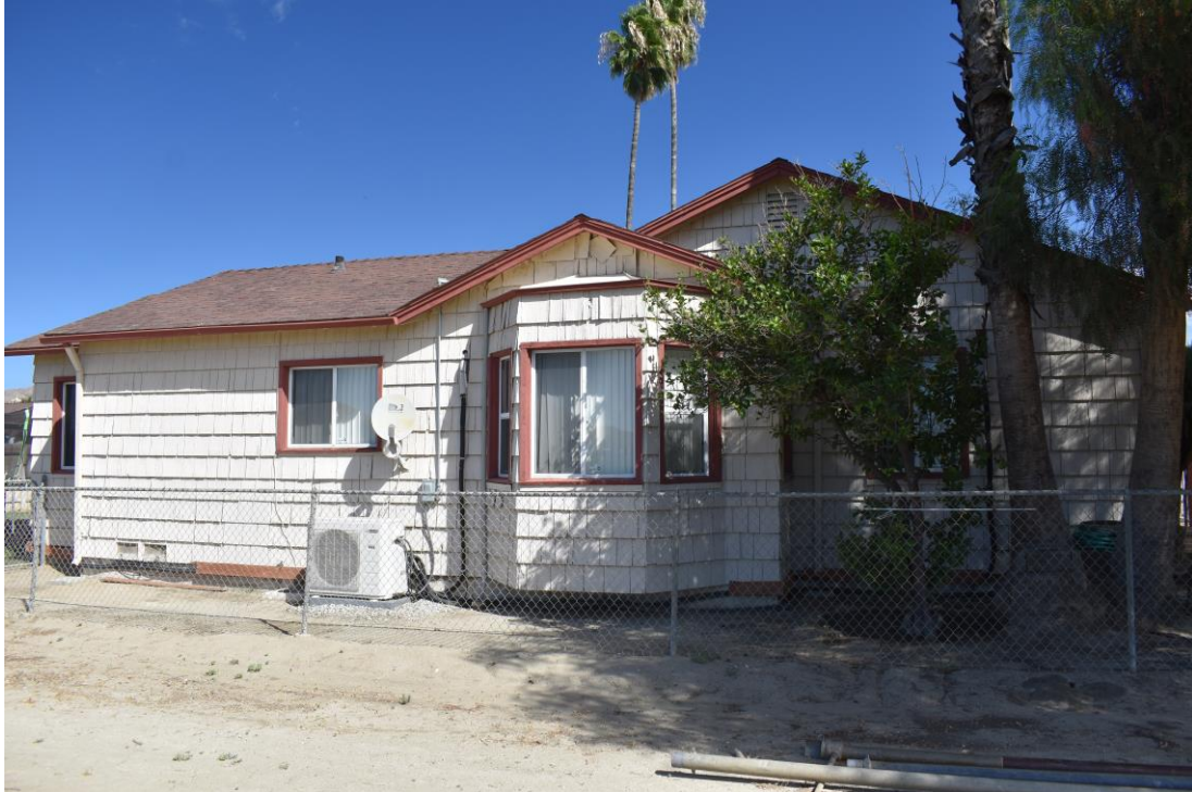
Exhibit 2. Overview of south elevation of Residence 1, facing northwest.
