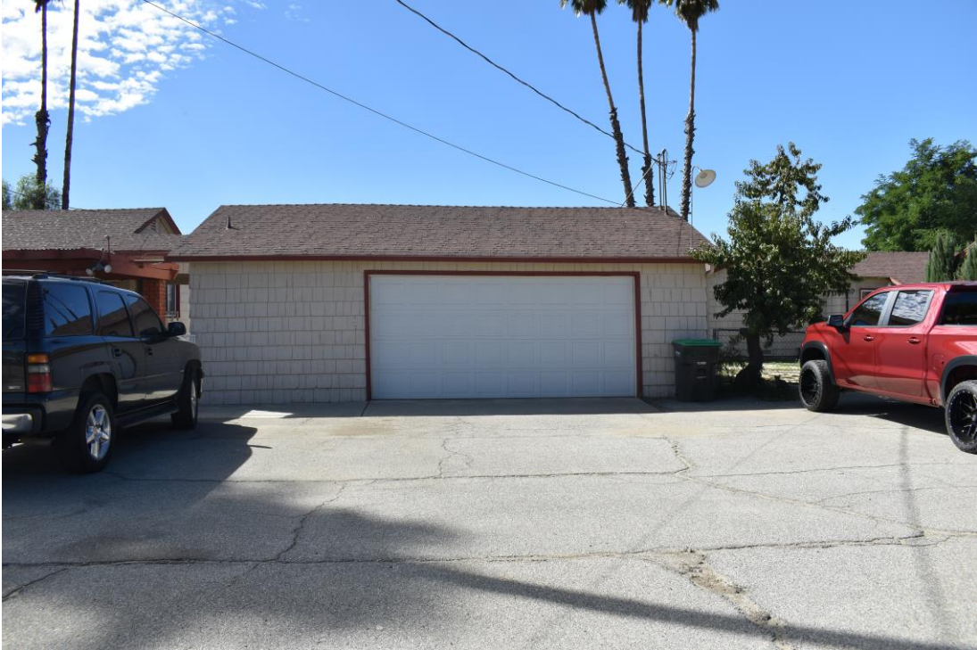
Exhibit 5. Overview of Garage 1 north elevation, facing south.
