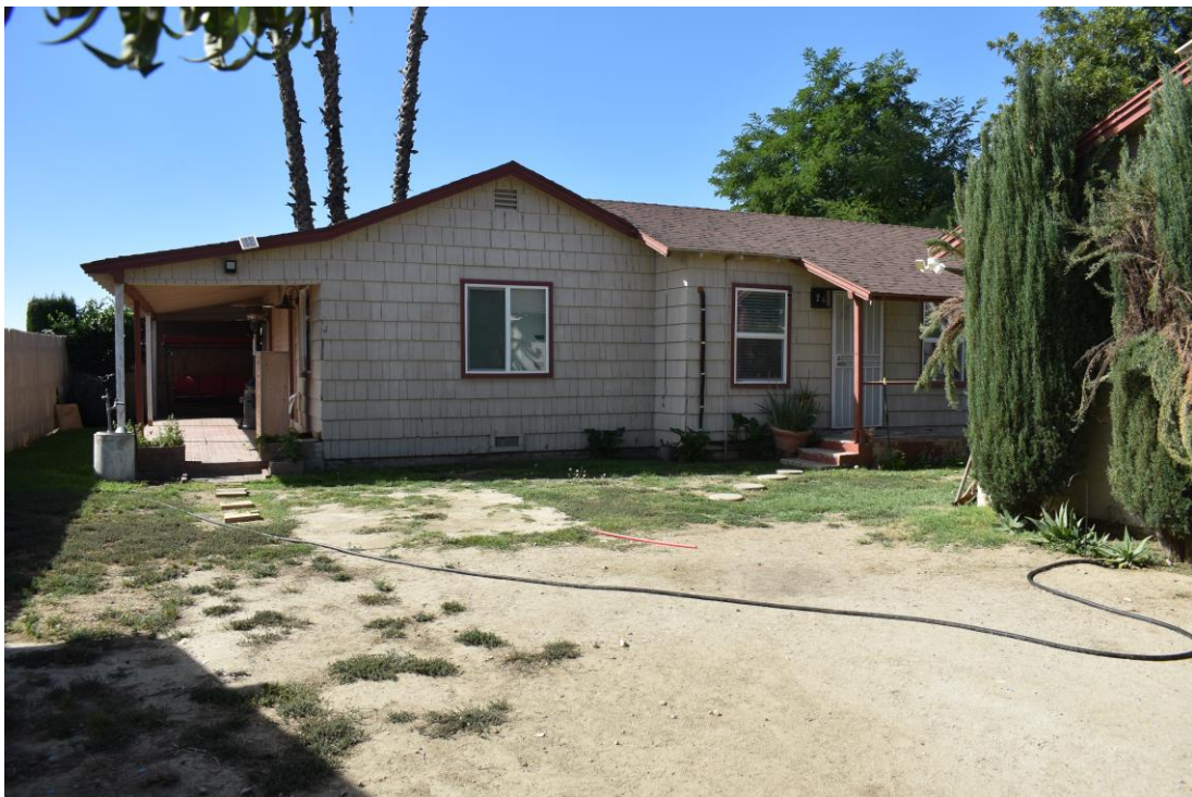
Exhibit 7. Overview of north and east elevations of Residence 2, facing southwest.
