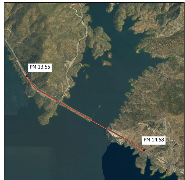
02-2K000 Whiskey Creek Bridge Emergency Repair
