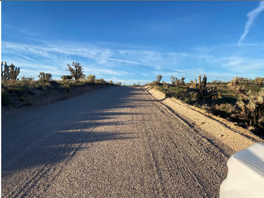
Photo 21: Mile Marker 13 – Looking South
