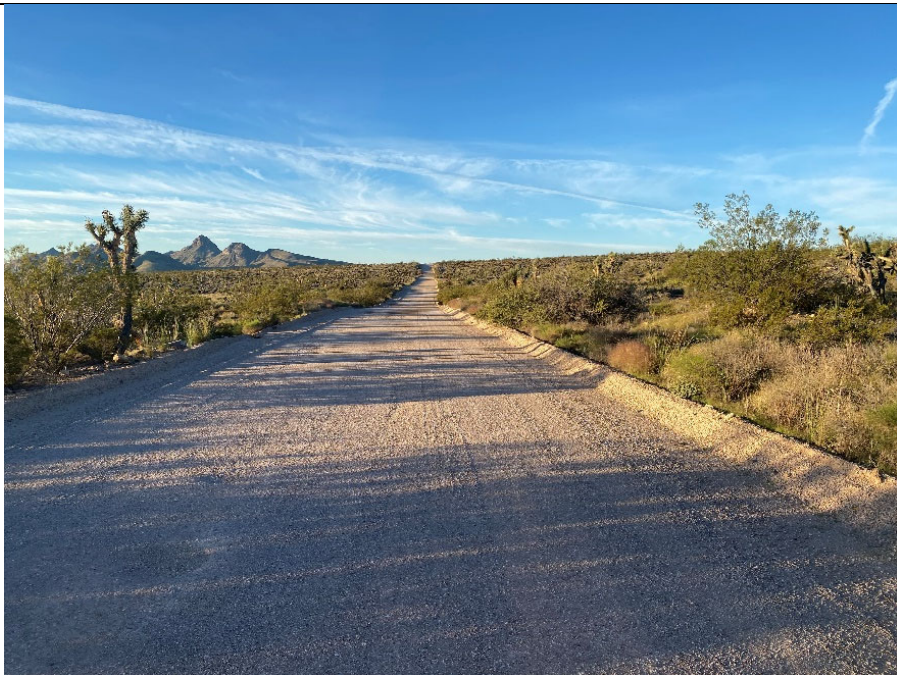
Photo 15: Mile Marker 7 – Looking South
