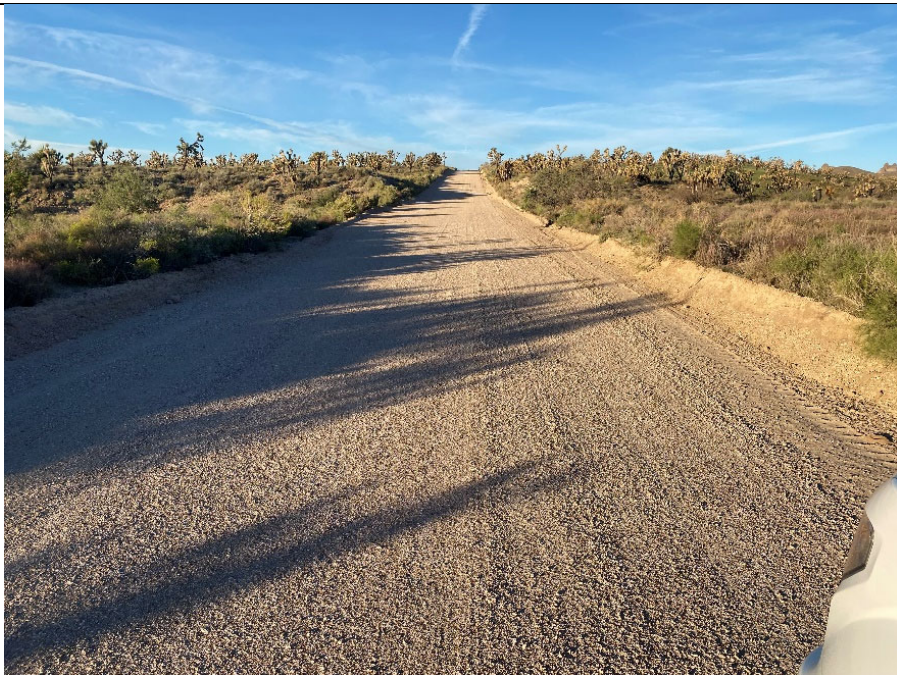
Photo 19: Mile Marker 11 – Looking South
