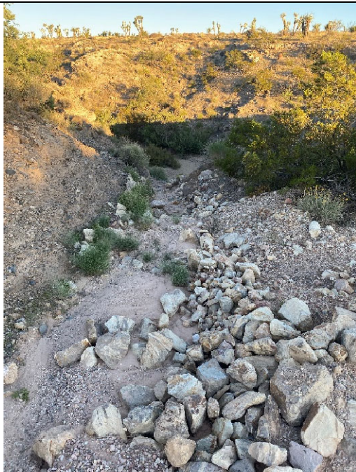
Photo 11: Mile Marker 5 – Looking West, showing drainage
