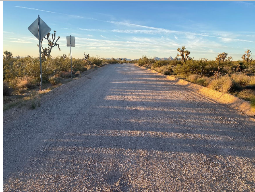
Photo 6: Mile Marker 1 – Looking South
