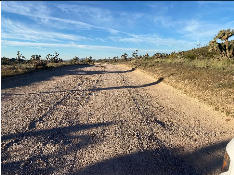
Photo 25: Mile Marker 17 – Looking South
