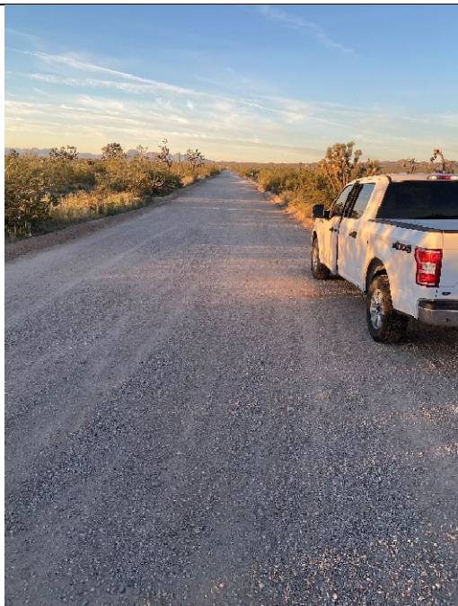
Photo 1: Mile Marker 0 - Looking South
