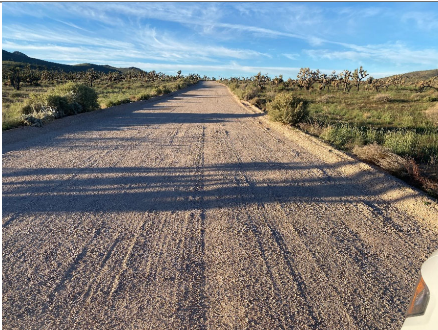
Photo 23: Mile Marker 15 – Looking South
