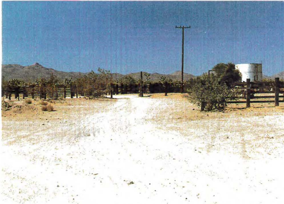
VIEWPOINT 1: South entrance to Walking Box Ranch Headquarters Area. Power line segment "B" would bypass headquarters fenced area and continue south along mine access road.
