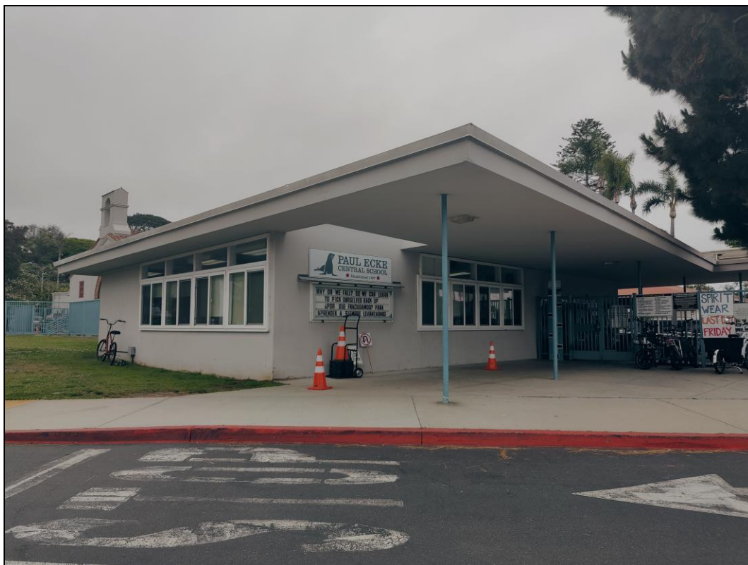
Building #2: north elevation (right) and west elevation (left), facing southeast.
