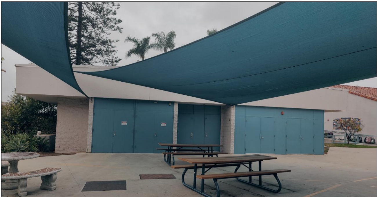
Building #8: east elevation, facing west.
