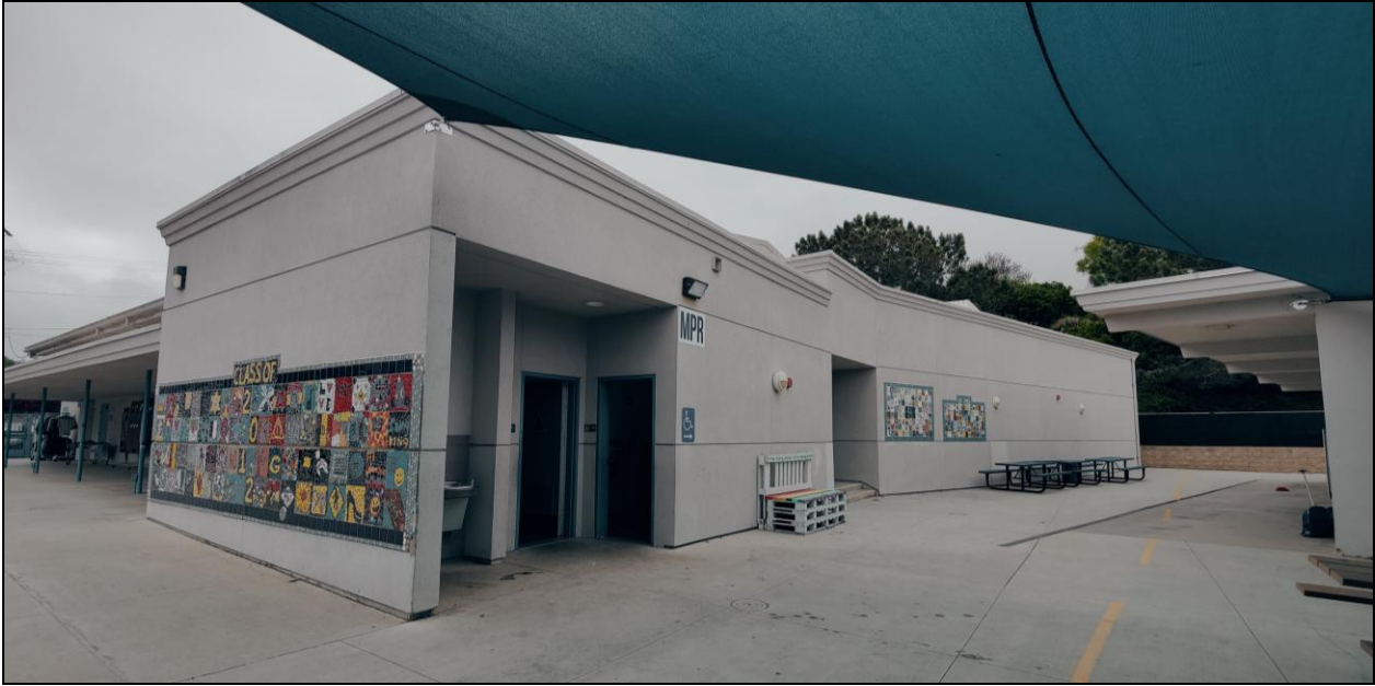
Figure 8. Building #4, south elevation (Multi-Purpose Room), facing northeast.
