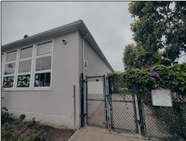
Building #1: western end of north façade (left) and west elevation (right), facing south.
