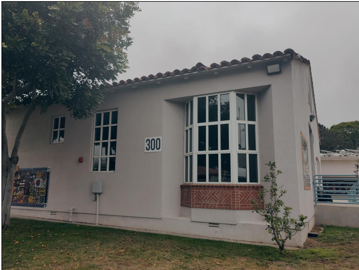
Building #3: southern end of west elevation, facing east.
