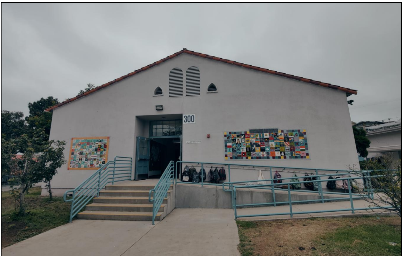
Building #3: south elevation, facing north.
