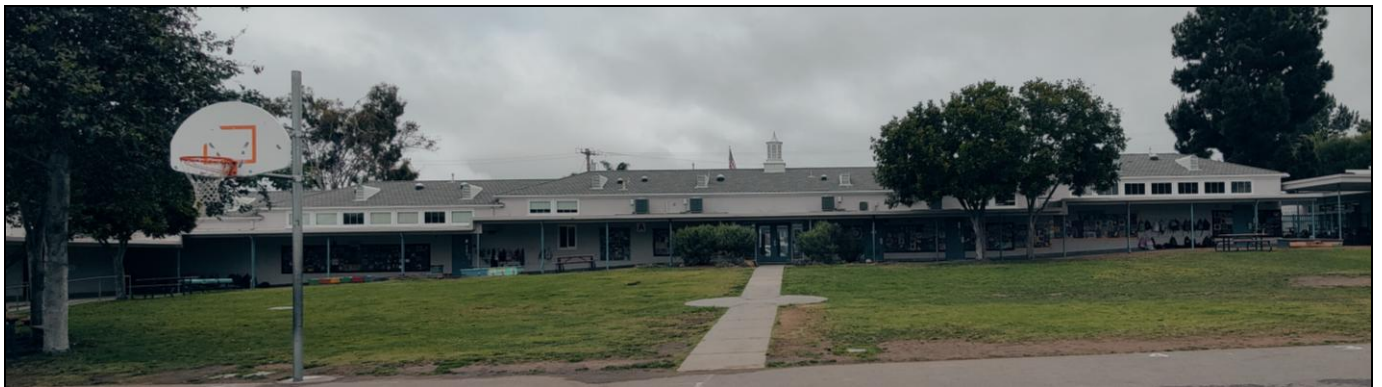
Building #1: south elevation, facing north.
