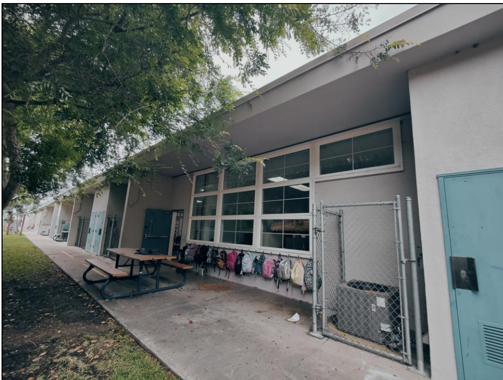
Building #7: overview of south elevation, facing northwest.
