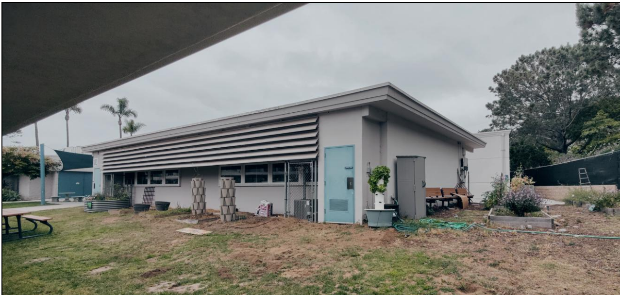
Building #6: south elevation (left) and east elevation (right), facing northwest.
