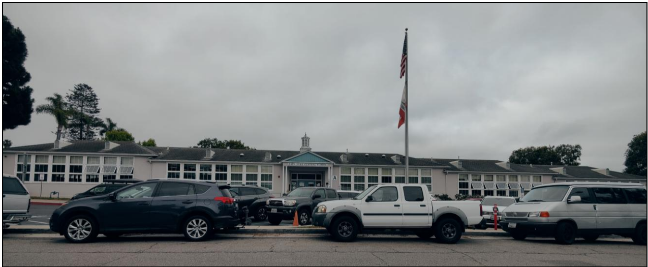
Figure 5. Building 1, north façade, main office and classrooms, facing south.
