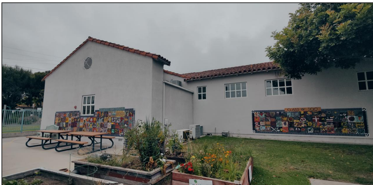
Building #3: northern end of west elevation, facing northeast.
