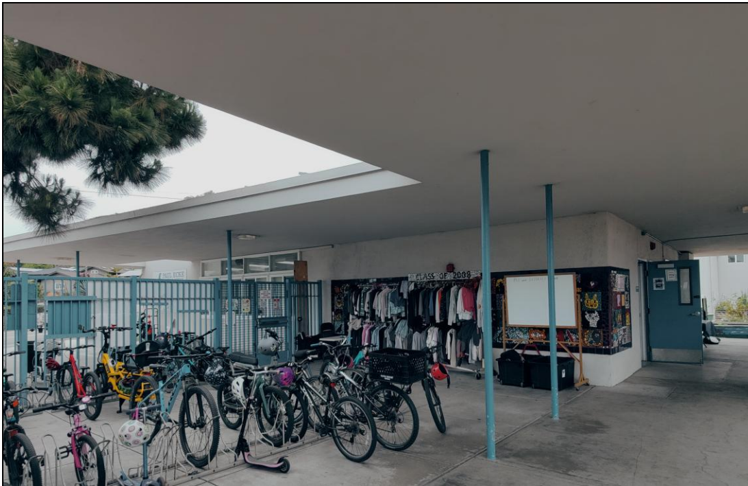
Building #2: west elevation and partial view of south elevation (right), facing northeast.
