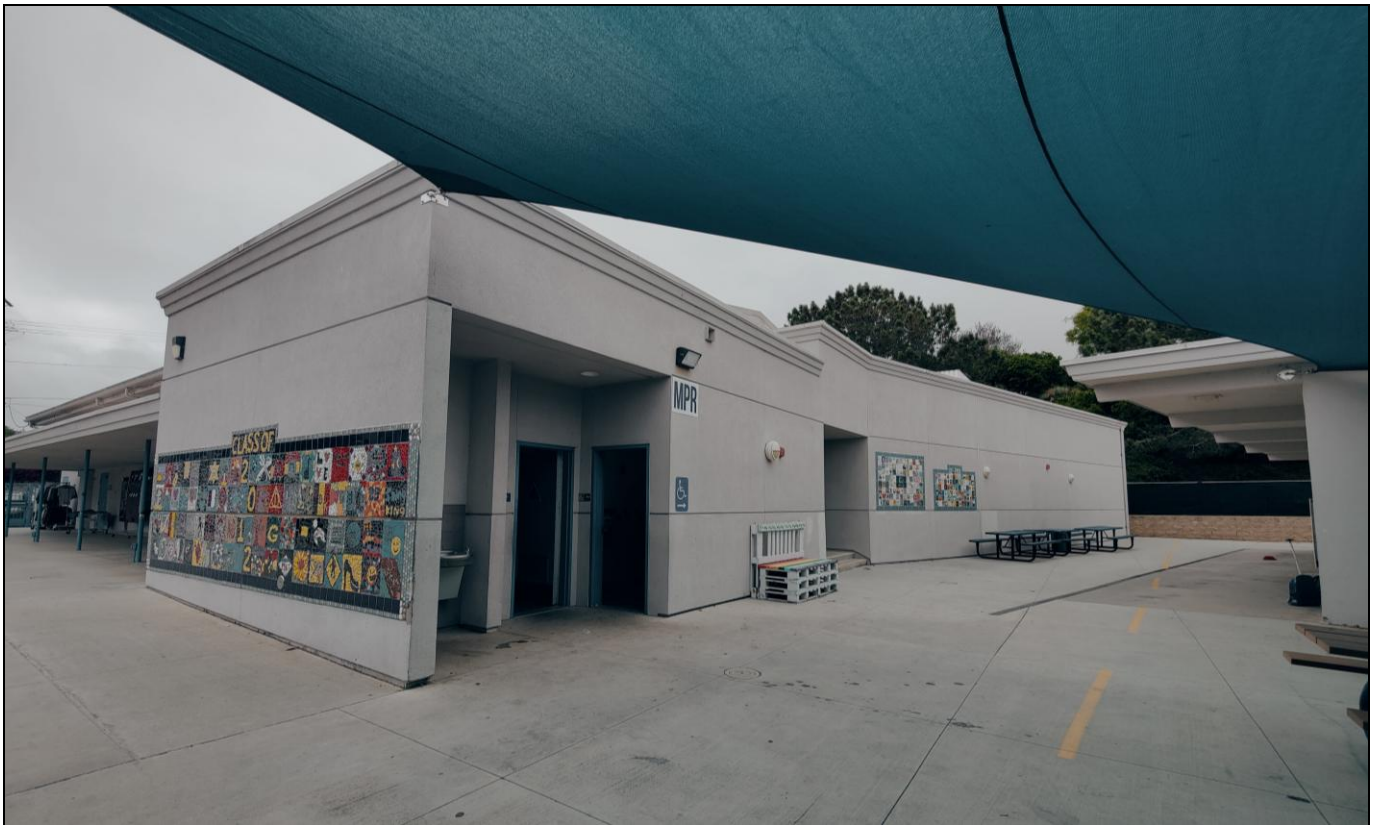
Building #4: south elevation (Multi-Purpose Room), facing northeast.
