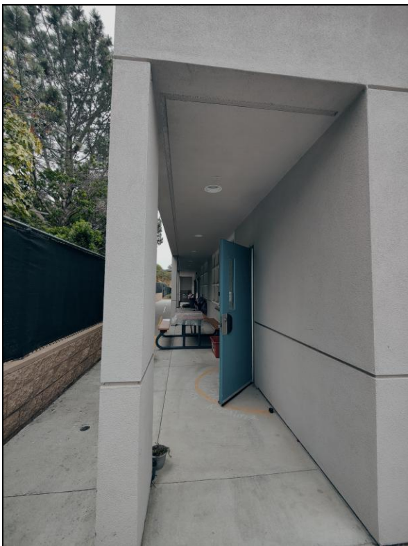
Building #4: east elevation, facing southeast.
