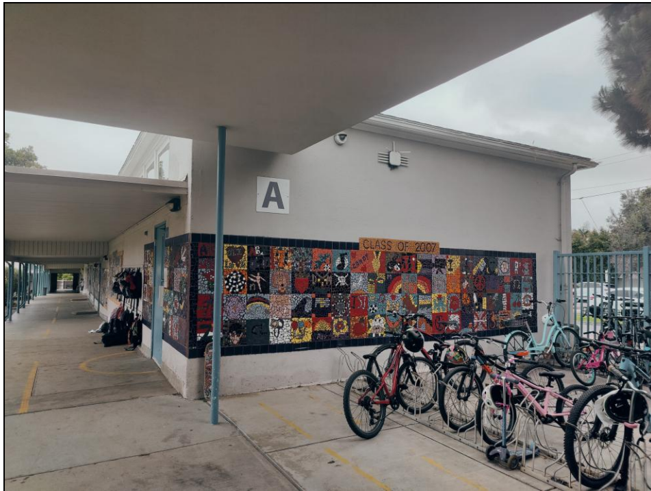
Building #2: east elevation, facing northwest.
