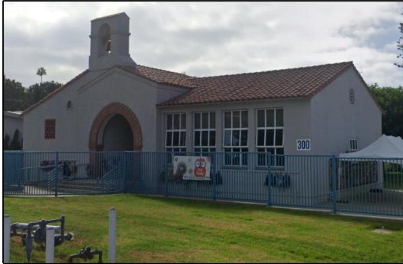
North façade of original school building to remain in place.
