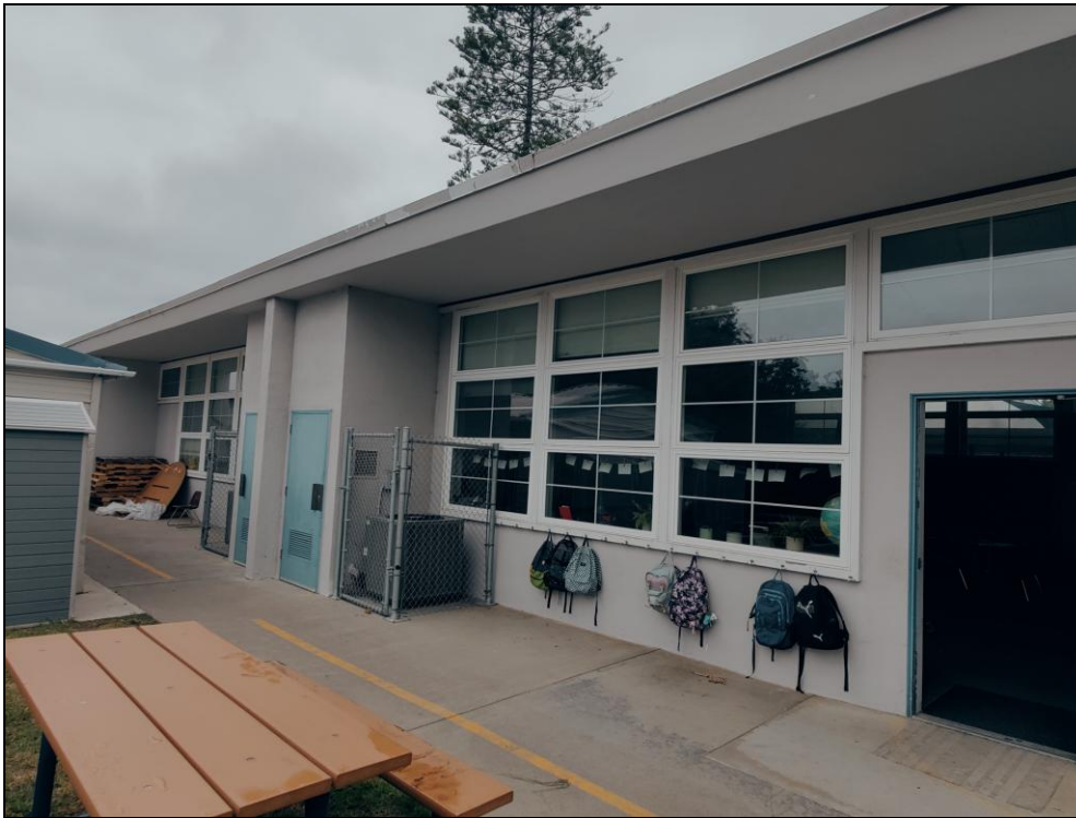
Building #7: western end of south elevation, facing northwest.
