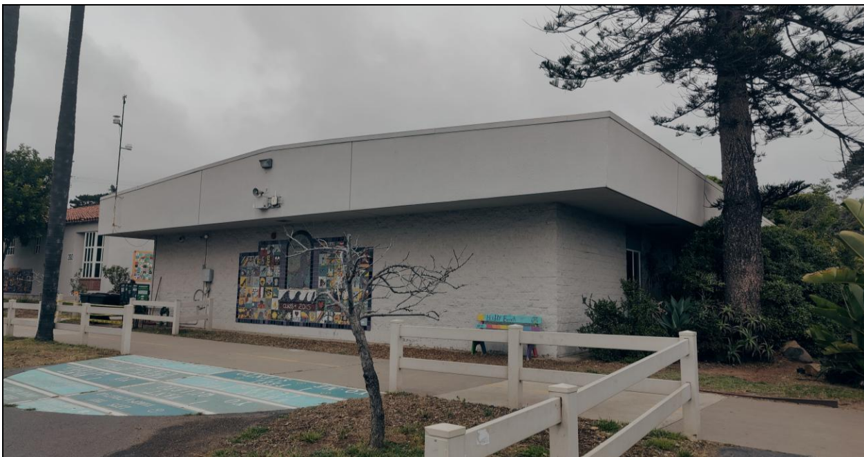
Building #8: west elevation and partial view of south elevation, facing northeast.
