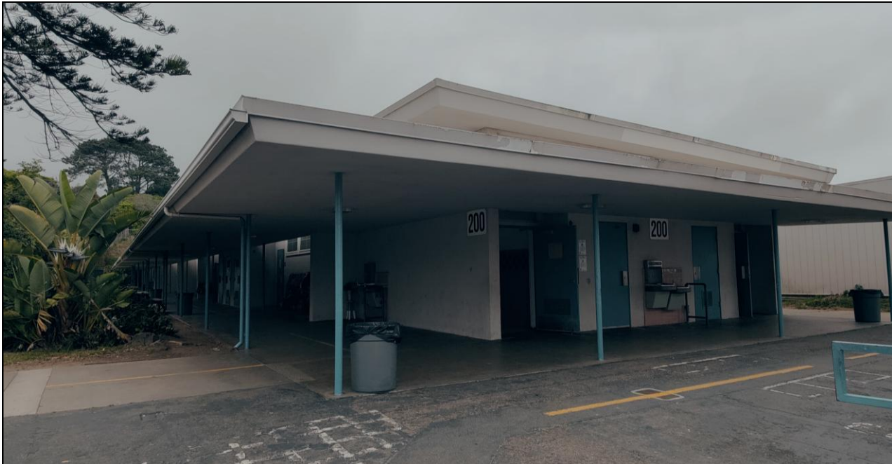
Building #7: north façade (left) and west elevation (right), facing southeast.
