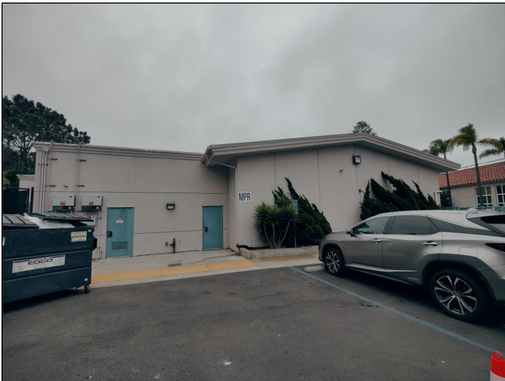
Building #4: northwest elevation, facing southeast.
