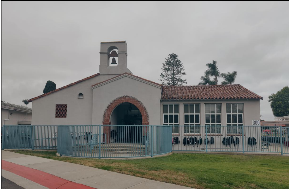
Figure 7. Building #3, north elevation, facing south.
