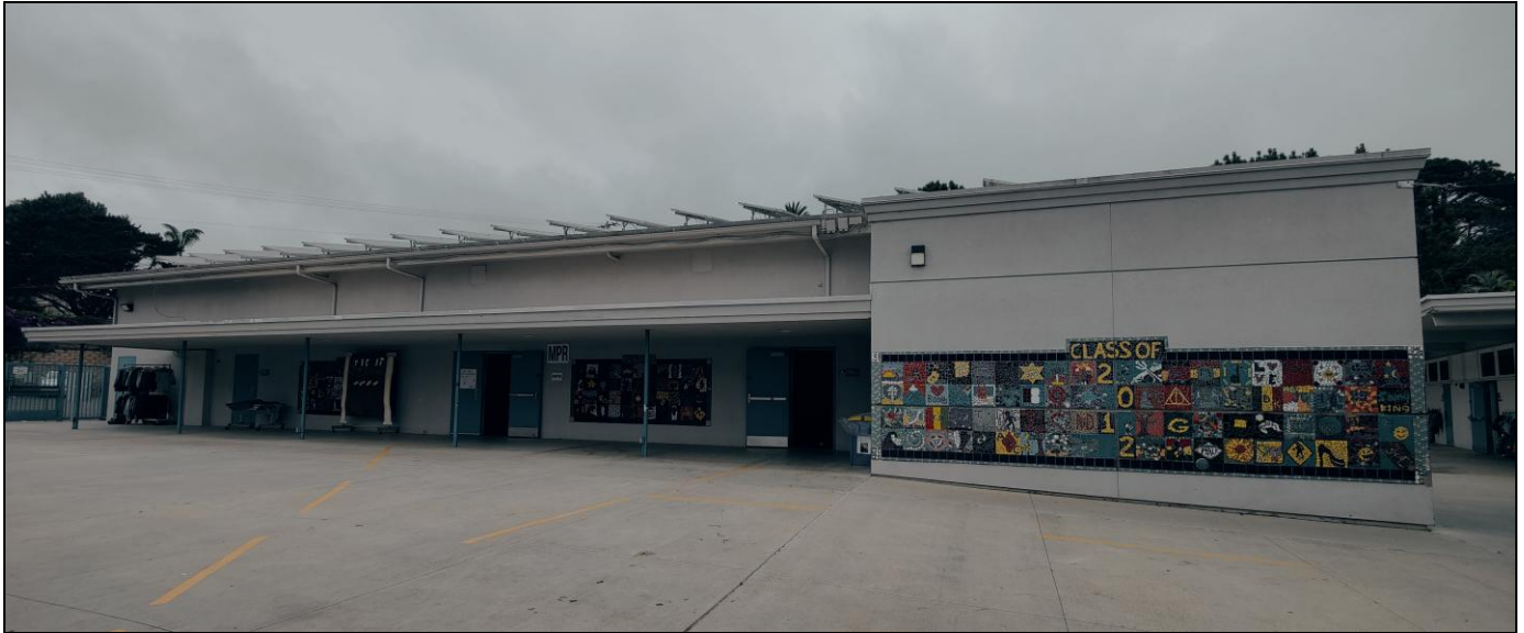
Building #4: southwest elevation (classrooms), facing northeast.
