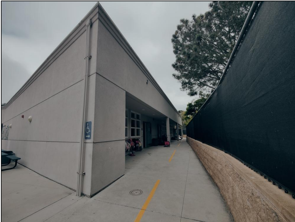
Building #4: south elevation (left) and southern end of east elevation (right), facing northwest.
