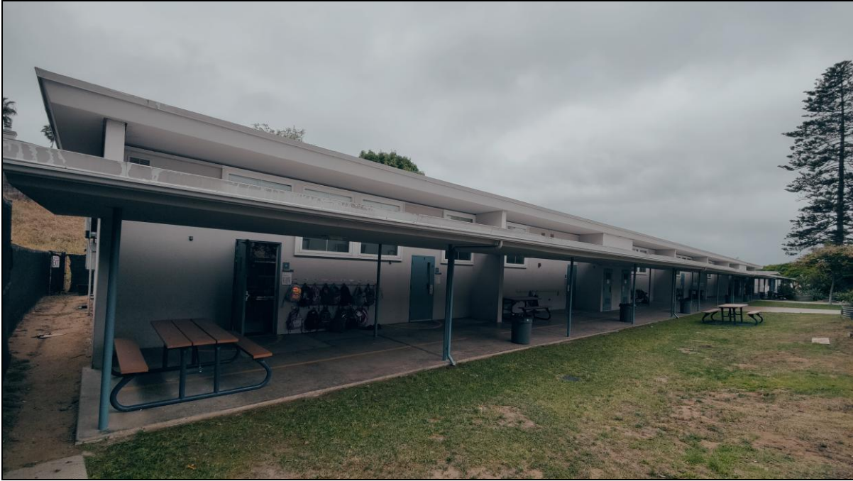
Figure 10. Building #7, north elevation, facing southwest.
