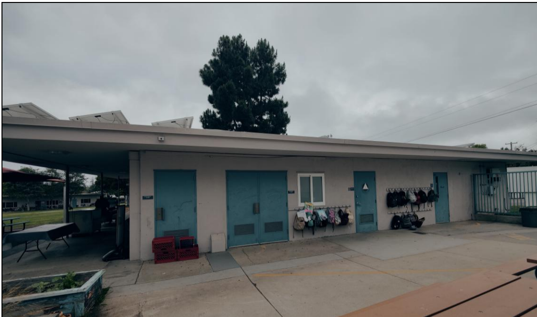
Building #2: east elevation, facing north.
