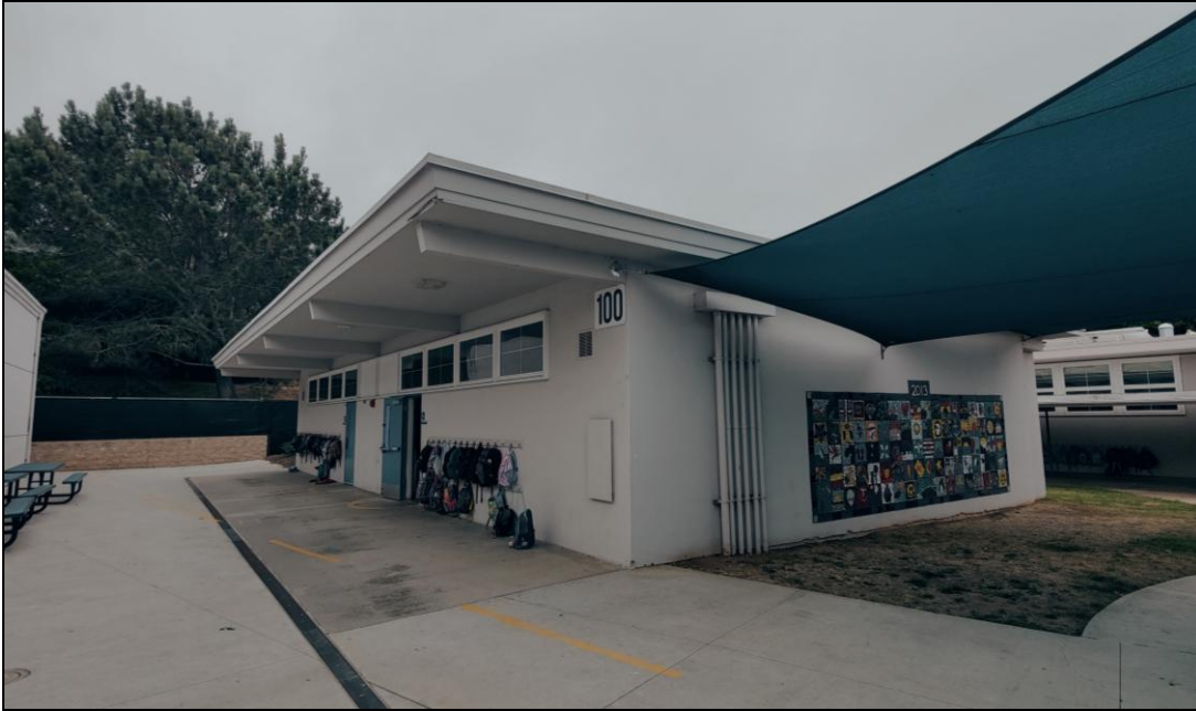
Figure 9. Building #6, north elevation (left) and west elevation (right), facing southeast.
