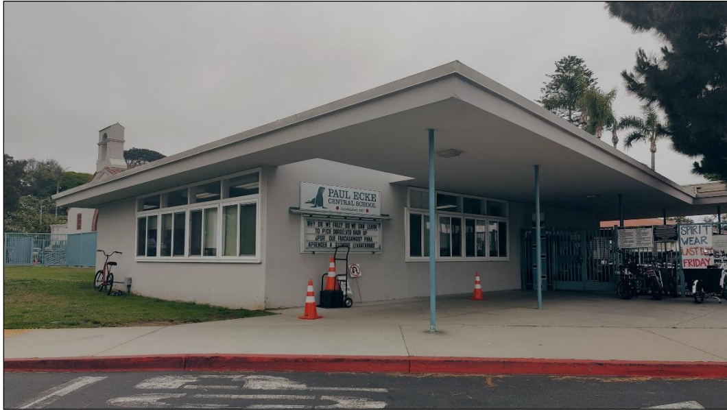
Figure 6. Building #2, north elevation (right) and west elevation (left), facing southeast.
