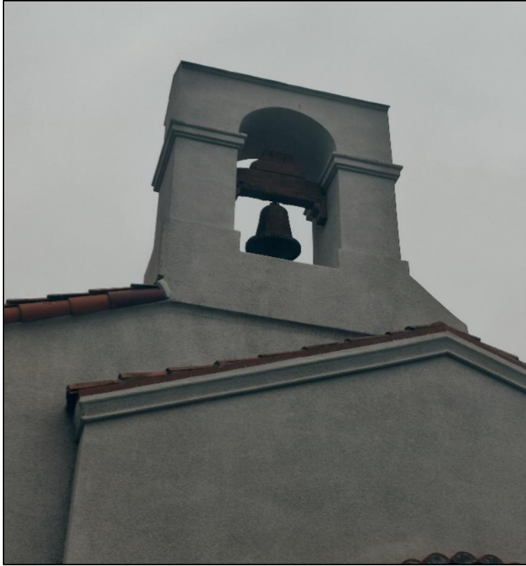
Figure 9. Bell tower at north façade.
