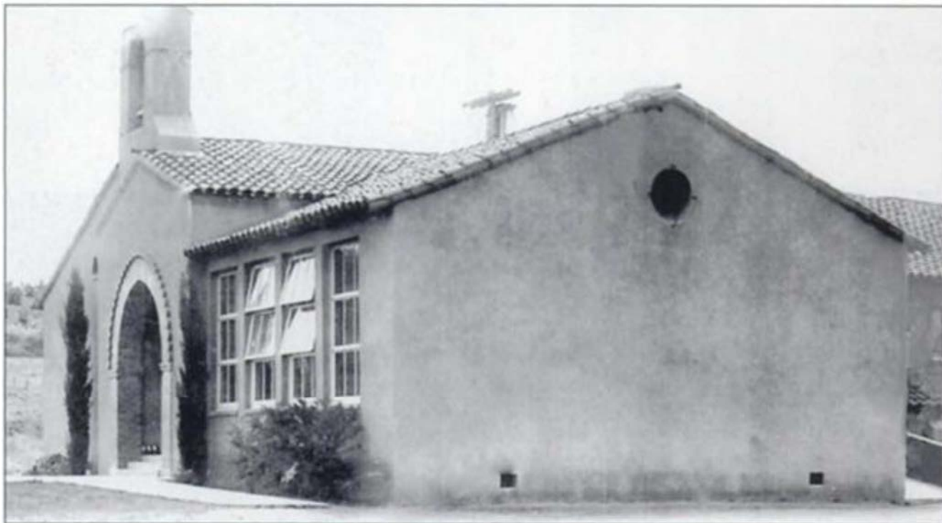
Figure 4. Building #3, 1932 photograph of north façade (left) and west elevation (right) (Holtzclaw 2006).
