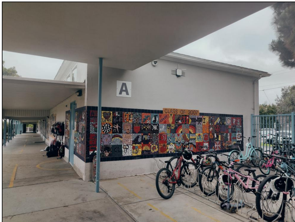
Building #2: east elevation, facing northwest.
