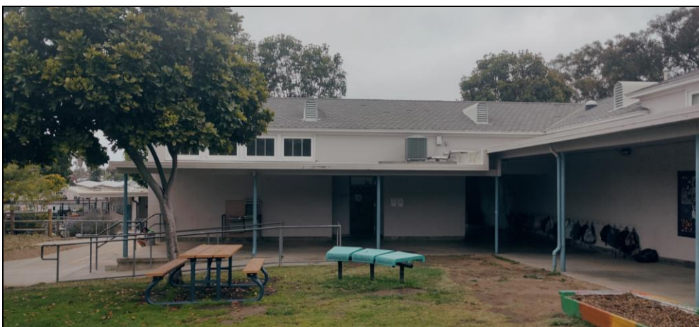
Building #1: western end of building, east elevation, facing west.
