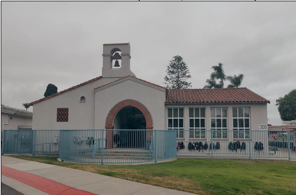
Building #3: north elevation, facing south.
