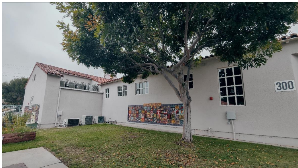
Figure 14. Overview of west elevation, facing northeast.
