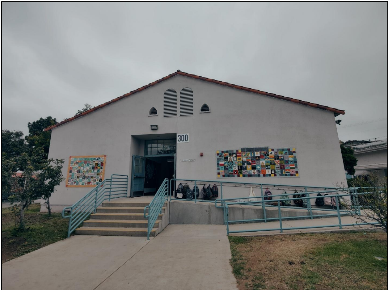
Figure 12. South elevation, facing north.
