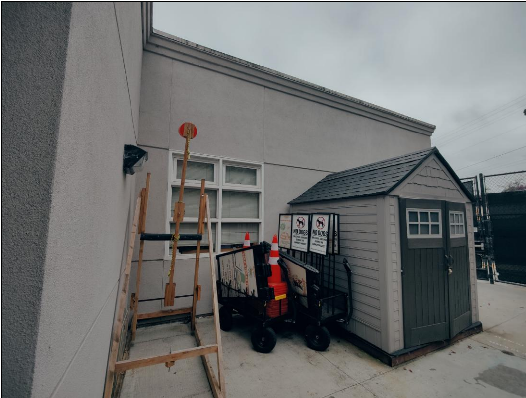
Building #4: northern end of east elevation, facing west.
