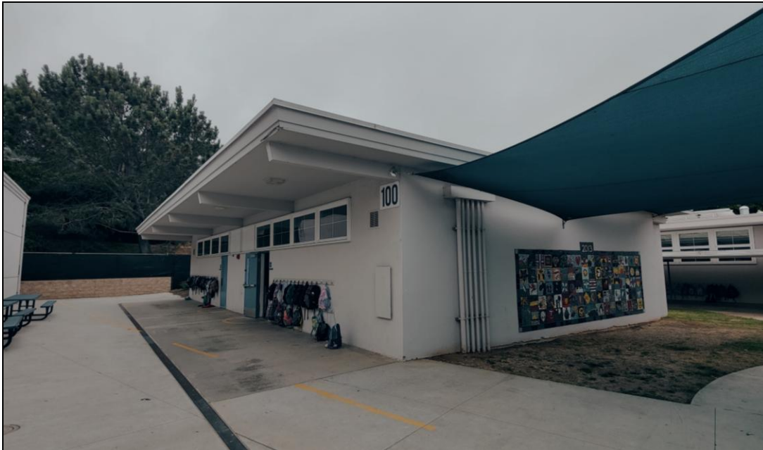
Building #6: north elevation (left) and west elevation (right), facing southeast.
