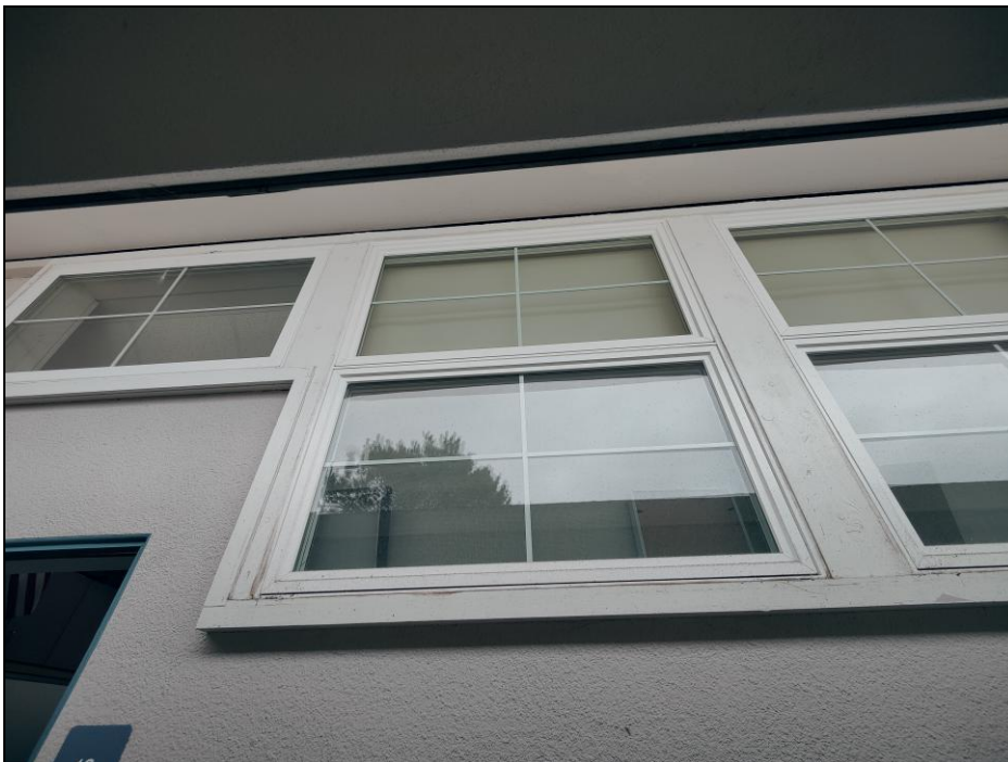
Building #7: close up of fixed windows at eave levels at north façade.
