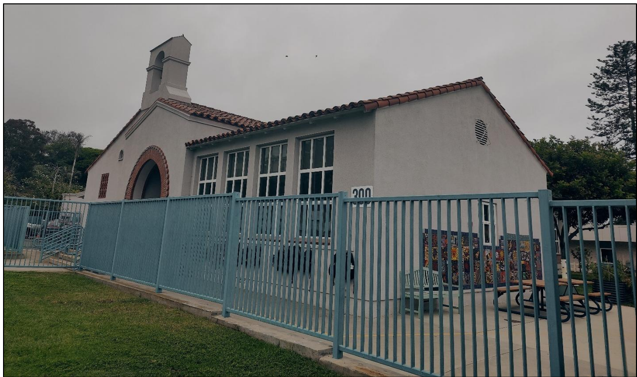
Figure 8. Building #3, north façade (left) and partial view of west elevation, facing southeast
