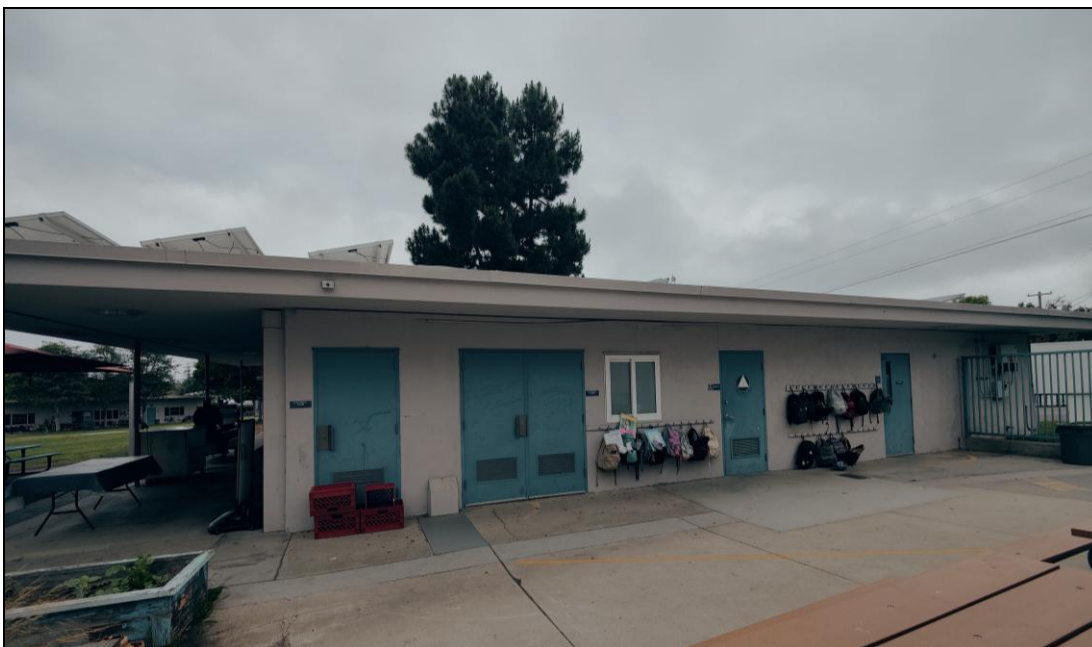
Building #2: east elevation, facing north.
