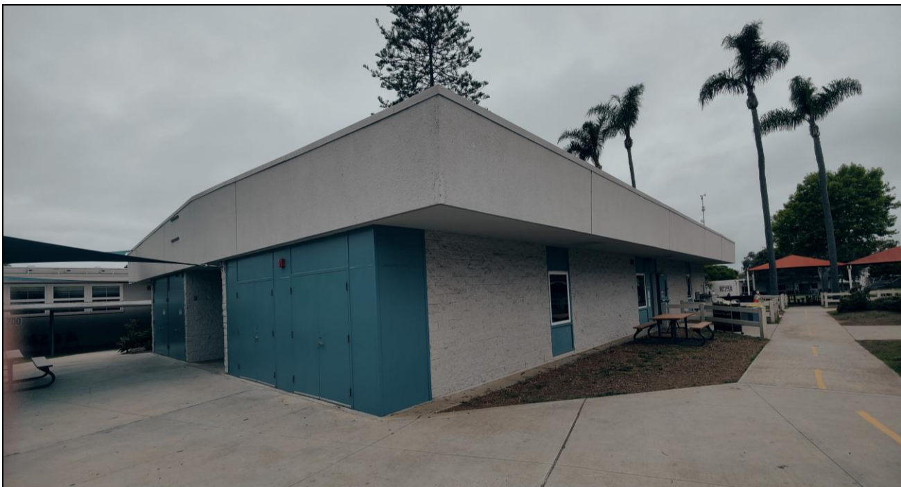
Building #8: east elevation (left) and north façade (right), facing southwest.
