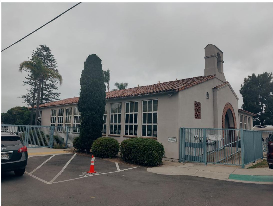
Building #3: east elevation (left) and north façade (right), facing southwest.
