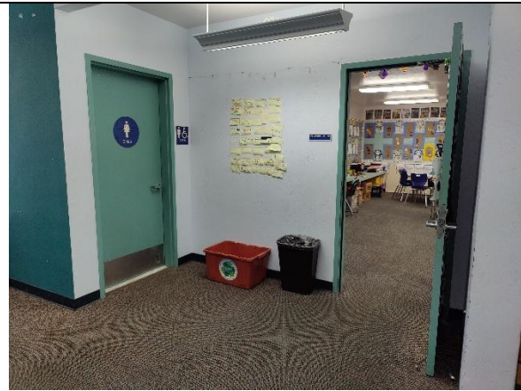
Girls restroom and Classroom 23 at north end of building.
