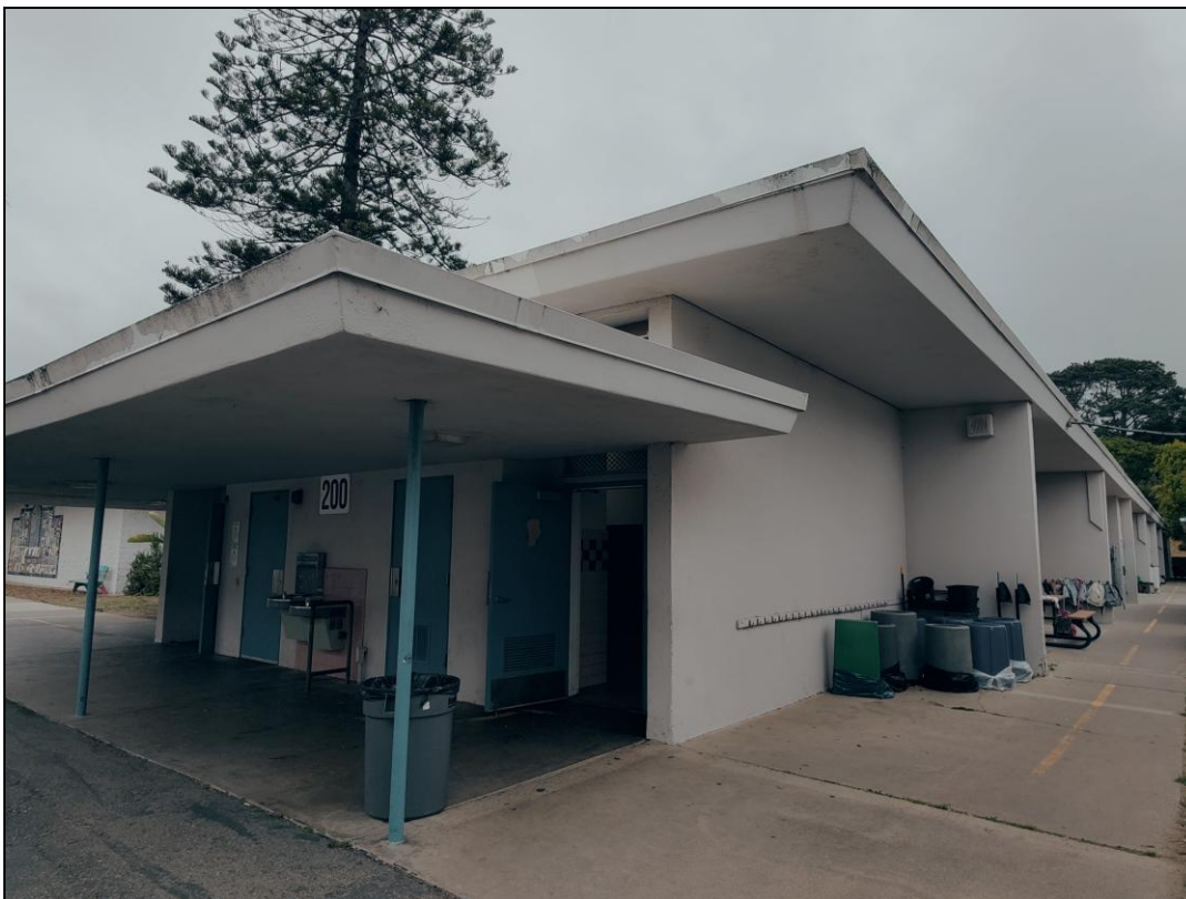
Building #7: west elevation (left) and western end of south elevation (right), facing northeast.
