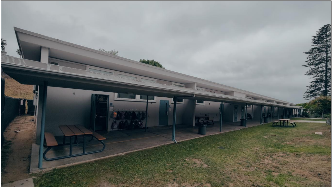
Building #7: north elevation, facing southwest.
