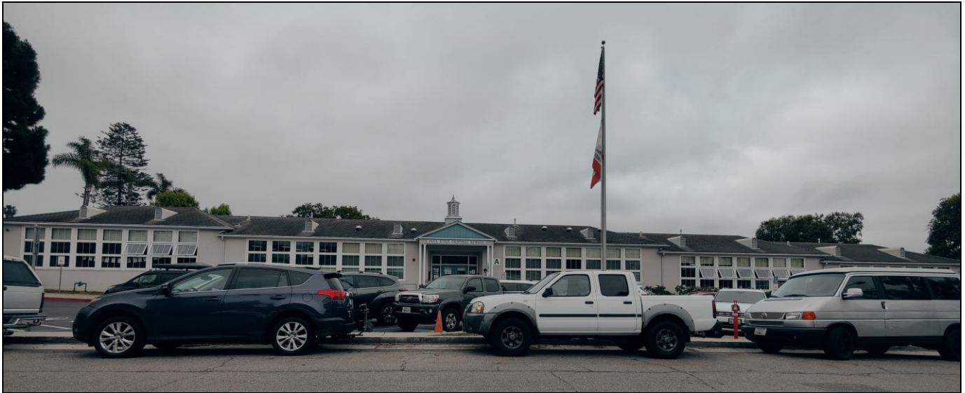
Building #1: North façade, main office and classrooms, facing south.
