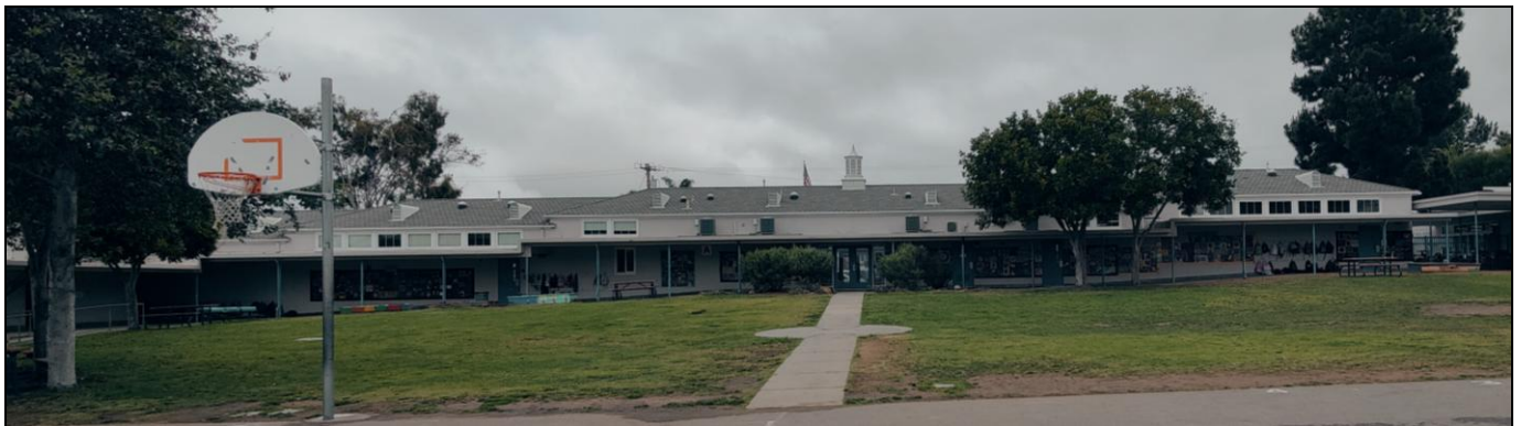
Building #1: south elevation, facing north.
