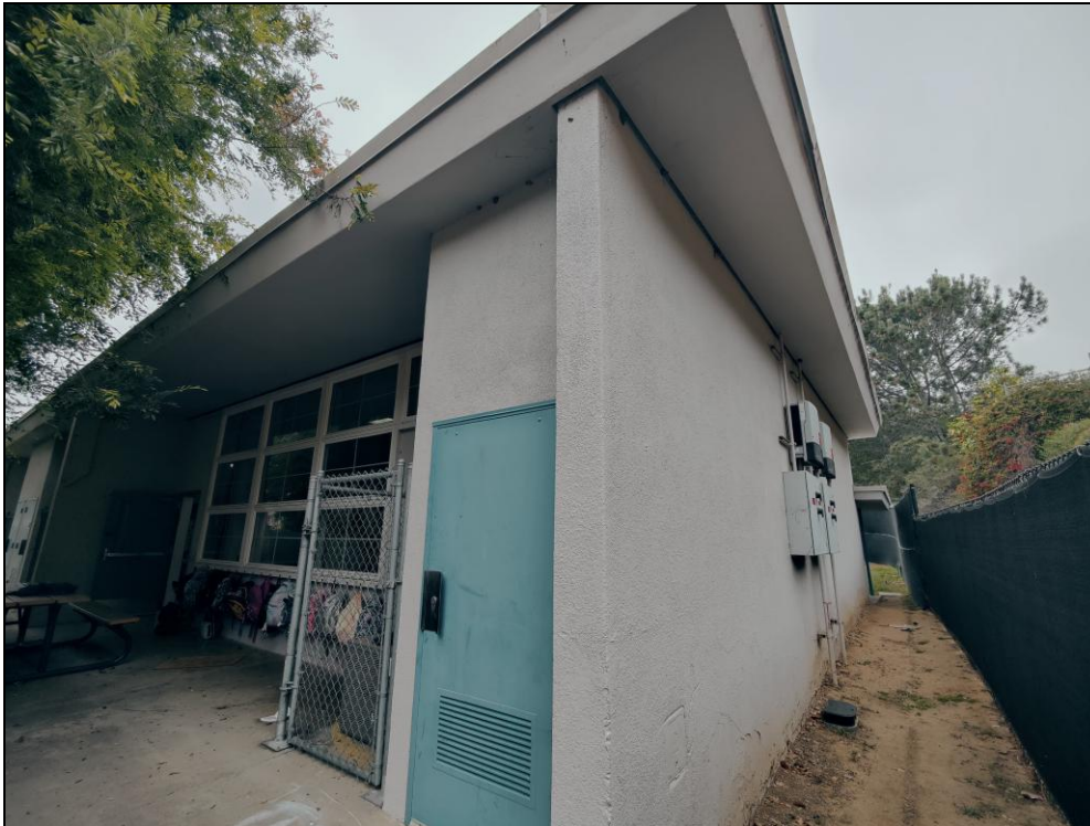
Building #7: eastern end of south elevation (left) and east elevation (right), facing northwest.
