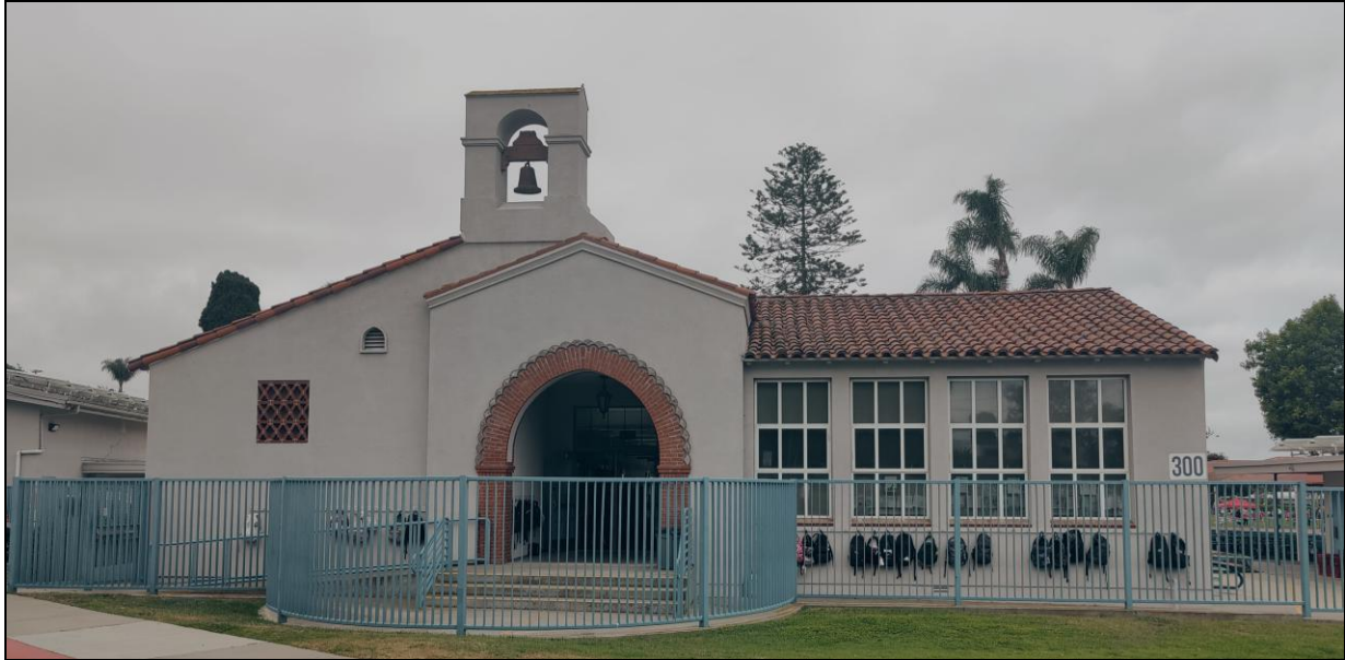
Figure 7. Building #3, north elevation, facing south.
