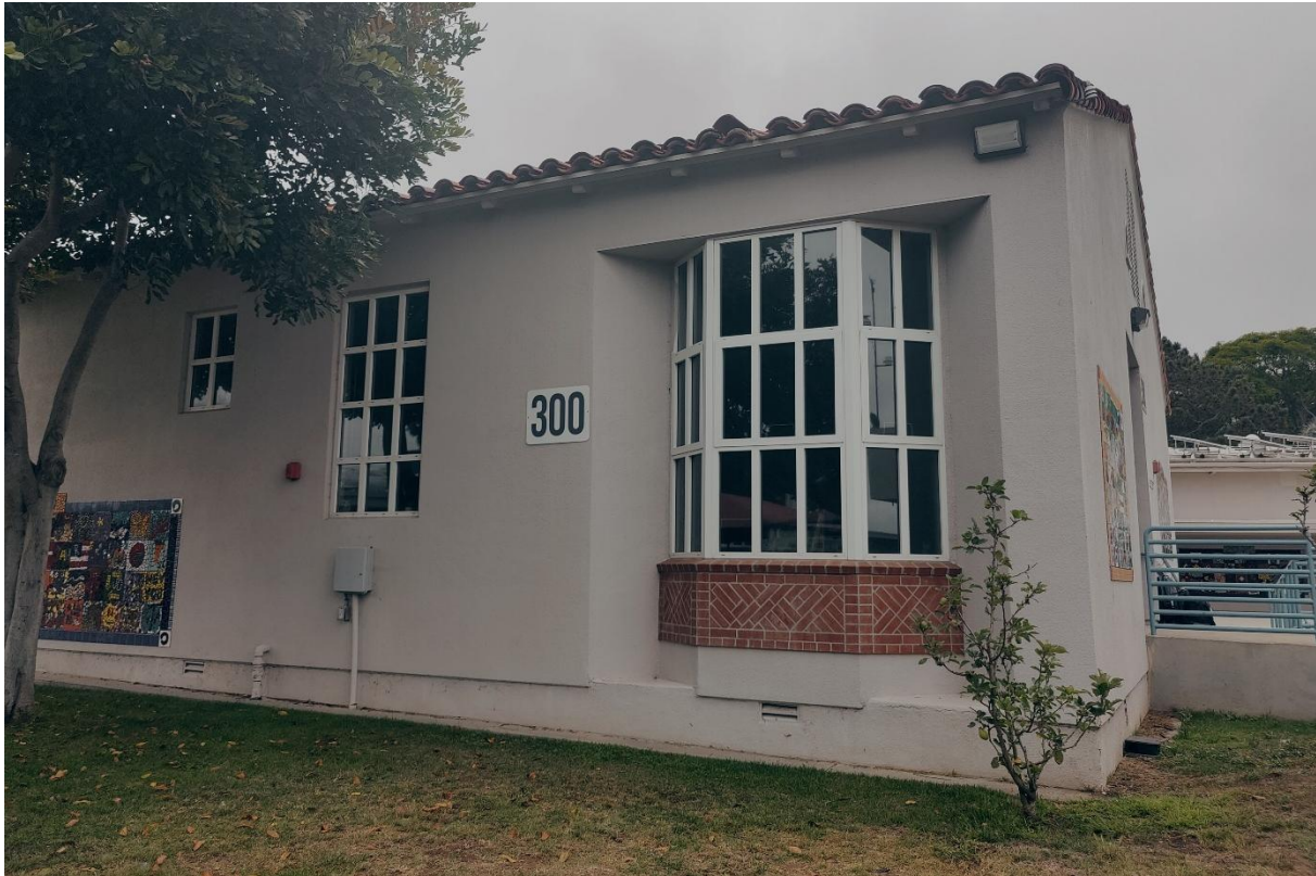
Figure 13. Canted window and decorative brick apron at southern end of west elevation, facing east.
