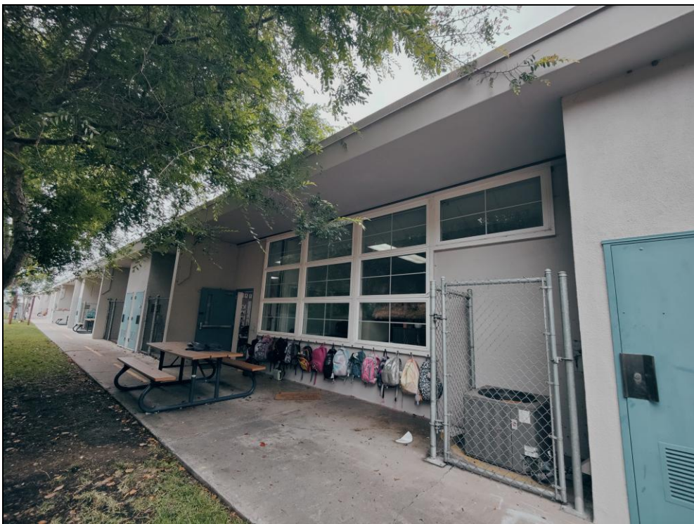
Building #7: overview of south elevation, facing northwest.
