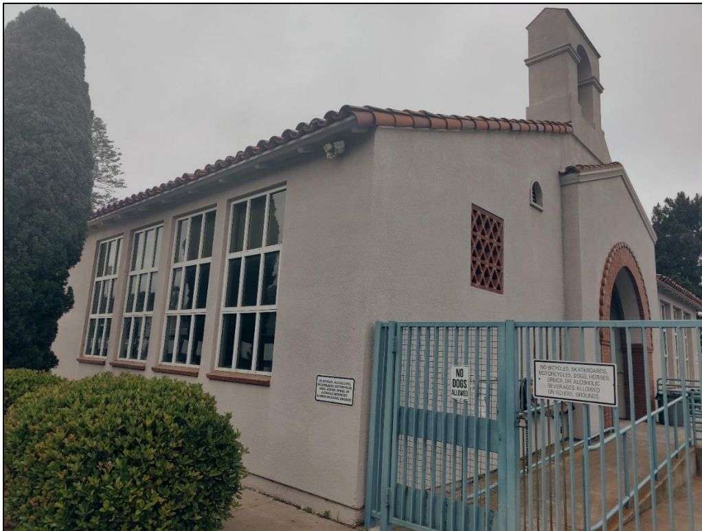
Figure 10. Partial view of east elevation (left) and north façade (right), facing southwest
