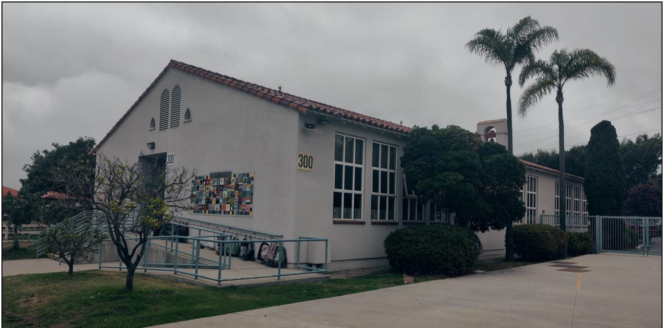
Building #3: south elevation (left) and east elevation (right), facing northwest.
