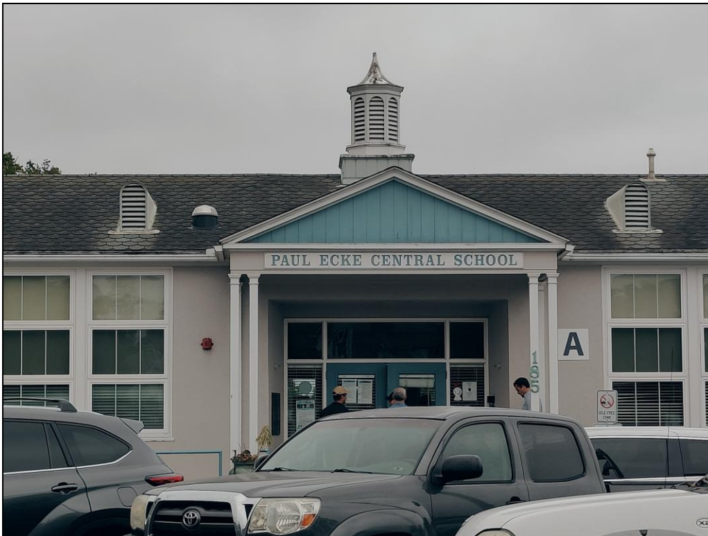
Building #1: Close up of main entrance, main office and classrooms, facing south.
