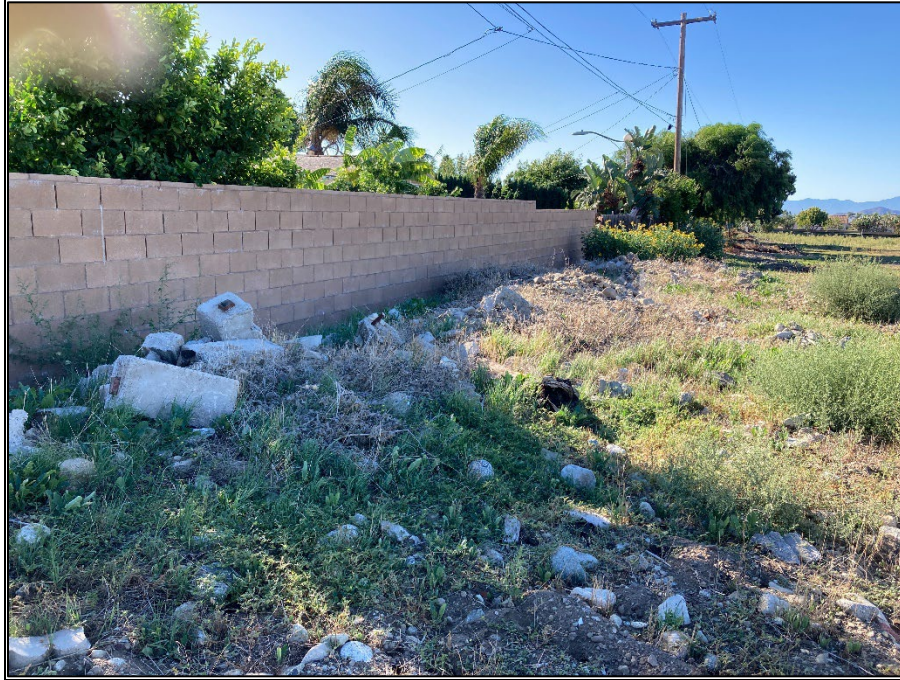
Photo 9. Trash and debris present along the eastern perimeter of the Project site, facing southeast.
