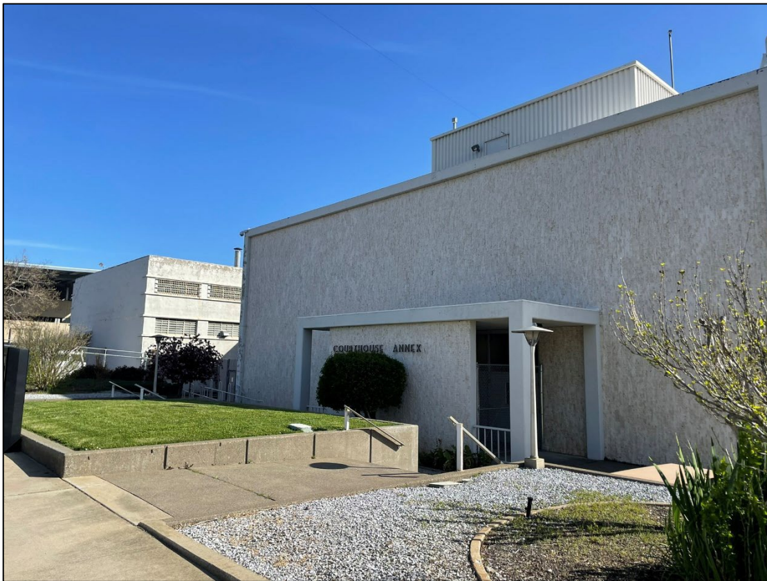
Photo 4. Viewing north along the existing courthouse building frontage.
