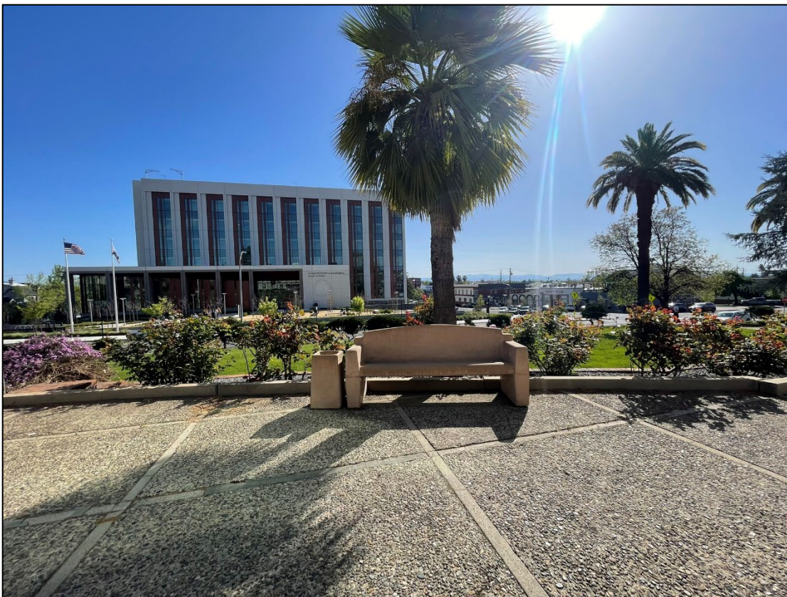
Photo 7. Viewing east toward Court Street from the front of the existing courthouse building.
