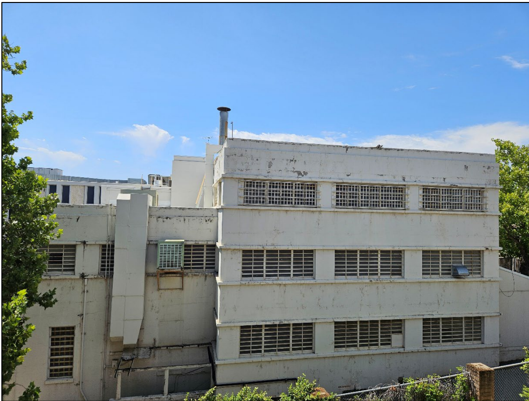
Photo 5. Viewing south toward the existing jail building from the adjacent parking garage.
