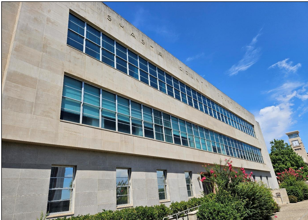
Photo 2. Viewing north along the existing courthouse building frontage.
