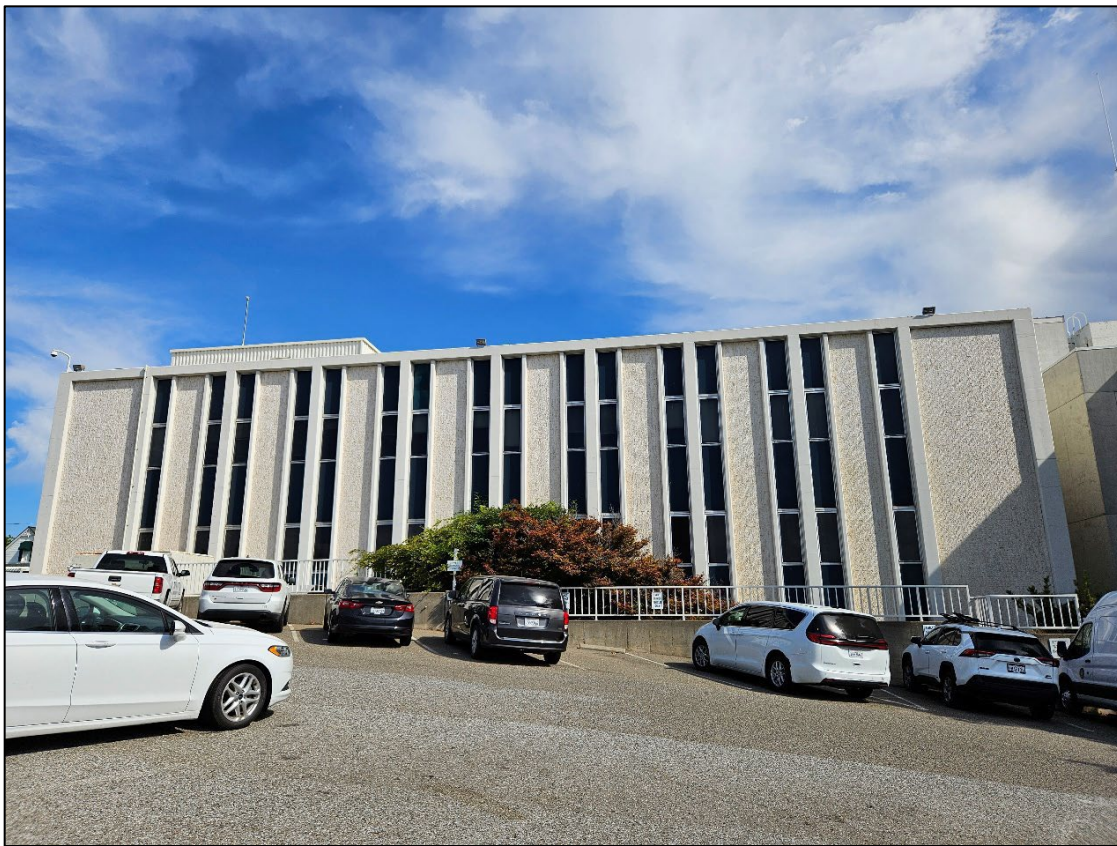
Photo 3. Viewing north toward the existing annex building from the parking lot.
