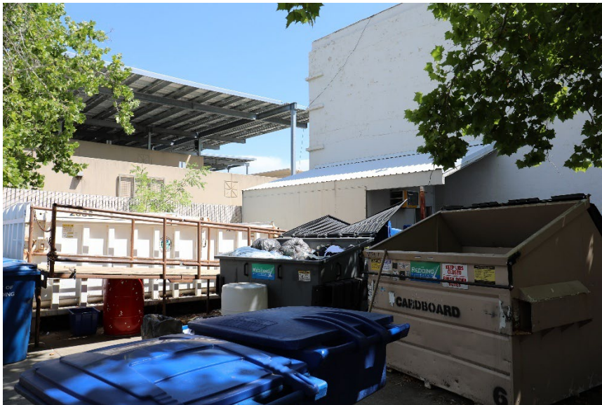
FIGURE 86 VIEW OF THE NORTHERN ENCLOSURE AREA AND THE LEAN-TO SHED, LOOKING NORTHEAST. (MIG 2025)
