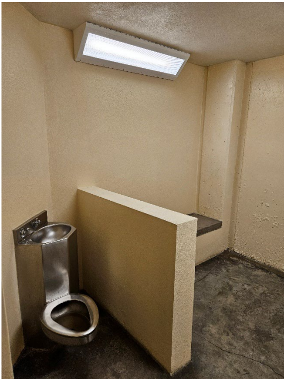
FIGURE 78 A TYPICAL INMATE HOLDING CELL IN THE SALLYPORT STRUCTURE. (MIG 2025)
