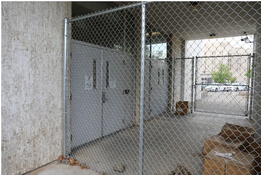
FIGURE 65 VIEW OF THE ENTRANCE DOORS TO THE COURTHOUSE ANNEX UNDER THE COVERED ENTRYWAY, LOOKING SOUTH-SOUTHEAST. (MIG 2025)
