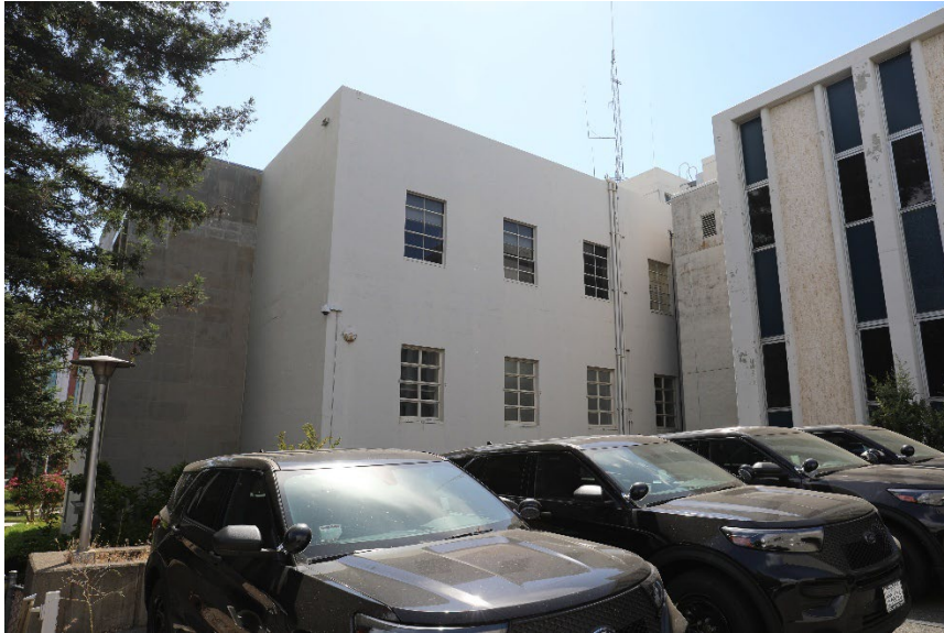
FIGURE 46 VIEW OF THE WEST ELEVATION OF THE MAIN COURTHOUSE, NORTH OF THE CONNECTING CORRIDOR, LOOKING EAST-SOUTHEAST. (MIG 2025)
