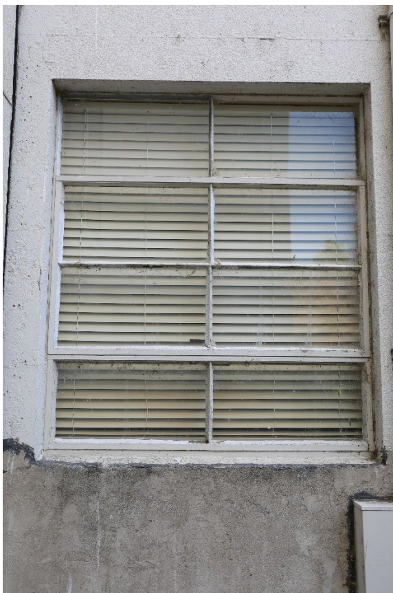
FIGURE 47 CLOSE-UP VIEW OF THE ALUMINUM WINDOW FOUND ON THE WEST ELEVATION OF THE MAIN COURTHOUSE. LOOKING EAST. (MIG 2025)
