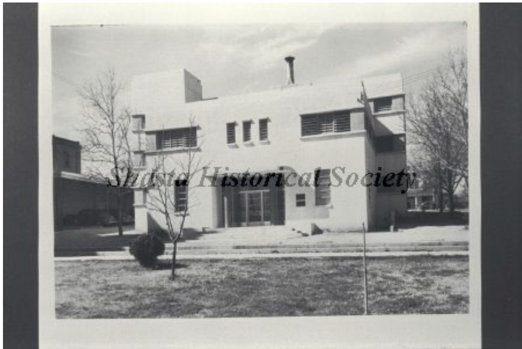
FIGURE 20 VIEW OF THE 1939 SHASTA COUNTY JAIL, LOOKING SOUTHWEST. C.1939-1967. ("SHASTA COUNTY JAIL," SHASTA HISTORICAL SOCIETY, CAT # 1978.58.52)
