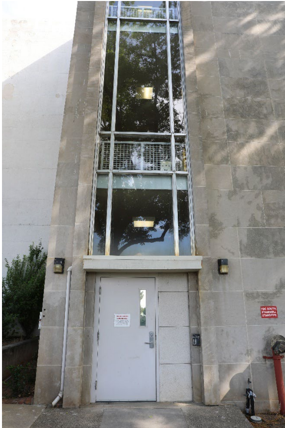
FIGURE 43 VIEW OF THE METAL DOOR AND GLAZING SYSTEM ON THE SOUTH ELEVATION, LOOKING NORTH. (MIG 2025)
