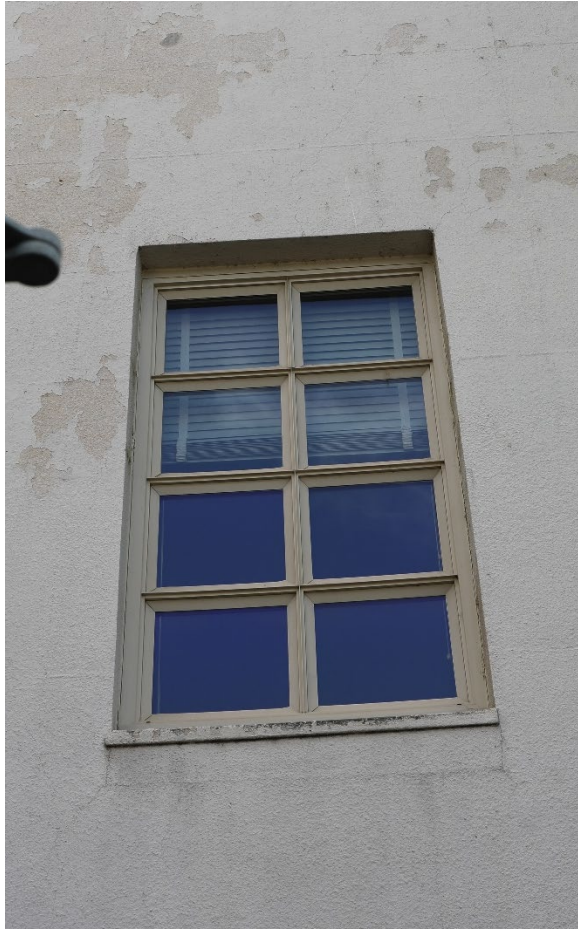
FIGURE 48 CLOSE-UP VIEW OF THE VINYL WINDOW FOUND ON THE WEST ELEVATION OF THE MAIN COURTHOUSE, LOOKING EAST. (MIG 2025)
