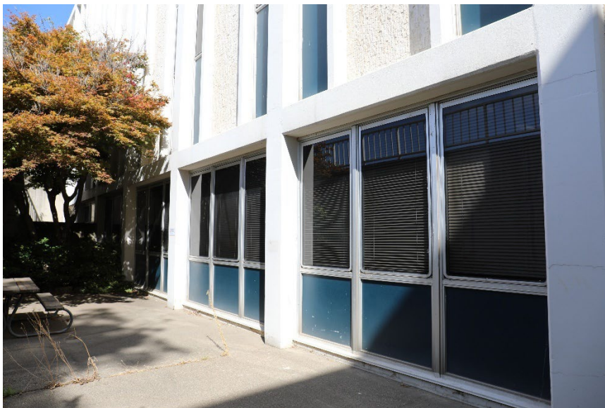
FIGURE 63 VIEW OF THE GROUND LEVEL FENESTRATION ALONG THE SOUTH ELEVATION OF THE COURTHOUSE ANNEX, LOOKING WEST-NORTHWEST. (MIG 2025)
