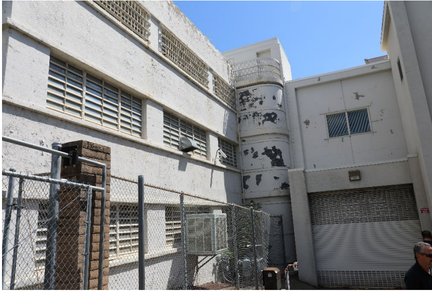
FIGURE 85 VIEW OF THE SOUTH ELEVATION AND THE ROUNDED CORNER OF THE STAIRWELL TOWER OF THE 1939 SHASTA COUNTY JAIL, LOOKING EAST. (MIG 2025)
