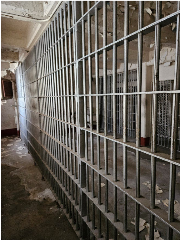
FIGURE 89 VIEW OF CELLBLOCK NO. 1. (MIG 2025)
