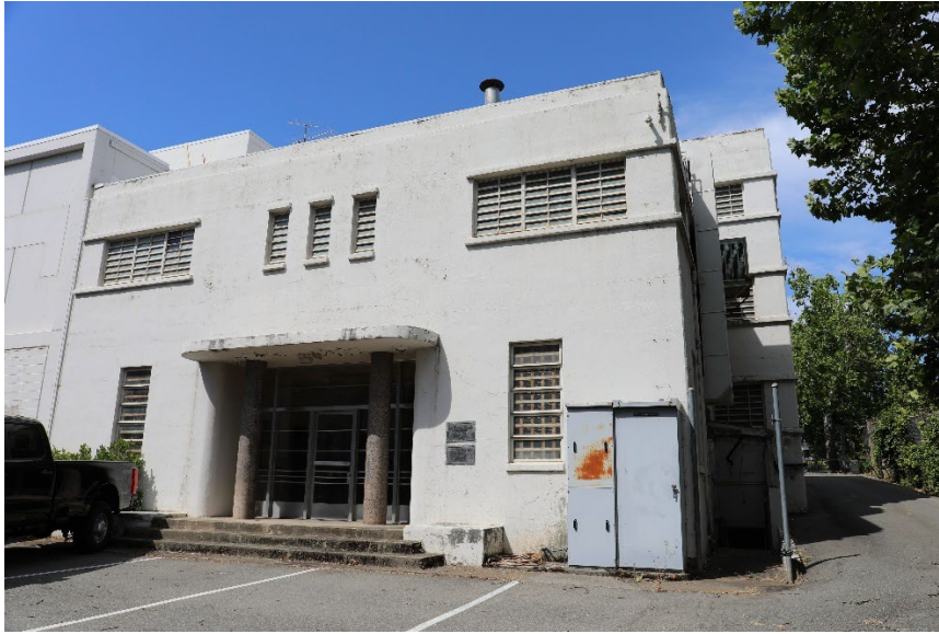
FIGURE 81 VIEW OF THE 1939 SHASTA COUNTY JAIL, LOOKING WEST-SOUTHWEST. (MIG 2025)
