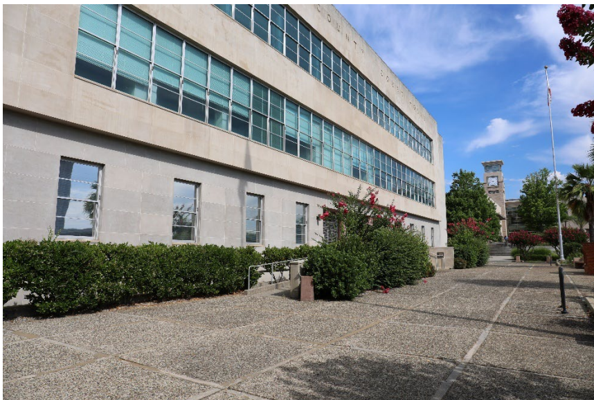
FIGURE 42 VIEW OF THE GROUND LEVEL WINDOWS AND THE AGGREGATE CONCRETE PLAZA IN THE FOREGROUND. LOOKING NORTHWEST. (MIG 2025)
