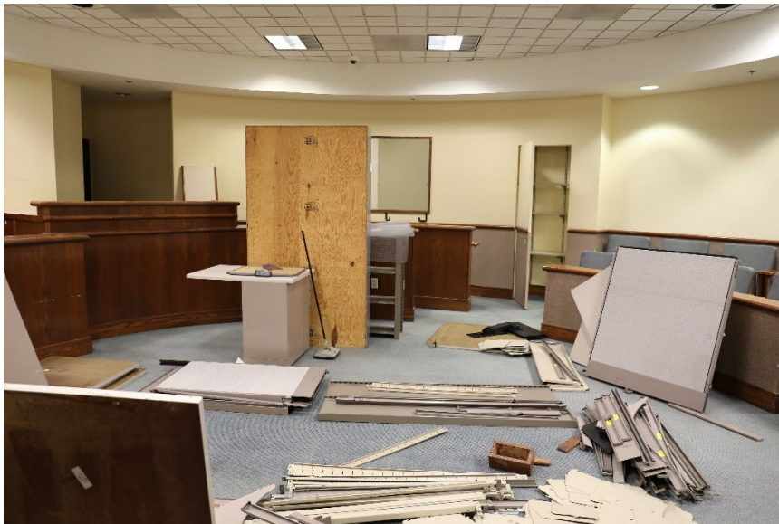
FIGURE 75 VIEW OF A FORMER COURTROOM IN THE COURTHOUSE ANNEX. NOTE THE REMNANTS OF THE SEMICIRCULAR LAYOUT. (MIG 2025)
