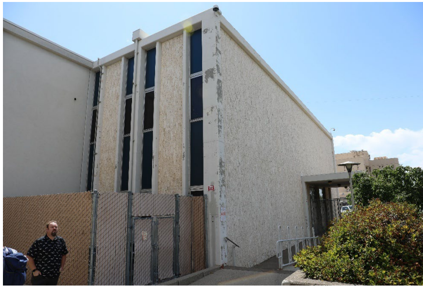
FIGURE 68 VIEW OF THE NORTH ELEVATION OF THE COURTHOUSE ANNEX, WEST OF THE SALLYPORT. LOOKING SOUTHEAST. (MIG 2025)
