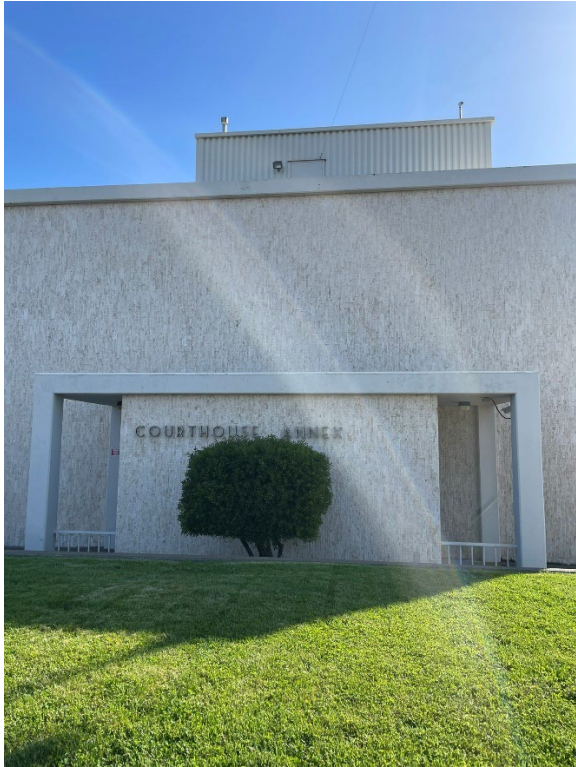
FIGURE 66 VIEW OF THE COVERED ENTRANCE ON THE WEST ELEVATION OF THE COURTHOUSE ANNEX, WITH THE LETTERING ON THE SCREEN WALL UNOBSCURED BY VEGETATION. LOOKING EAST. (MIG 2025)
