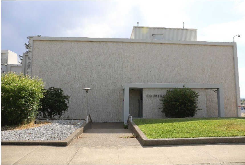
FIGURE 64 VIEW OF THE WEST ELEVATION OF THE COURTHOUSE ANNEX, LOOKING EAST. (MIG 2025)
