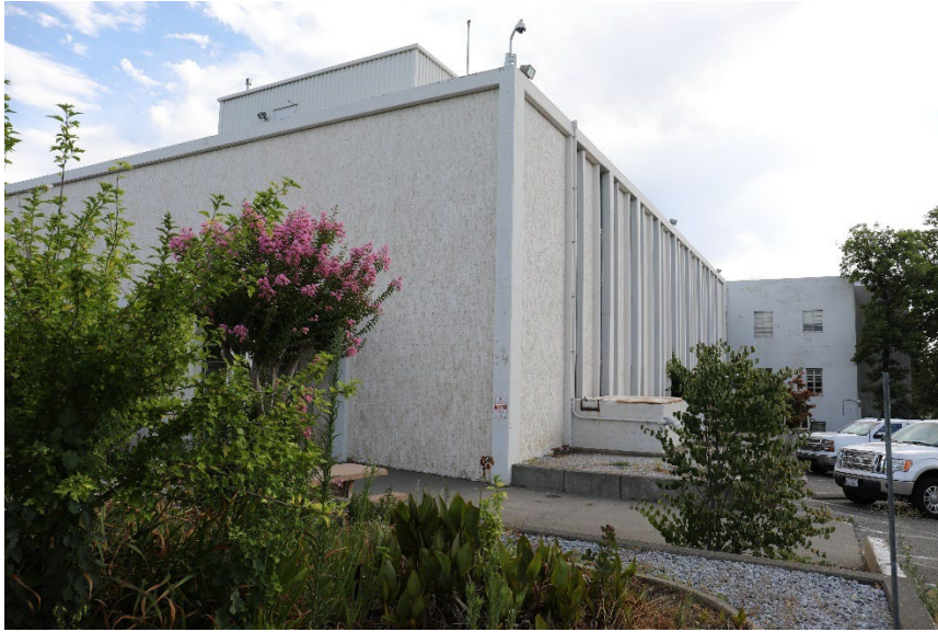
FIGURE 71 VIEW OF THE COURTHOUSE ANNEX WITH THE PLANTERS IN THE FOREGROUND, LOOKING EAST-NORTHEAST. (MIG 2025)
