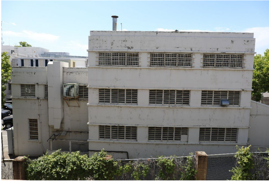
FIGURE 83 VIEW OF THE NORTH ELEVATION OF THE 1939 COUNTY JAIL FROM THE PARKING STRUCTURE ALONG BUTTE STREET, LOOKING SOUTH. (MIG 2025)
