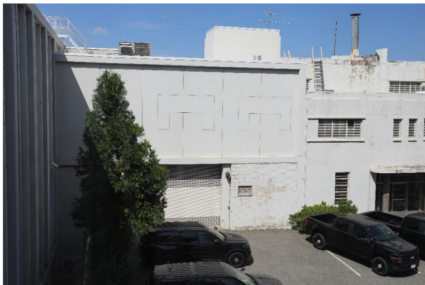
FIGURE 76 VIEW OF THE SALLYPORT STRUCTURE FROM THE MAIN COURTHOUSE, LOOKING WEST. (MIG 2025)
