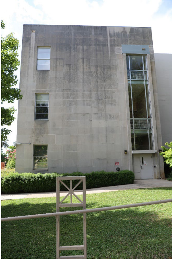
FIGURE 44 VIEW OF THE NORTH ELEVATION OF THE COVERED STAIRWELL, LOOKING SOUTH. (MIG 2025)
