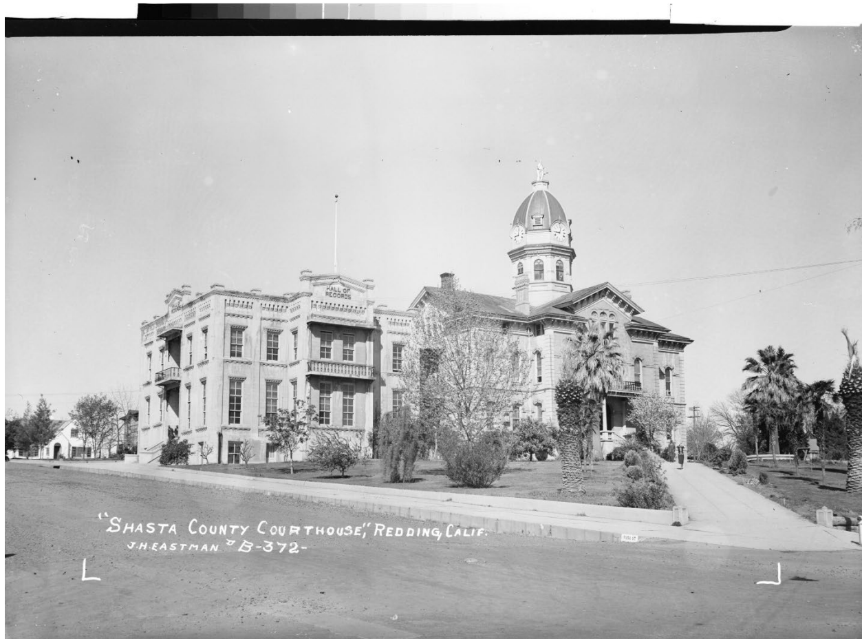
FIGURE 15 PHOTOGRAPH OF THE 1889 COURTHOUSE AND THE 1909 HALL OF JUSTICE BUILDINGS, 1937. PHOTOGRAPHED BY JERVIE HENRY EASTMAN. (B-372, EASTMAN'S ORIGINAL COLLECTION, U.C. DAVIS SPECIAL COLLECTIONS LIBRARY.)
