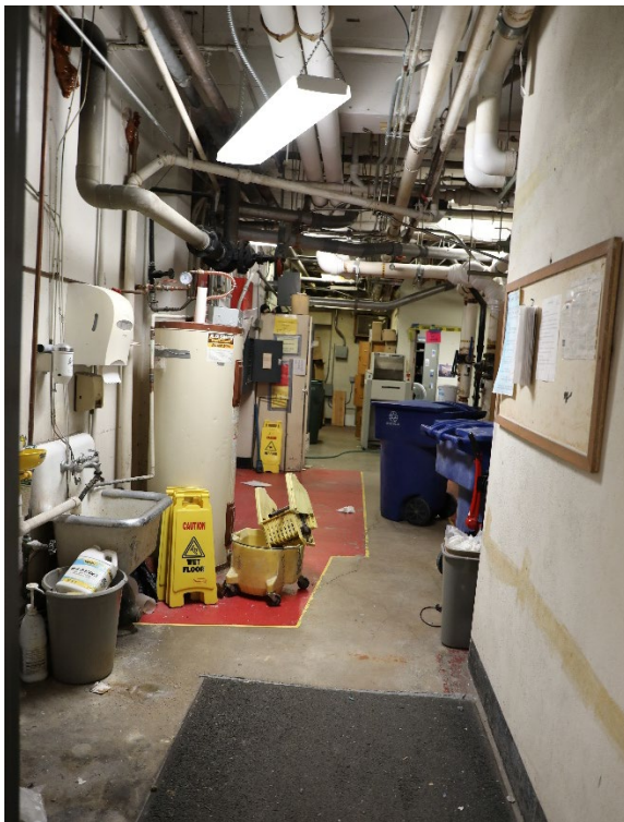
FIGURE 54 VIEW OF THE MECHANICAL ROOM. (MIG 2025)
