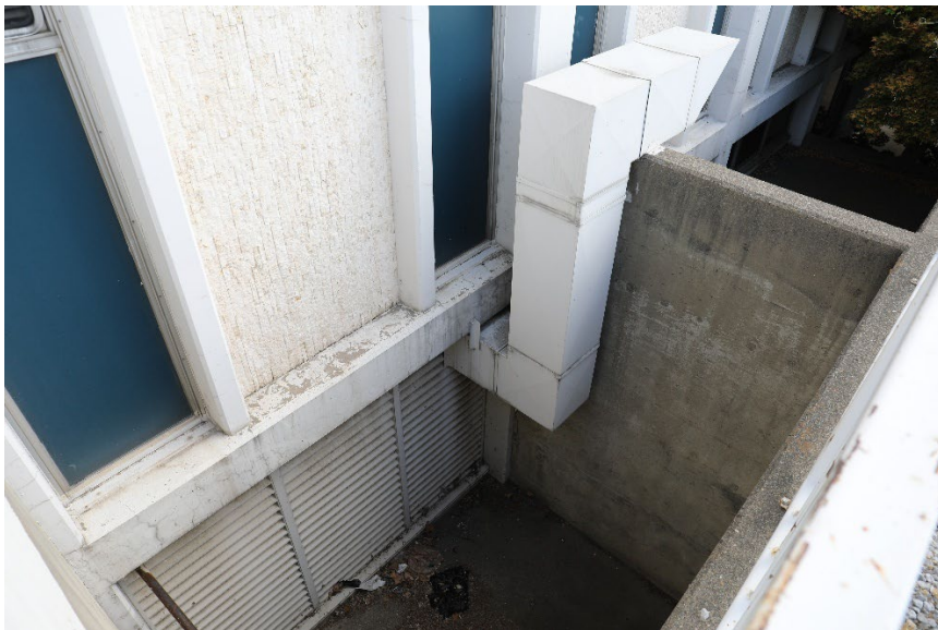
FIGURE 70 VIEW OF THE ENCLOSED SPACE THAT HOUSES THE VENTILATION AND MECHANICAL DUCTS ALONG THE SOUTH ELEVATION OF THE COURTHOUSE ANNEX. (MIG 2025)
