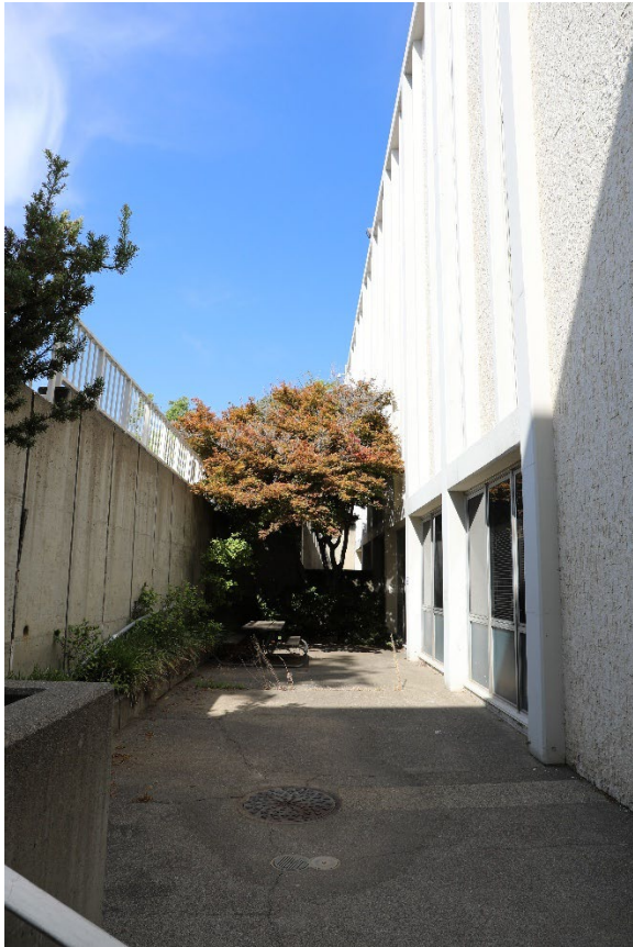
FIGURE 69 VIEW OF THE ENCLOSED PATIO ALONG THE SOUTH ELEVATION OF THE COURTHOUSE ANNEX, LOOKING WEST. (MIG 2025)
