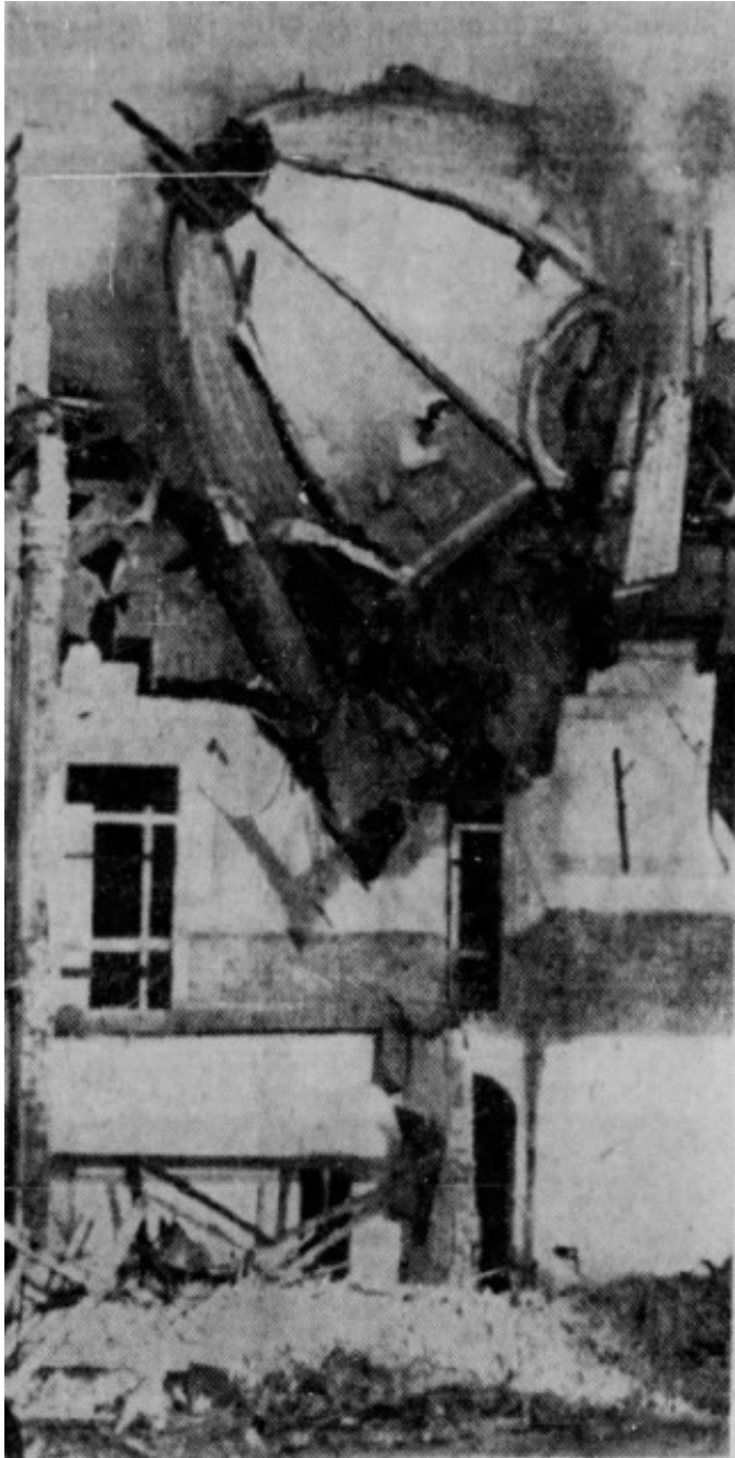
FIGURE 33 IMAGE OF THE CUPOLA GETTING PULLED DOWN IN THE DEMOLITION OF THE 1889 COURTHOUSE IN 1963. ("TOWER TUMBLES," THE SAN FRANCISCO EXAMINER , MARCH 6, 1963.)
