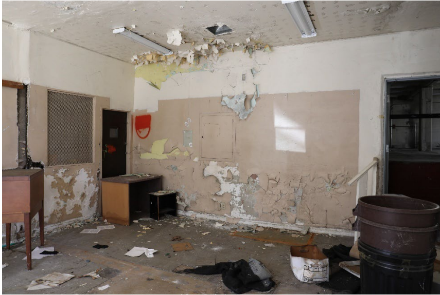
FIGURE 91 VIEW OF THE RECEPTION ROOM THROUGH THE MAIN ENTRANCE, LOOKING WEST-SOUTHWEST. NOTE THE FLOORING MATERIAL. (MIG 2025)
