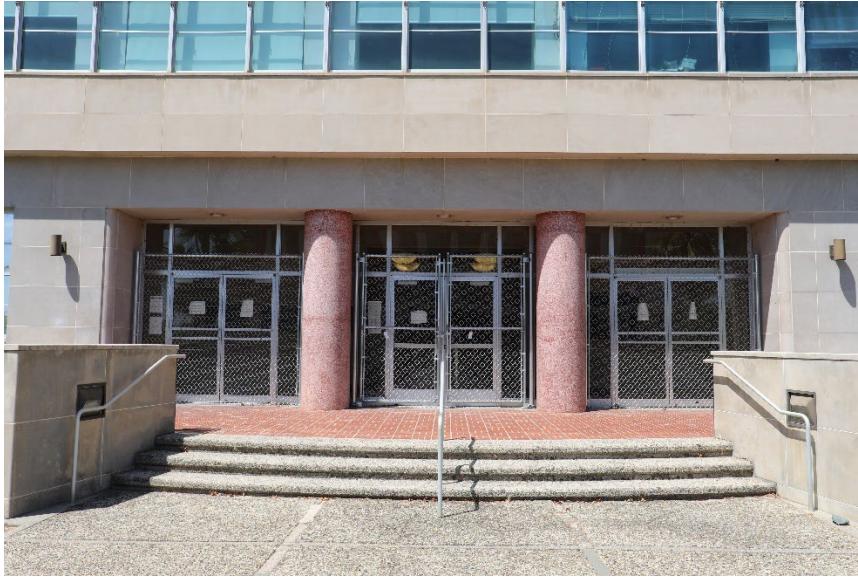
FIGURE 41 CLOSER VIEW OF THE MAIN ENTRANCE TO THE MAIN COURTHOUSE. LOOKING WEST. (MIG 2025)
