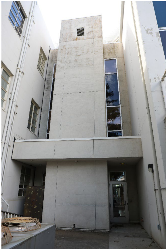
FIGURE 61 VIEW OF THE ELEVATOR SHAFT AND ENTRYWAY ON THE NORTH SIDE OF THE CONNECTING CORRIDOR, LOOKING SOUTH. (MIG 2025)
