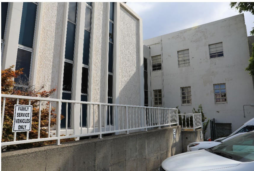
FIGURE 45 VIEW OF THE WEST ELEVATION OF THE MAIN COURTHOUSE, SOUTH OF THE CONNECTING CORRIDOR, LOOKING EAST-NORTHEAST. (MIG 2025)
