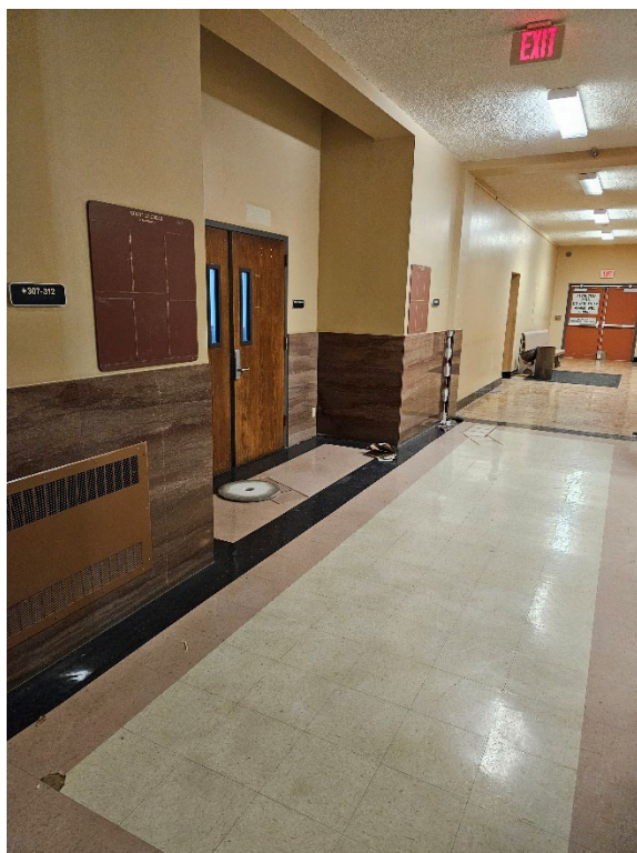
FIGURE 52 VIEW OF THE THIRD FLOOR CORRIDOR. NOTE THE RED MARBLE PANELING ON THE LOWER HALF OF THE WALL. (MIG 2025)
