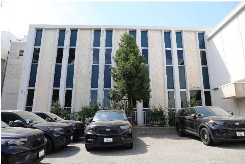
FIGURE 67 VIEW OF THE NORTH ELEVATION OF THE COURTHOUSE ANNEX, EAST OF THE SALLYPORT, LOOKING SOUTH. (MIG 2025)
