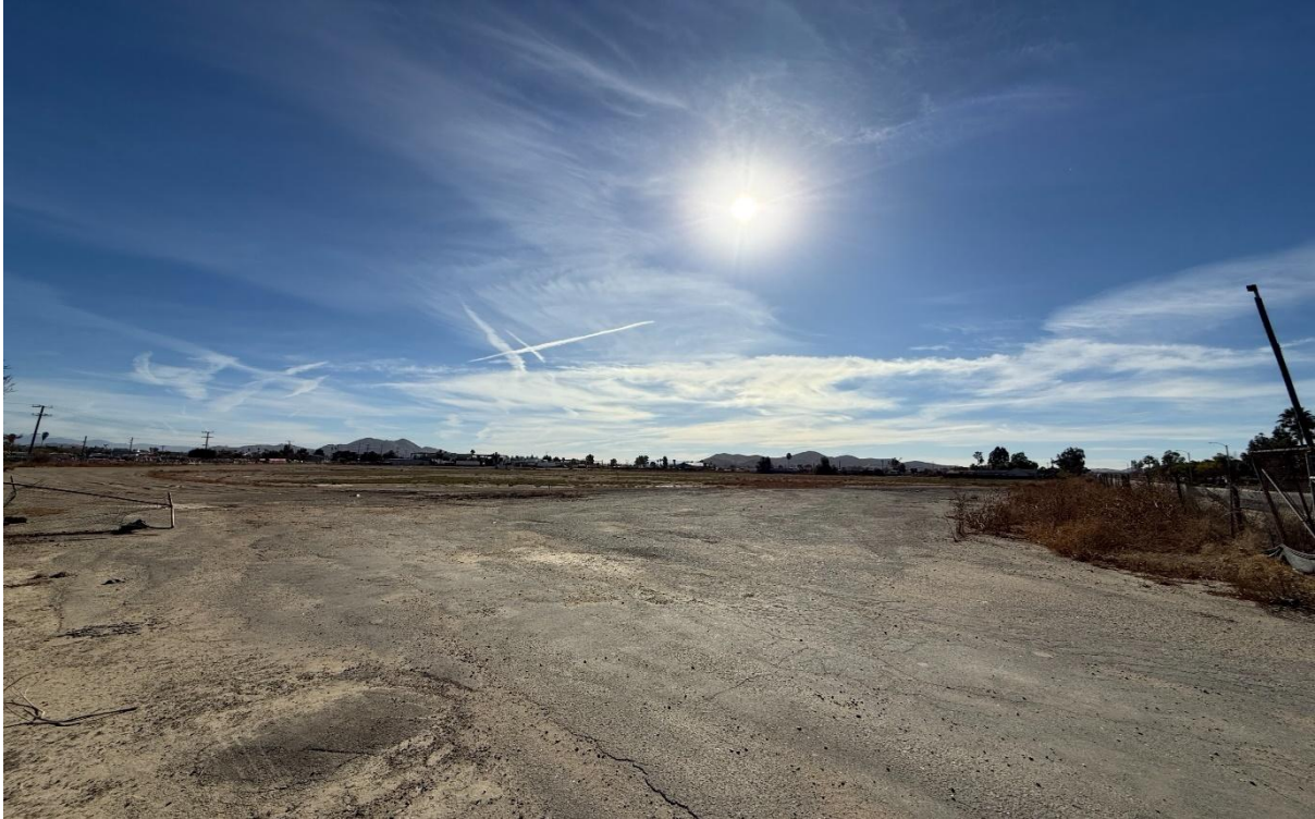
Photograph 1. View from northwest corner looking southeast within project site.
