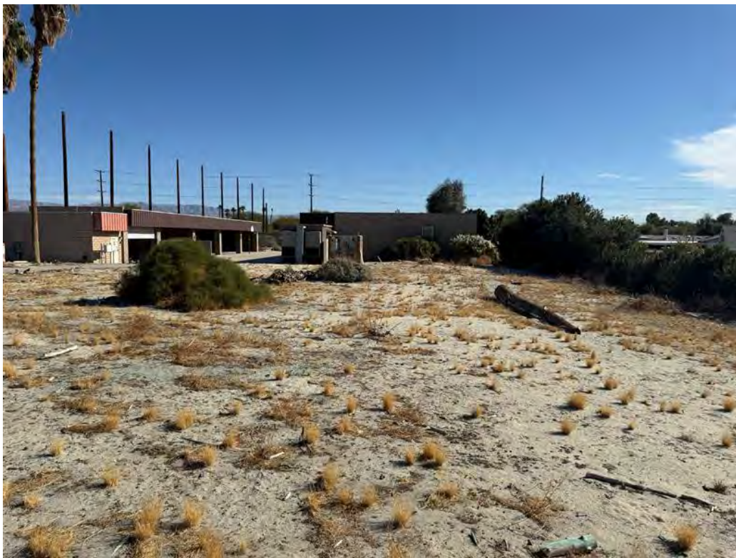
Photograph 4: East-facing view of the building in the southeast corner of the Project site.
