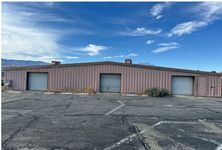
Photo 1: Maintenance facility's east-facing side; photo facing west.
