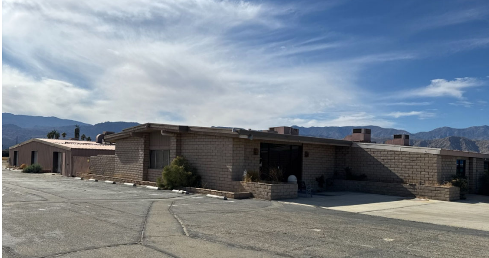
Photo 2: Clubhouse's northeast face; photo facing southwest.
