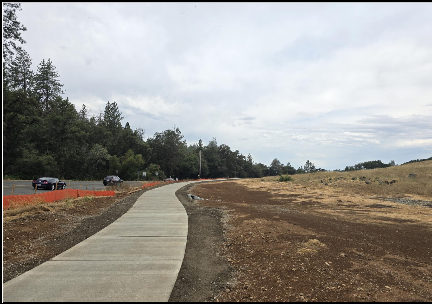
Figure 2: Project Site – Looking West
