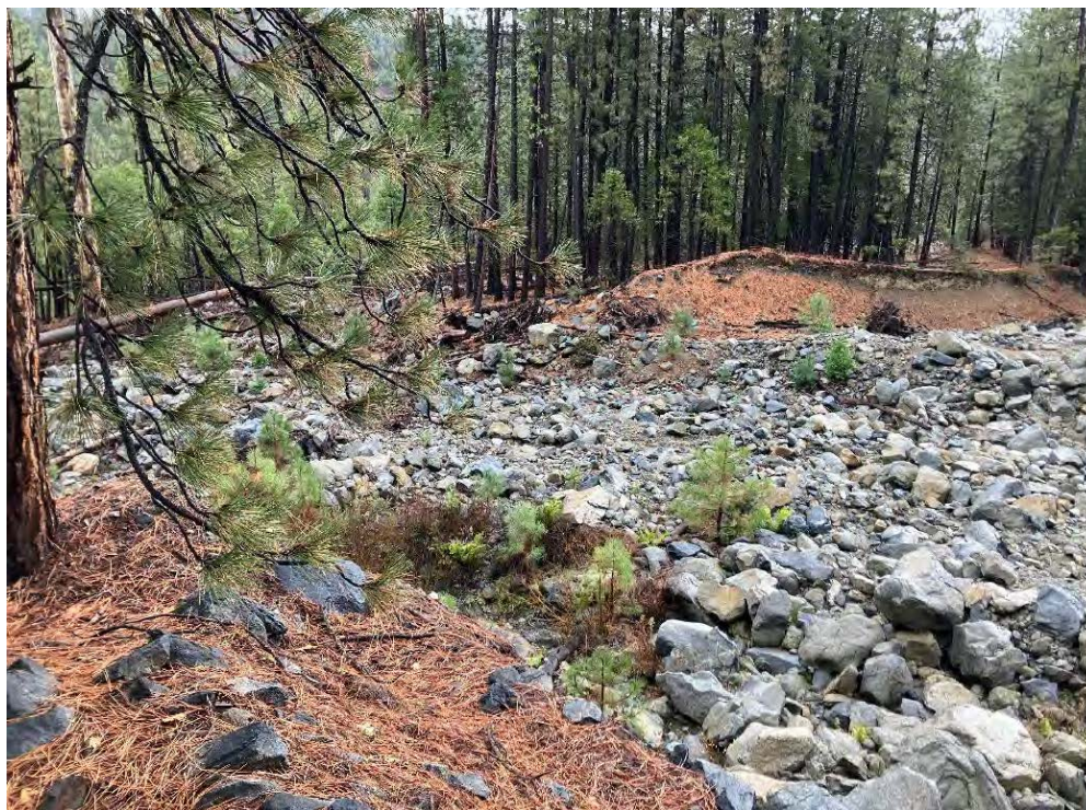
Figure 9 Project Work Area Looking Downstream (East Channel to the Left, Discharge Channel to the Right), Existing Conditions
