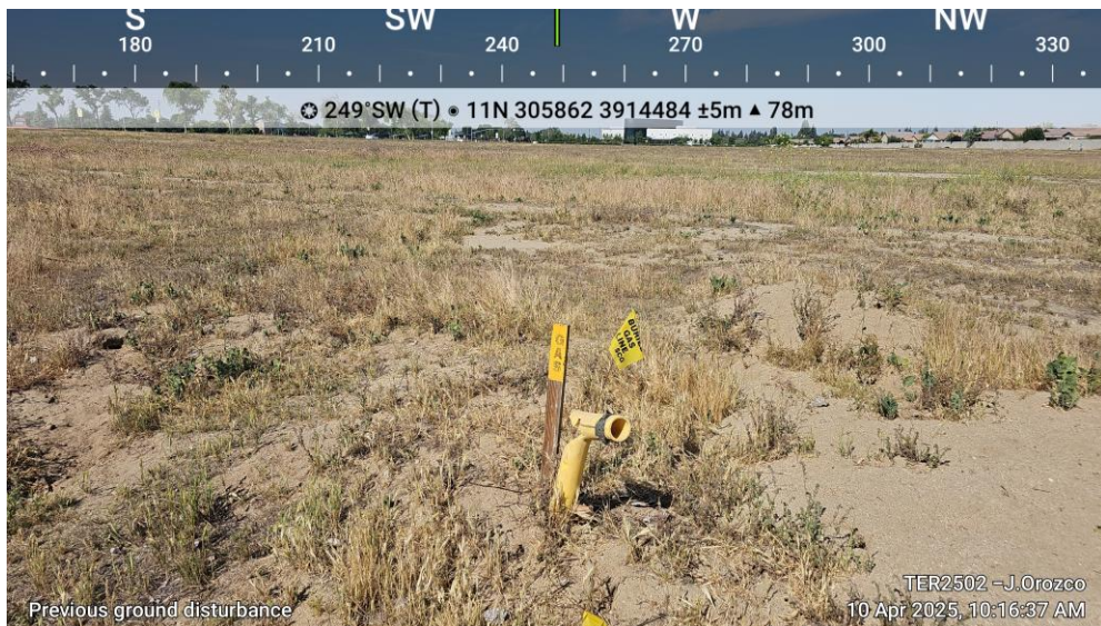
Photo 4: Modern Gas Pipeline in the former area of the Pioneer Canal (View SW)
