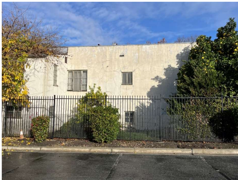
Figure 4. The south elevation of 944 San Leandro Avenue.
