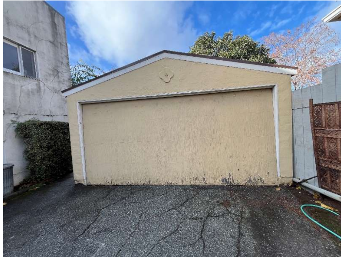
Figure 10. The east façade of the detached garage between 944 and 950 San Leandro Avenue elevation of 944 San Leandro Avenue.
