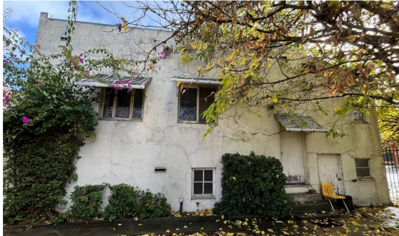
Figure 3. The west (rear) elevation of 944 San Leandro Avenue.
