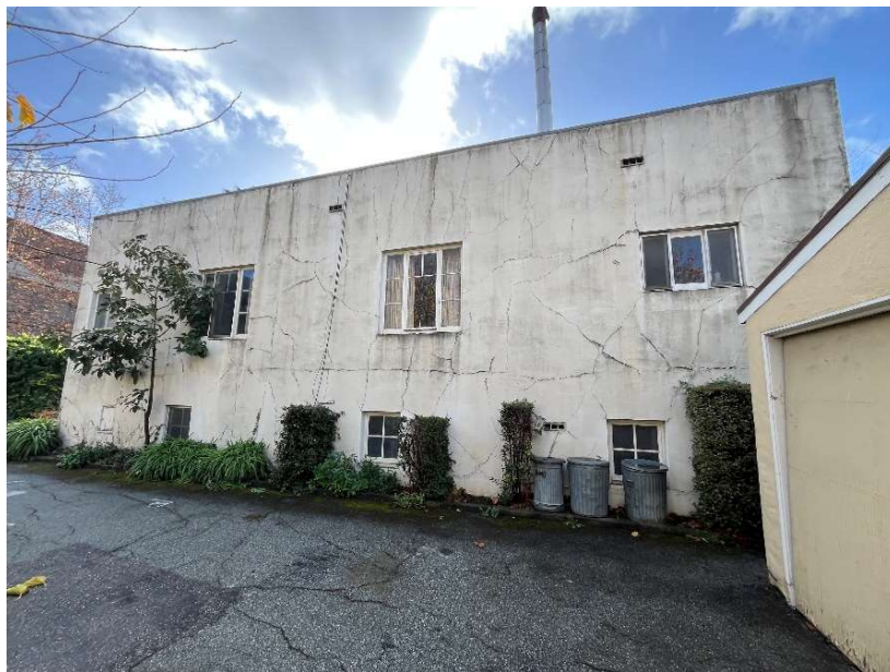
Figure 2. The north elevation of 944 San Leandro Avenue.
