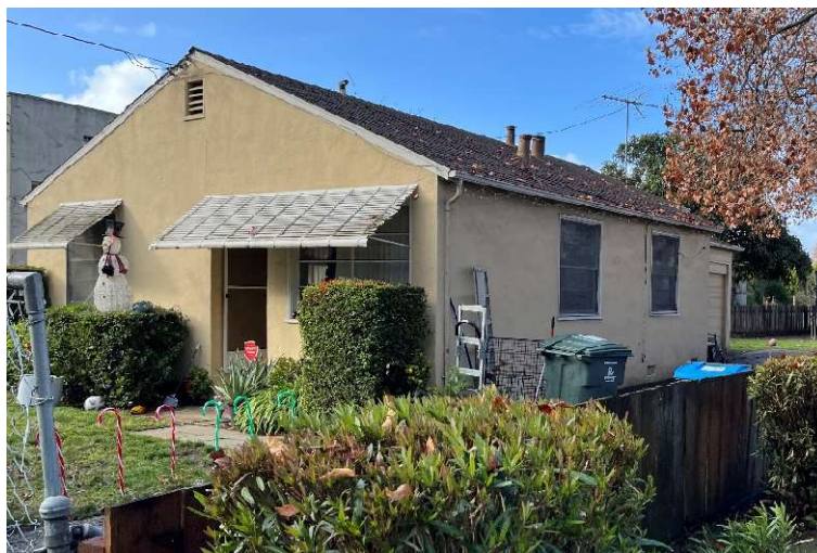
Figure 6. The east (main) and north elevations of the house at 950 San Leandro Avenue.
