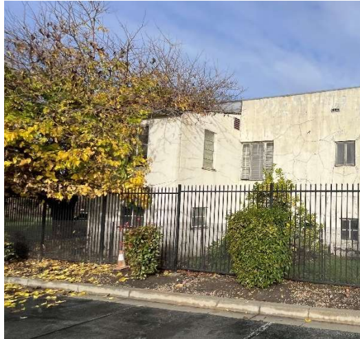
Figure 5. Detail of the two-story addition on the south elevation of 944 San Leandro.
