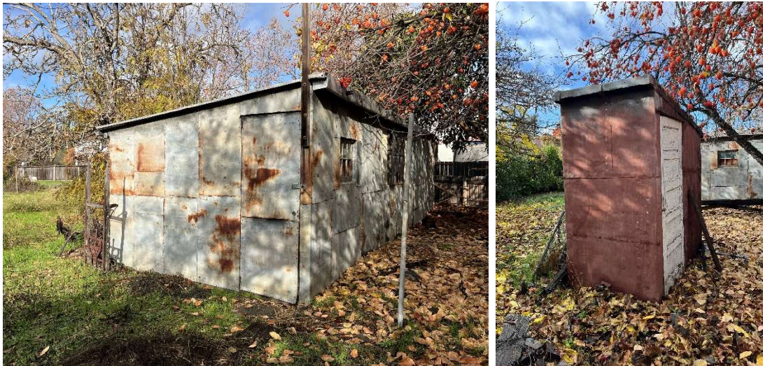
Figures 11 and 12. Two outbuildings behind 944 and 950 San Leandro Avenue.
