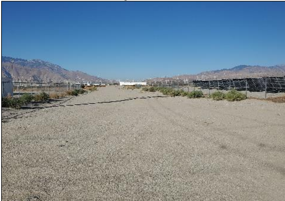
Overview of Project Site/19 th Avenue, with waste water reclamation facility at left, solar farm at right, view to the west.
