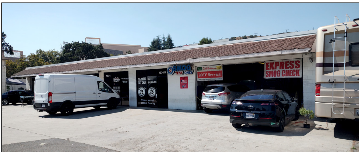
Figure 10. Auto service shop at 1934 E. Thousand Oaks Boulevard, circa 1960. (Photograph taken on August 5, 2025; view to the south)
