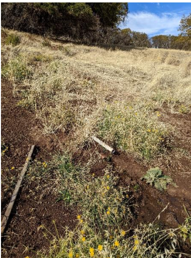
Spring 2 – PVC Visible. Flow measured at 0.01 gpm. Nov 11, 2022
