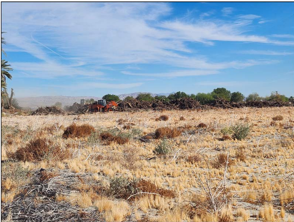
Figure 4. Overview of eastern side of APN 780010014 showing vegetation removal; view to the east.
