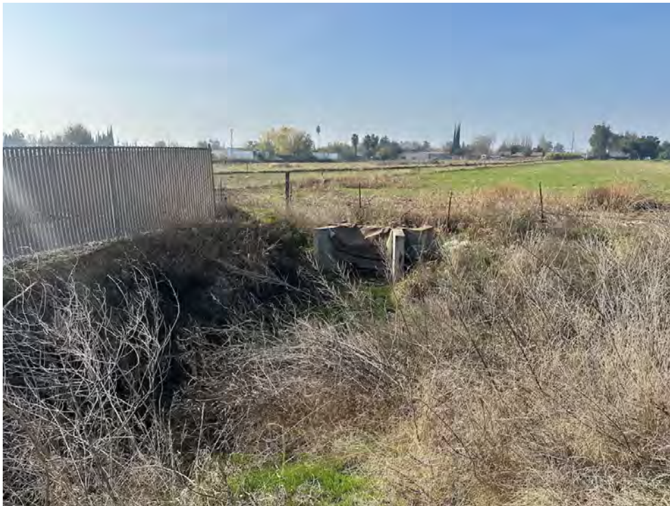
8. Facing west, the photo shows the culvert, located outside of the Survey Area, where water from feature ED 1b flows underground into the stormwater drainage system.
