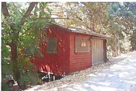
Garage structure (c. 1920s)
