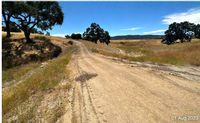
Photo 3: View southwest from existing culverted road crossing installed in February 2022 over unnamed blueline drainage.
