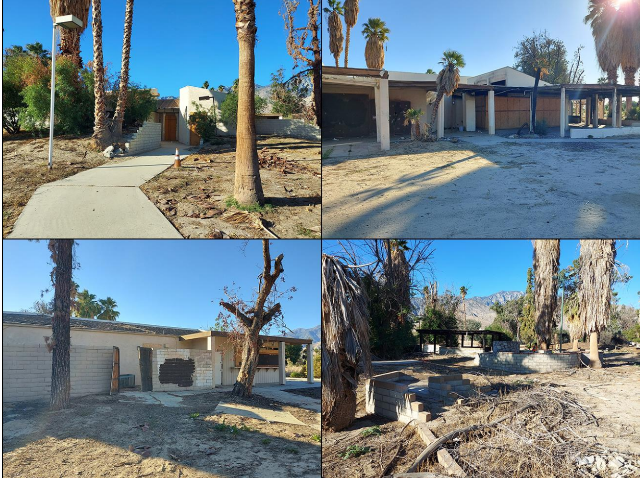
Bel Air Greens clubhouse. Clockwise from top left: northern side, view to the south; southern side, view to the north; front entry area, view to the southwest; western side, view to the east. (Taken on November 9, 2023)
