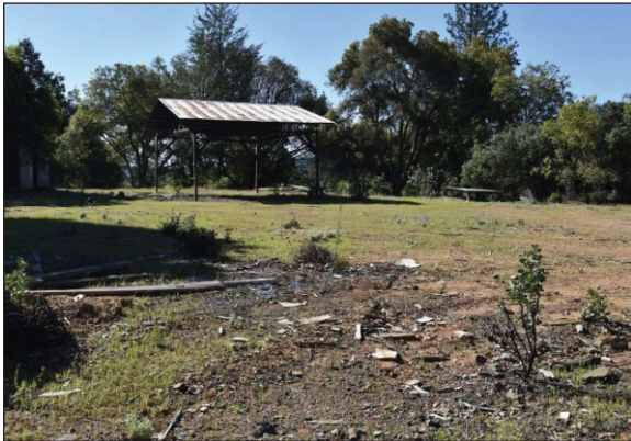
Photograph 2: View of the existing open-walled shed and trailer along the site's northeastern boundary. The shed will be demolished and the trailer will be removed by the City.
