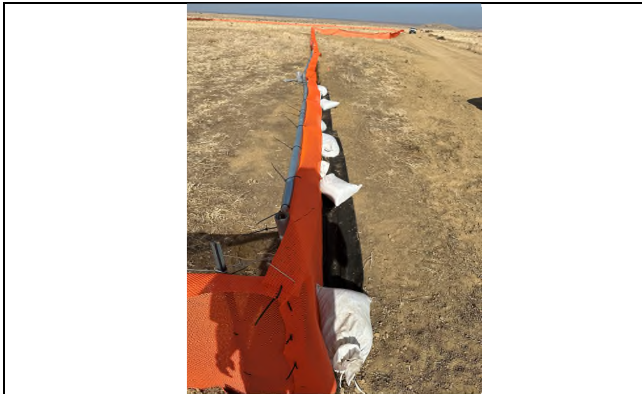
Photo 4. Exclusion fence installed around approximately 2.1 acres of grassland habitat within the Well Site.
