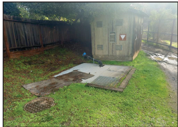
View of the sewage pump house adjacent to Redwood Road and the pond, that is planned for removal.
