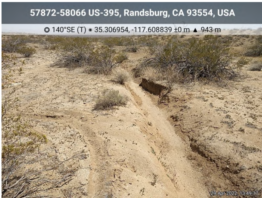
Image 2: View of channel in dry wash on western survey area.
