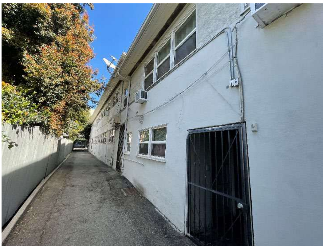
Figure 7-9. Western façade, facing northwest.
