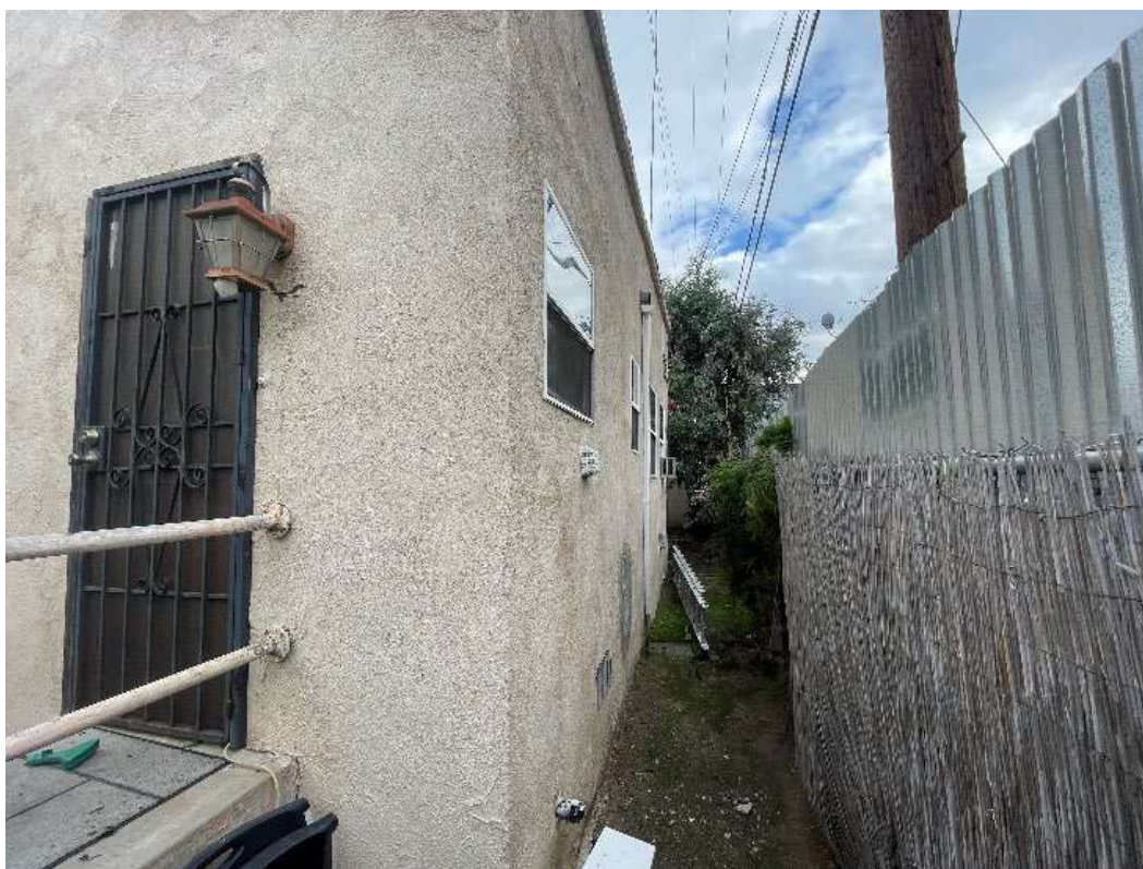
Figure 7-38. Southern façade, facing east.
