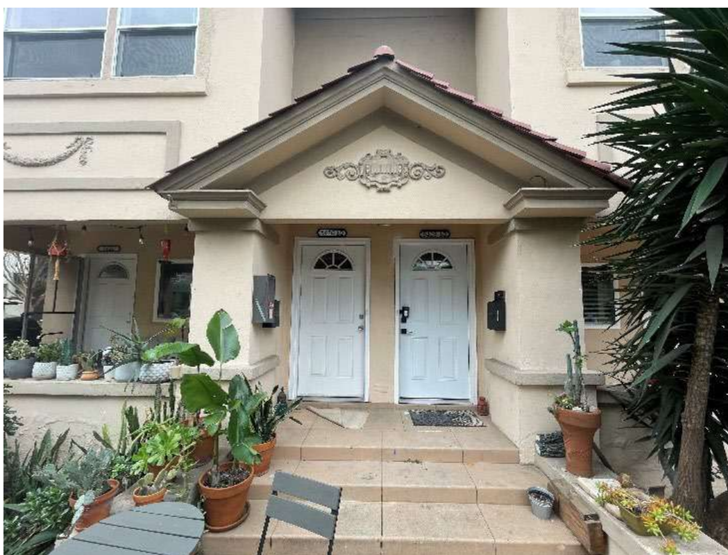
Figure 7-29. Primary façade, facing south.
