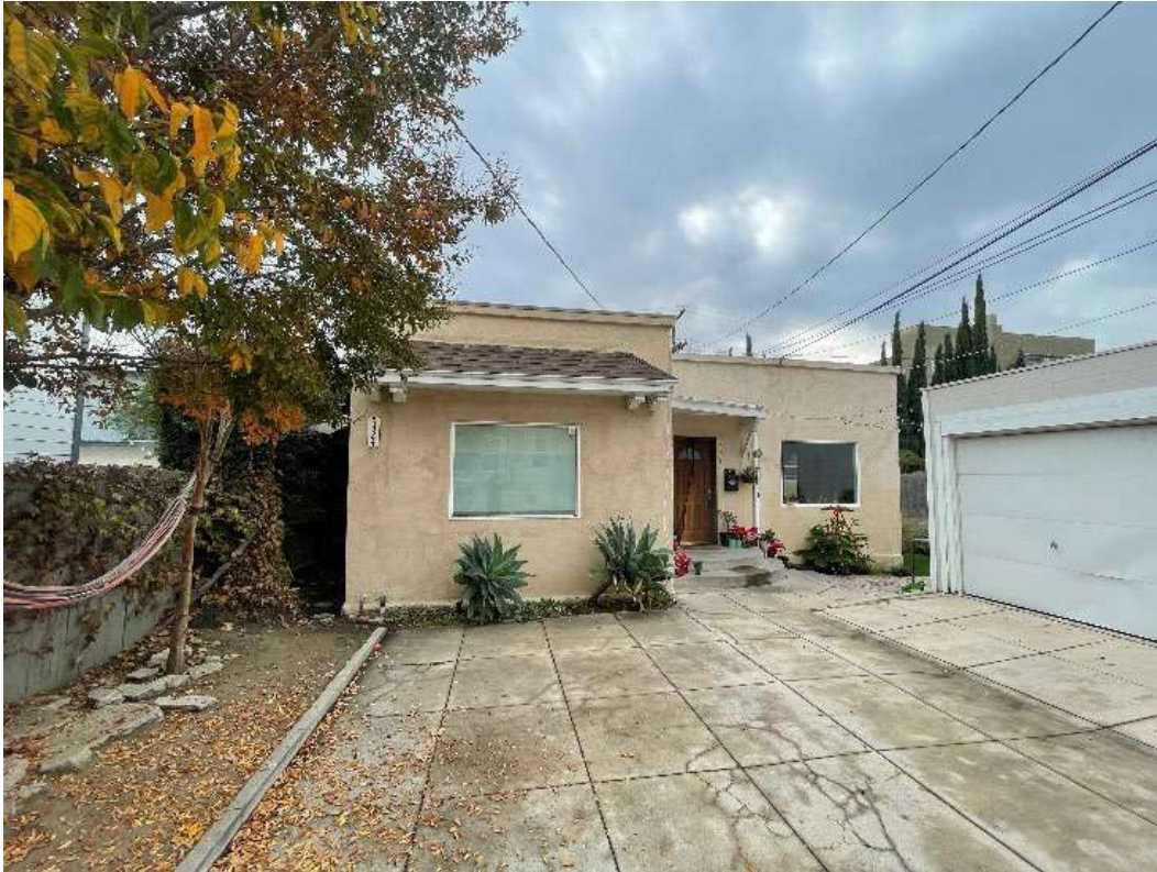
Figure 7-37. Primary façade, facing south.
