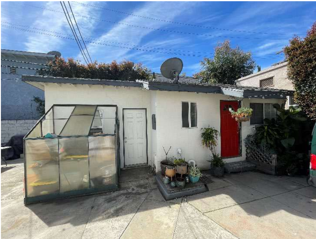
Figure 7-25. ADU, facing south.
