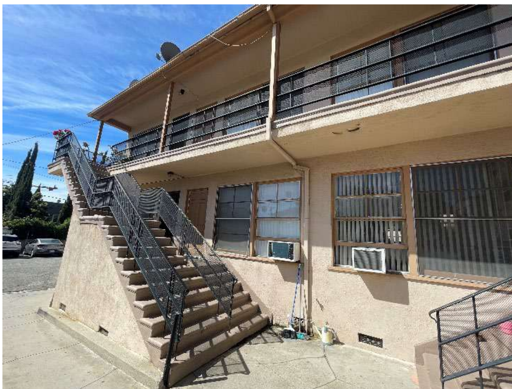
Figure 7-53. Eastern façade, facing southwest.
