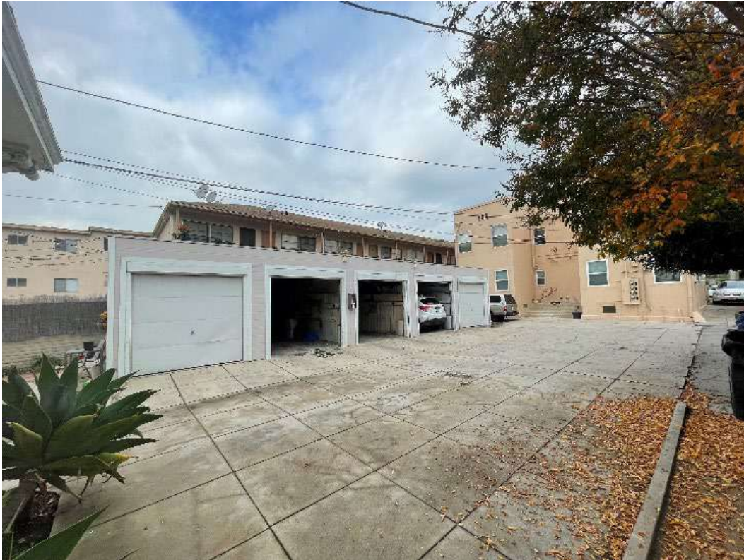
Figure 7-43. Auto garage, facing northwest.
