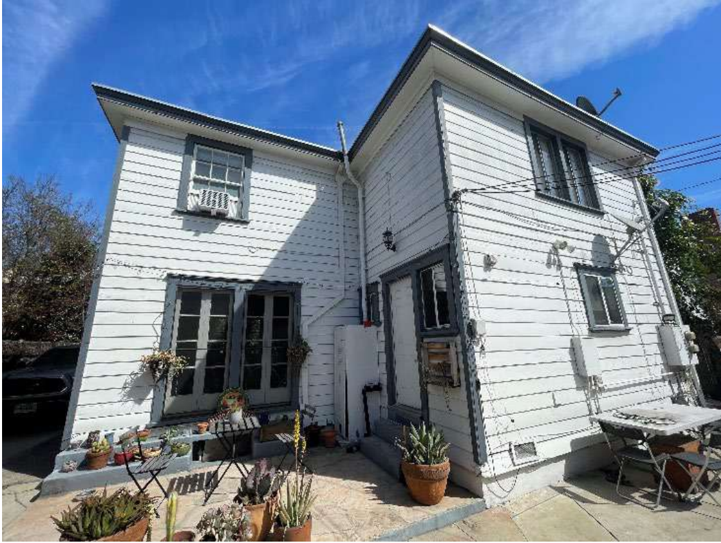
Figure 7-19. Southern façade, facing north.
