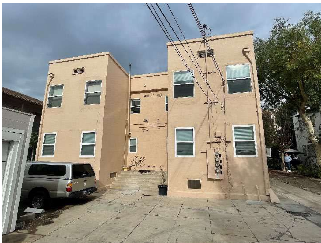
Figure 7-31. Southern façade, facing northwest.
