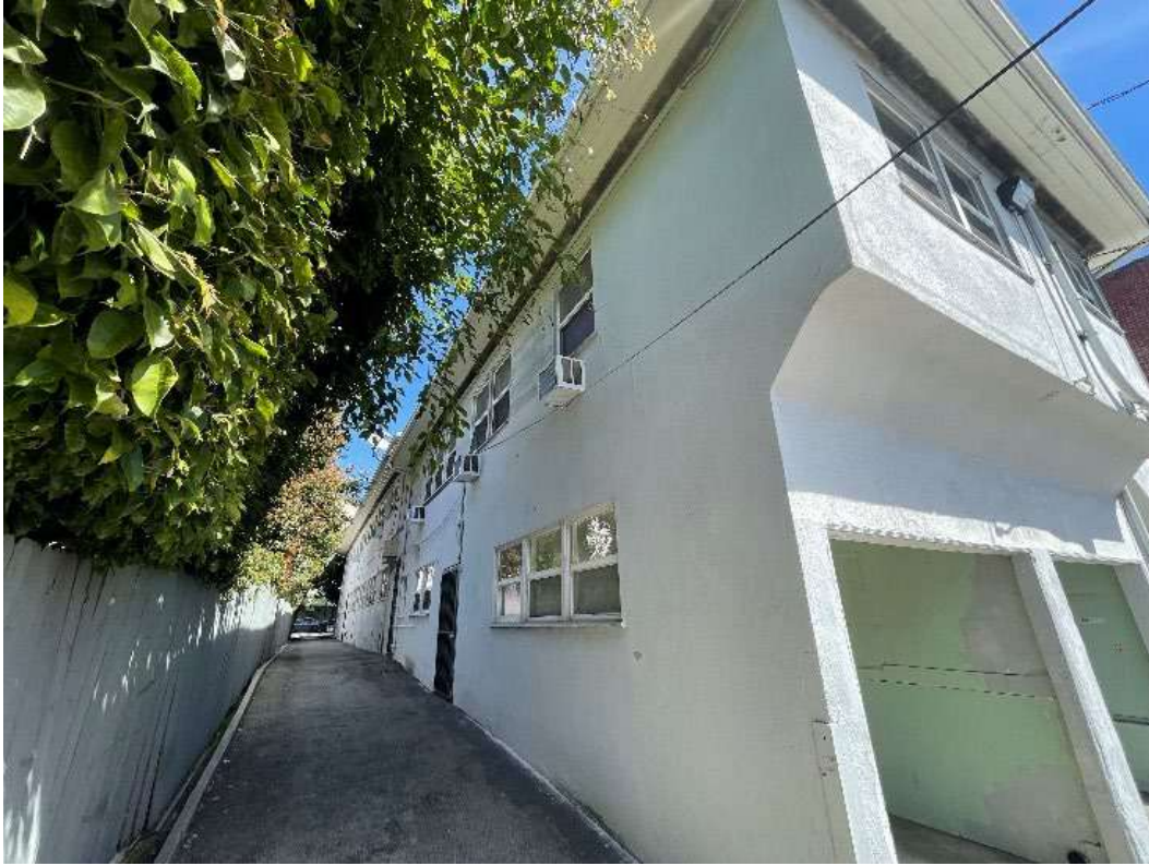
Figure 7-10. Western façade, facing northwest.
