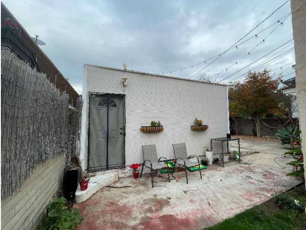
Figure 7-44. Auto garage side entry door, facing north.
