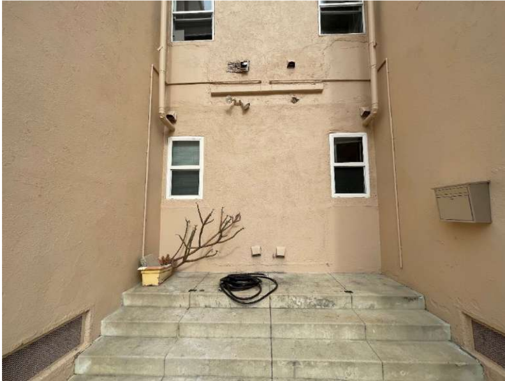
Figure 7-47. Door infill, facing north.
