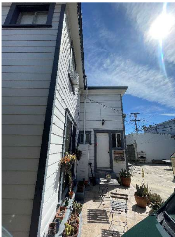
Figure 7-24. Western façade, facing east.
