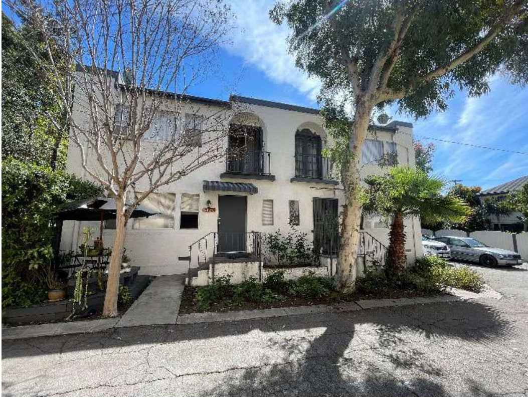
Figure 7-13. Primary façade, facing east.
