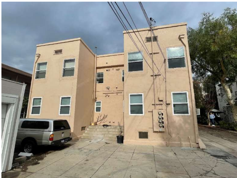
Figure 7-46. Rear porch area and door infill, facing northwest.
