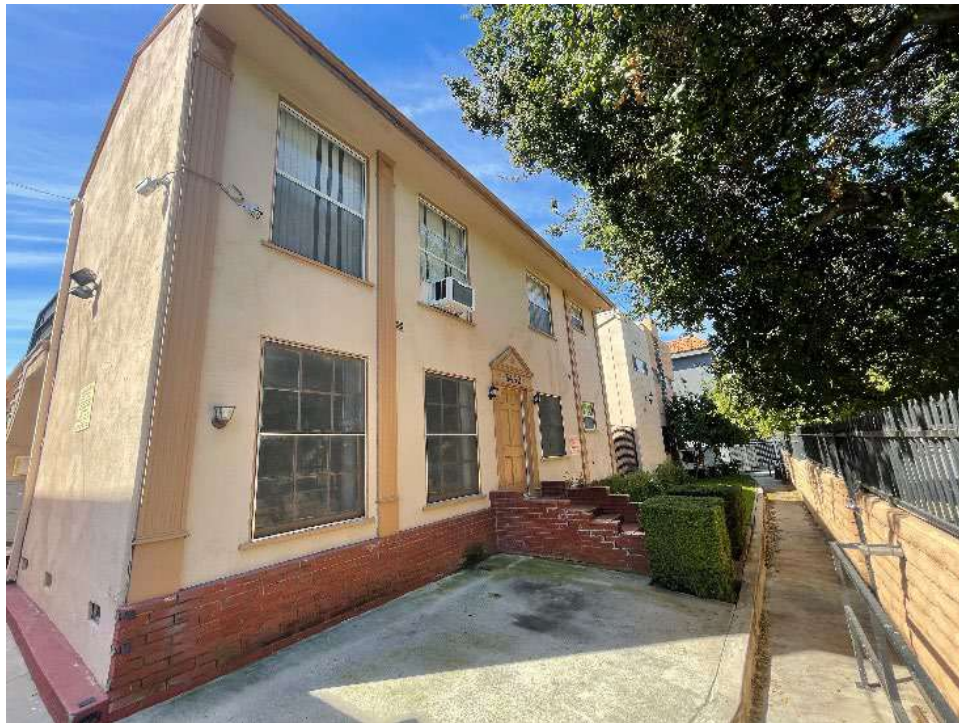
Figure 7-49. Primary façade, facing southwest.
