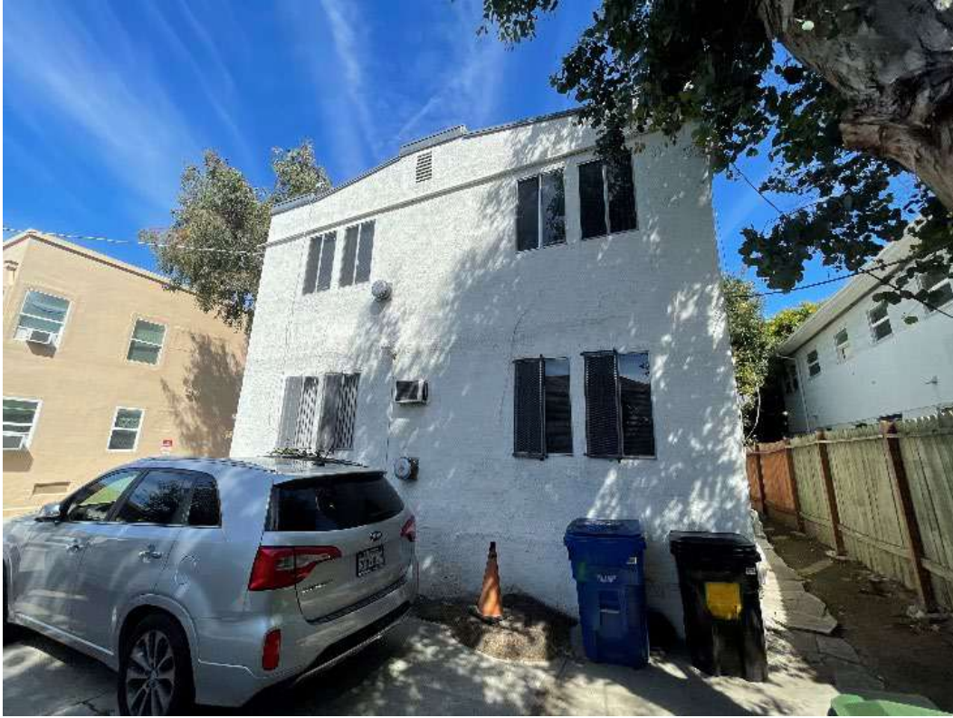
Figure 7-17. Southern façade, facing north.
