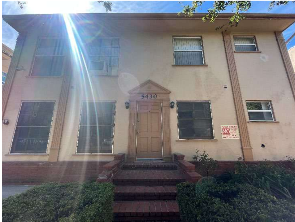
Figure 7-48. Primary façade, facing south.
