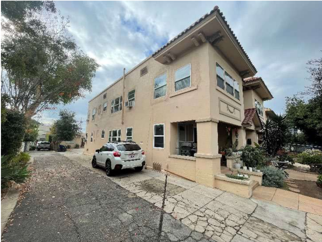
Figure 7-33. Eastern façade, facing southwest.
