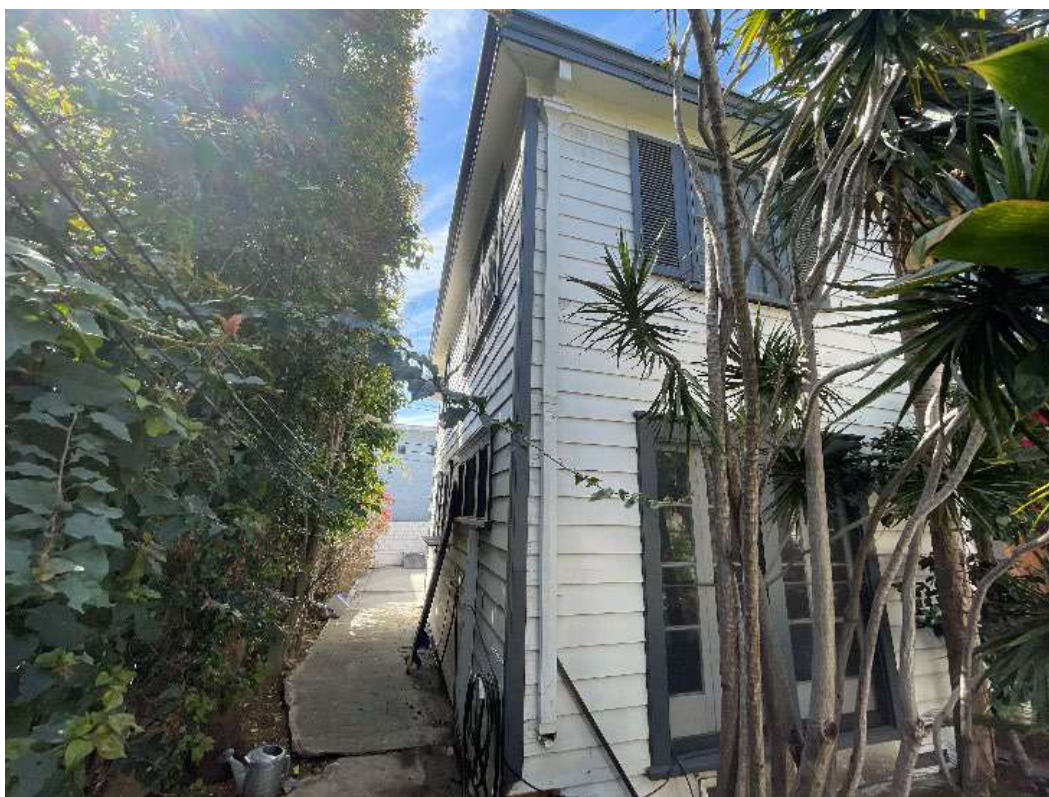
Figure 7-20. Eastern façade, facing southwest.
