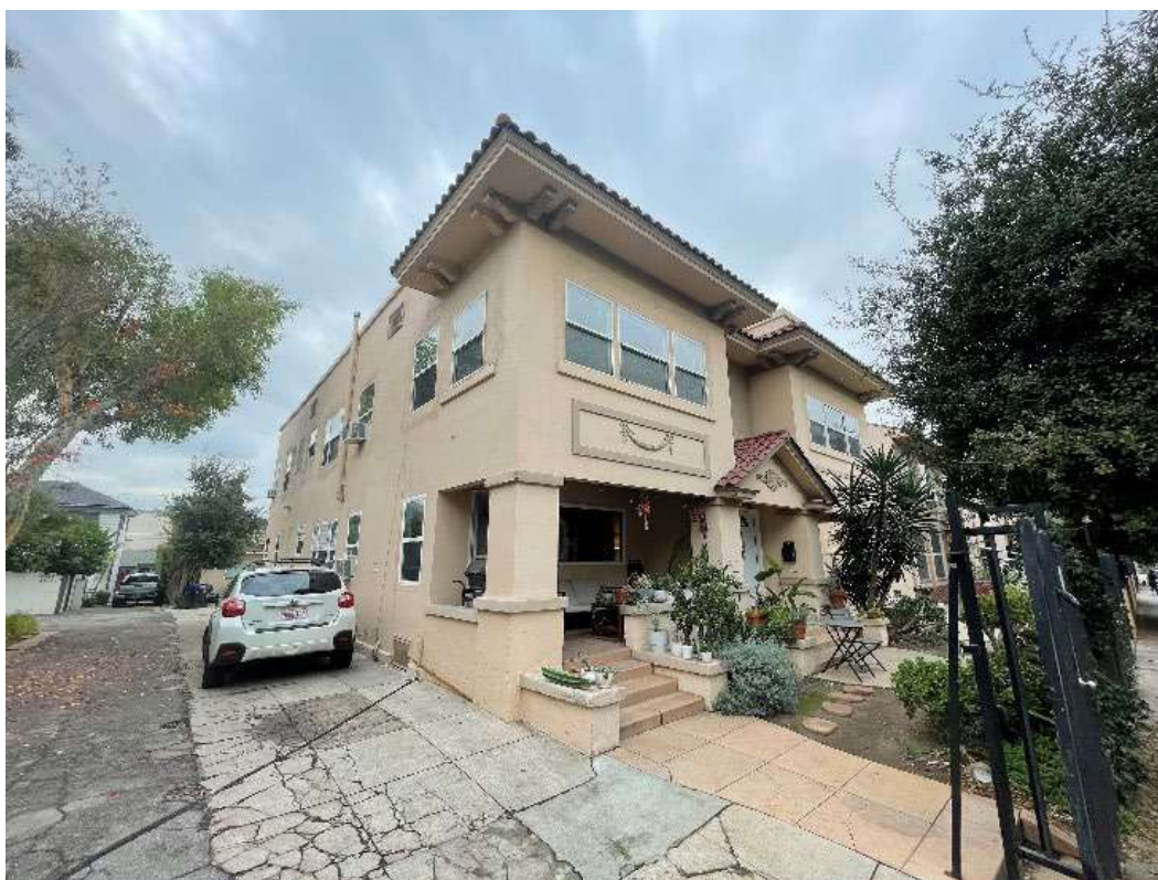
Figure 7-28. Primary façade, facing southwest.
