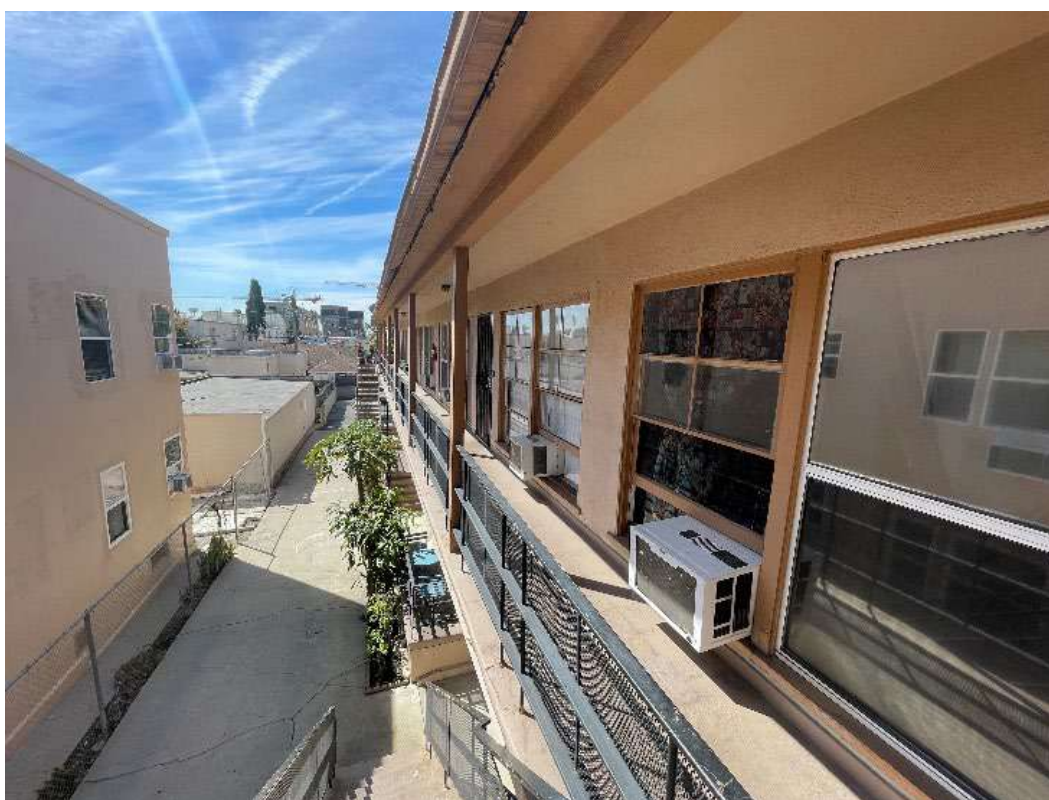
Figure 7-54. Eastern façade second floor, facing southwest.
