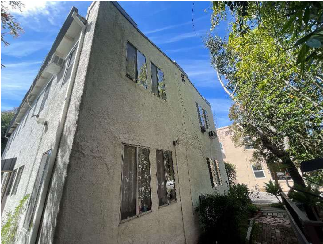
Figure 7-16. Northern façade, facing southwest.
