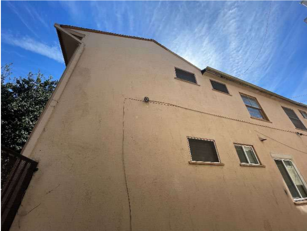
Figure 7-55. Western façade, facing east.
