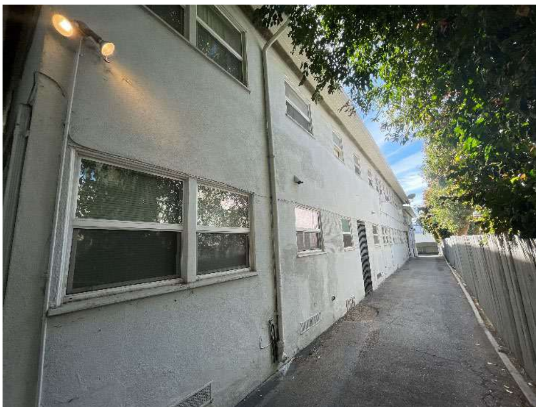
Figure 7-8. Western façade, facing south.
