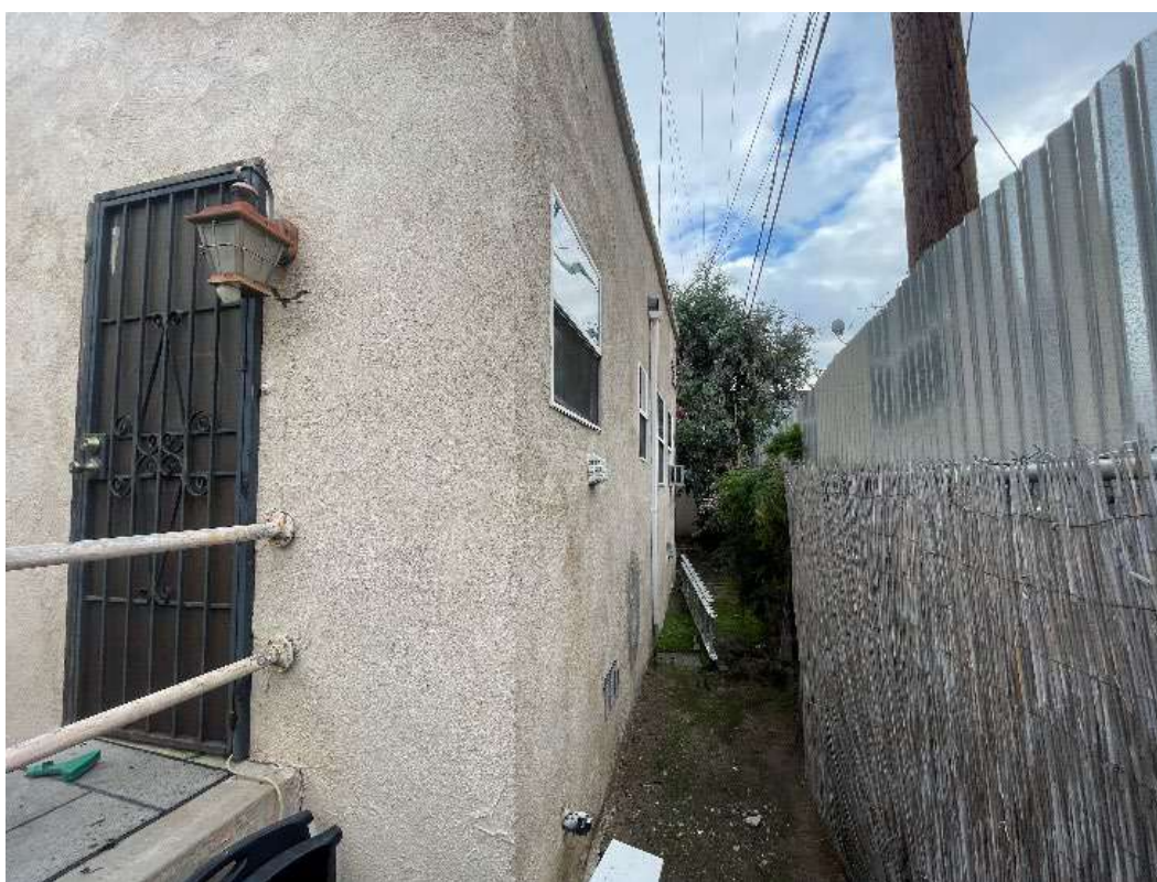
Figure 7-42. Western façade security door, facing northeast.
