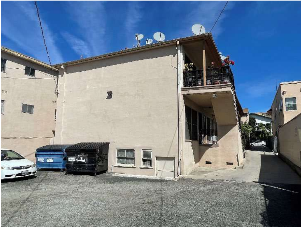
Figure 7-50. Southern façade, facing north.
