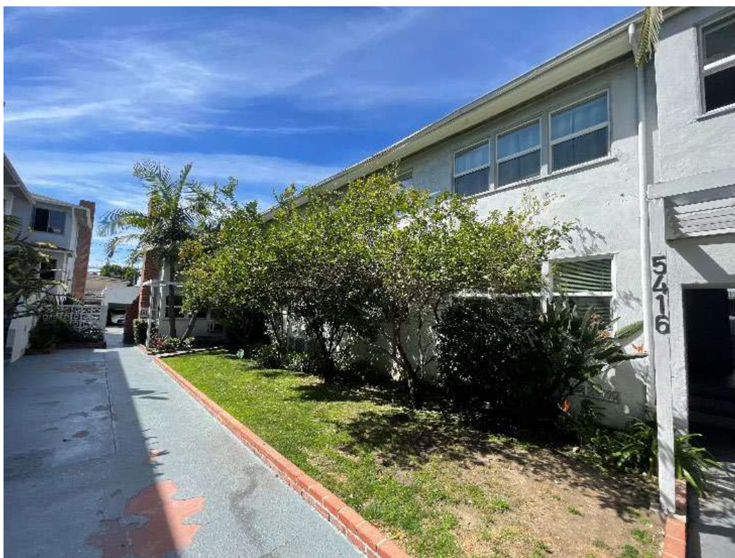
Figure 7-5. Eastern façade, facing southwest.
