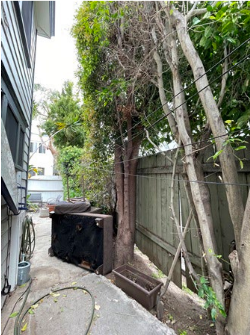
#11 Brush cherry – note narrow planter and lifted paving.
