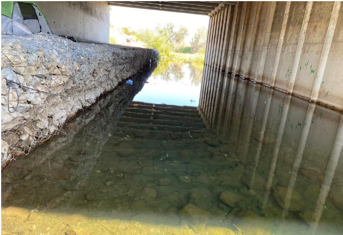
Figure 3-4 Blossom Hill Road Project Site Photo 2: Rock Gabion and Pool Habitat Under Bridge
