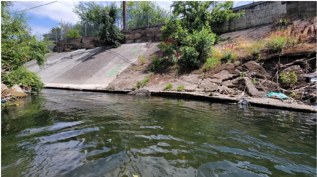
Figure 3-2 Malone Road Project Site Photo 2: Failed Concrete Lined Bank
