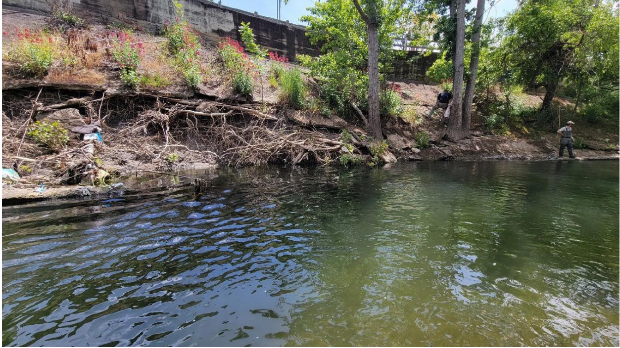
Figure 3-2 Malone Road Project Site Photo 2: Failed Concrete Lined Bank
