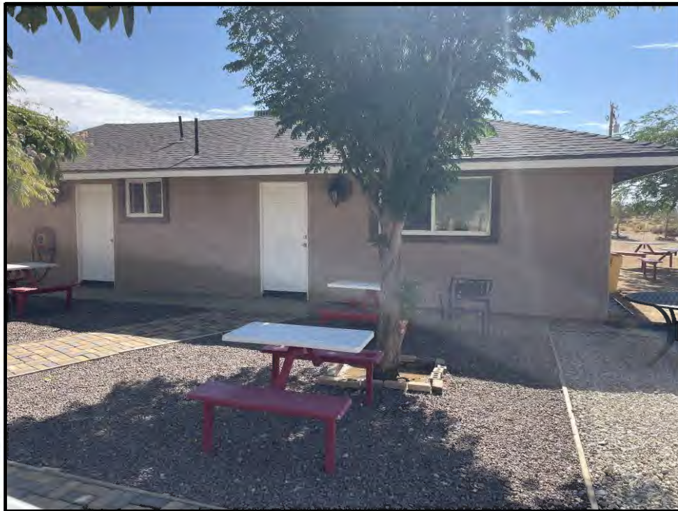
Plate 3.2–7: Overview of the west façade of the laundry building, facing east.
