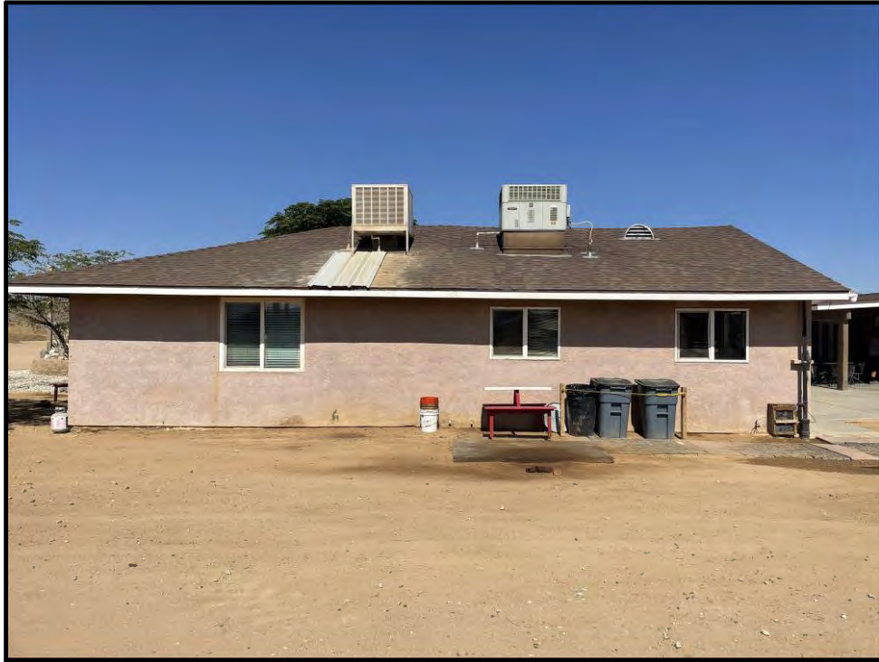
Plate 3.2–8: Overview of the east façade of the laundry building, facing west.
