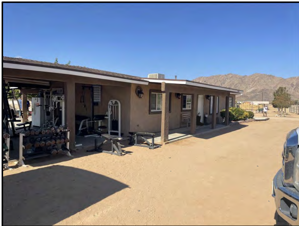
Plate 3.2–5: Overview of the north façade of the administration building, facing southwest.
