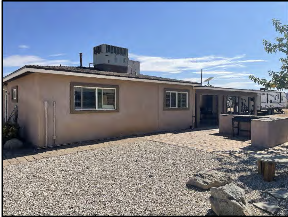
Plate 3.2–6: Overview of the south façade of the administration building, facing northwest.
