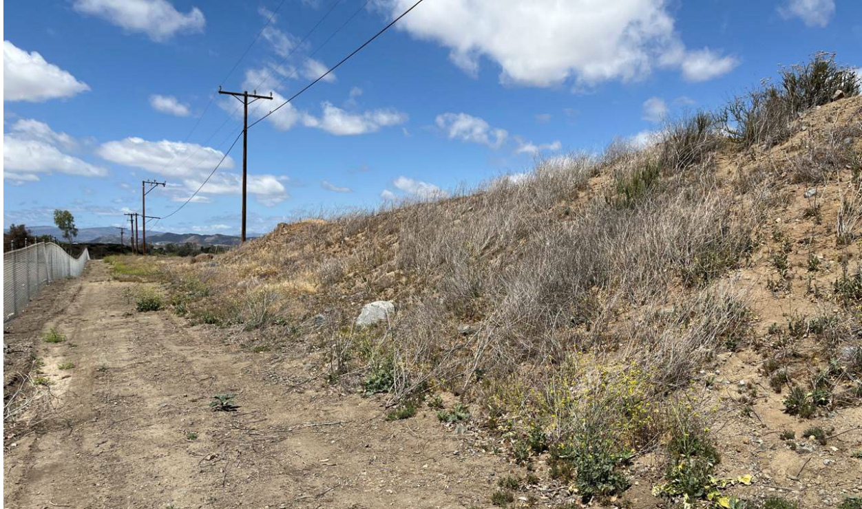
Figure 8. View of an ~10 foot tall berm of artificial fill in the southeastern portion of the site. Photo was taken facing west.
