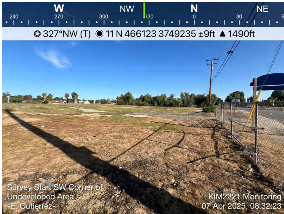
Photo 6: Overview of Project Site near SE Corner (View Northwest).
