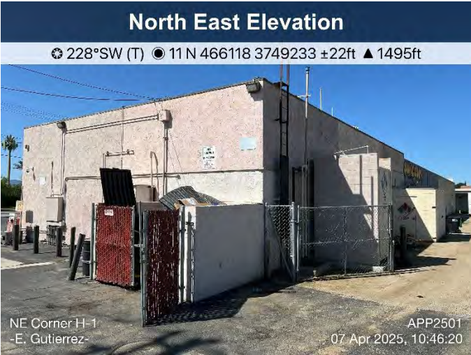
Photo 2: 16970 Van Buren Blvd. Overview (View SW)
