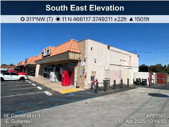
Photo 1: 16970 Van Buren Blvd. Overview (View NW)
